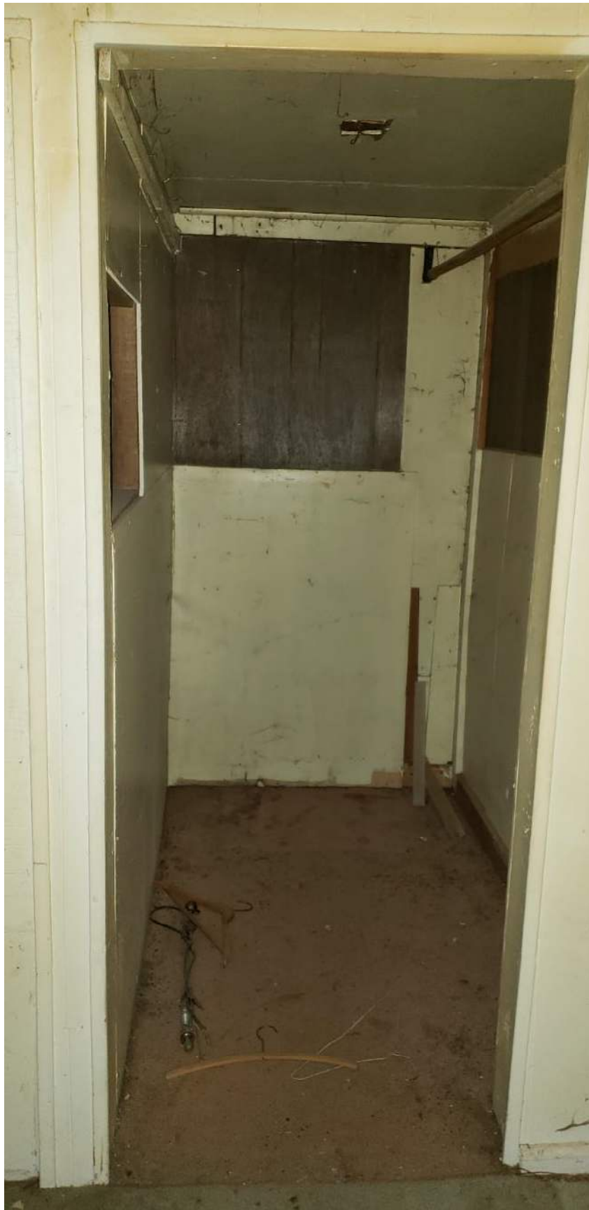
Photo 25. 814 W Coconino Ave ADU closet off bedroom's SW corner to S.
