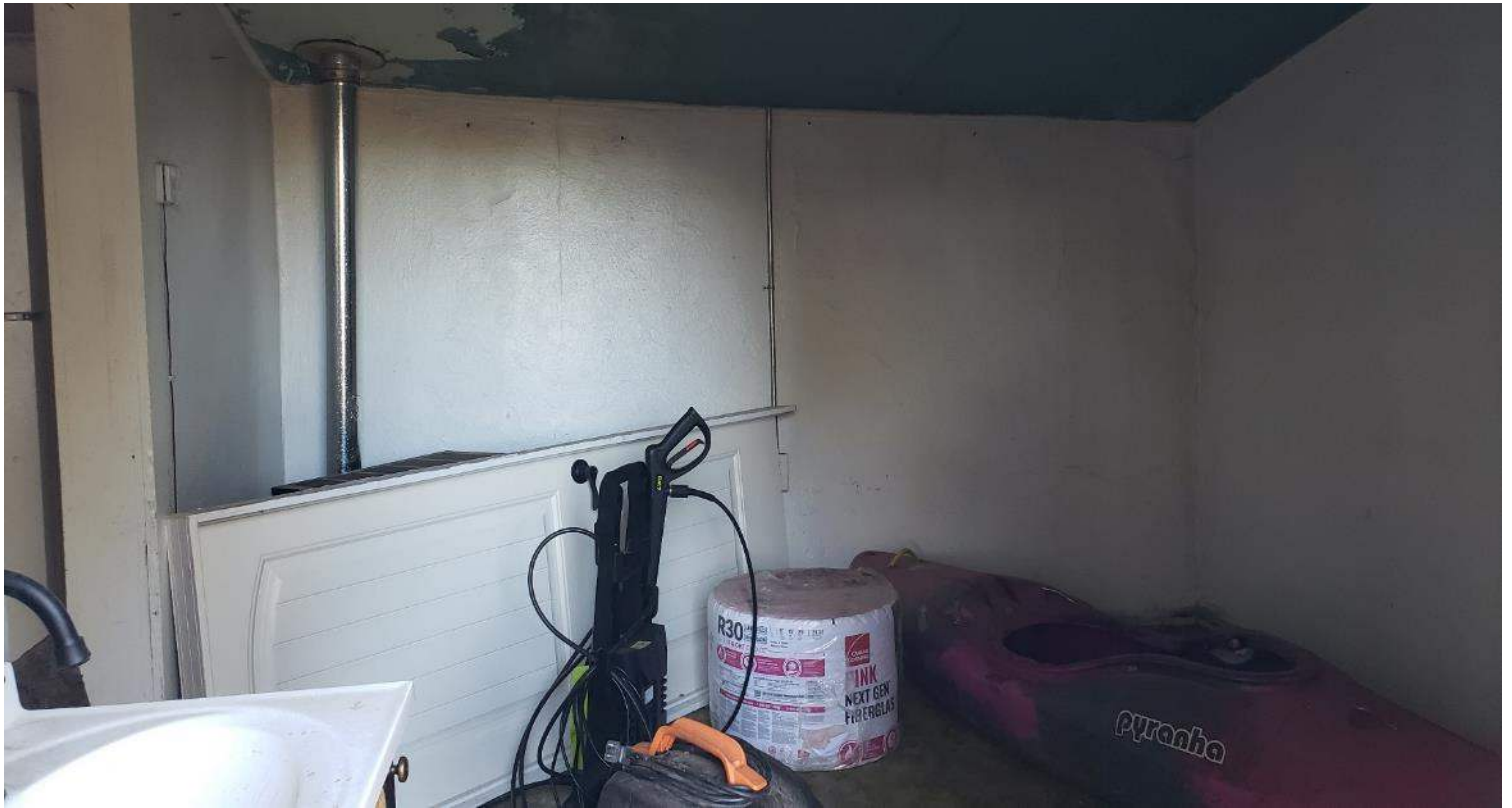
Photos 17–18. 814 W Coconino Ave ADU living room W½ to W with kitchen in background (top) and living room to N from front door (bottom).
