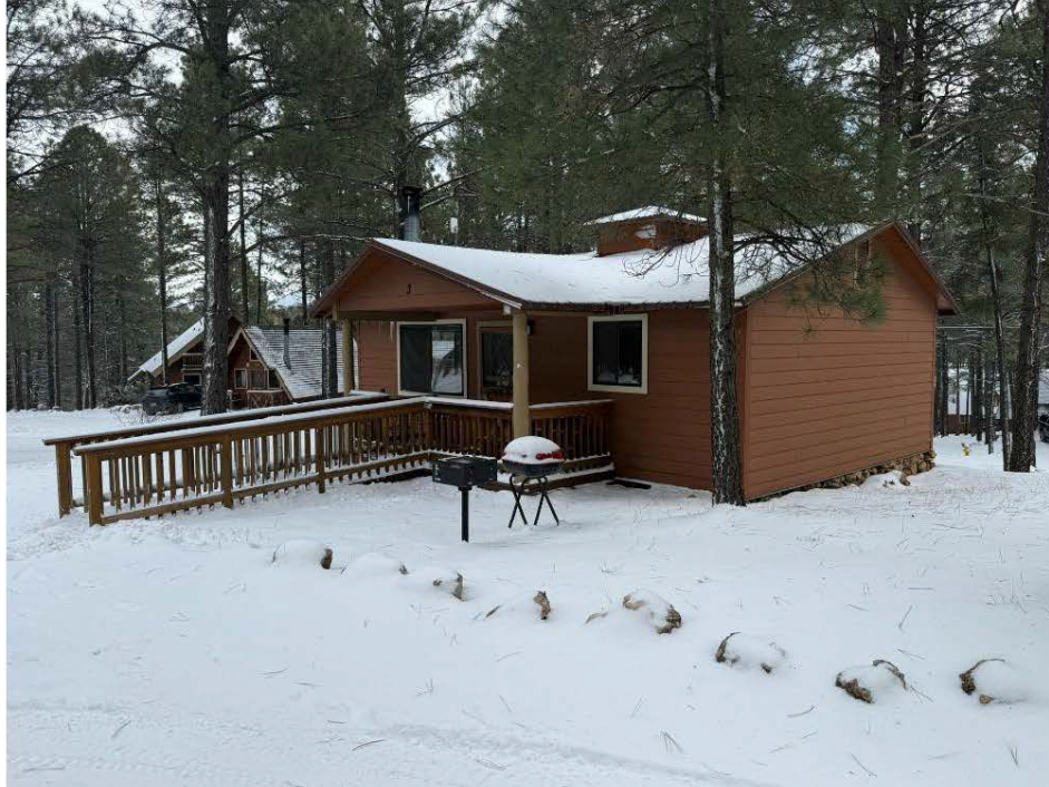
Figure 5-6. Cabin Three (View to the Northeast)
