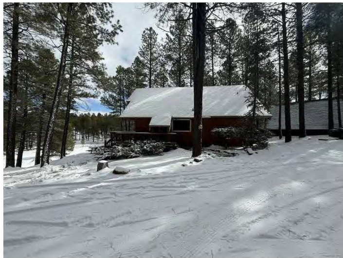
West wall of Cabin Sixteen, view east.
