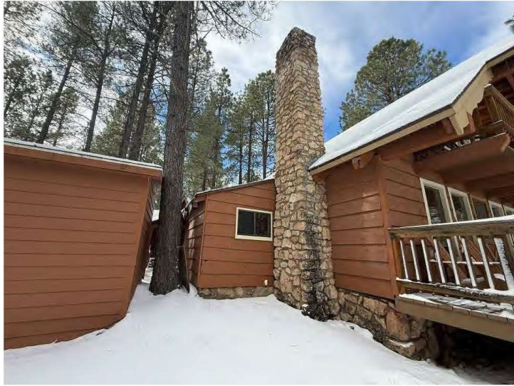
East wall and chimney of Cabin Sixteen, view south-southeast.
