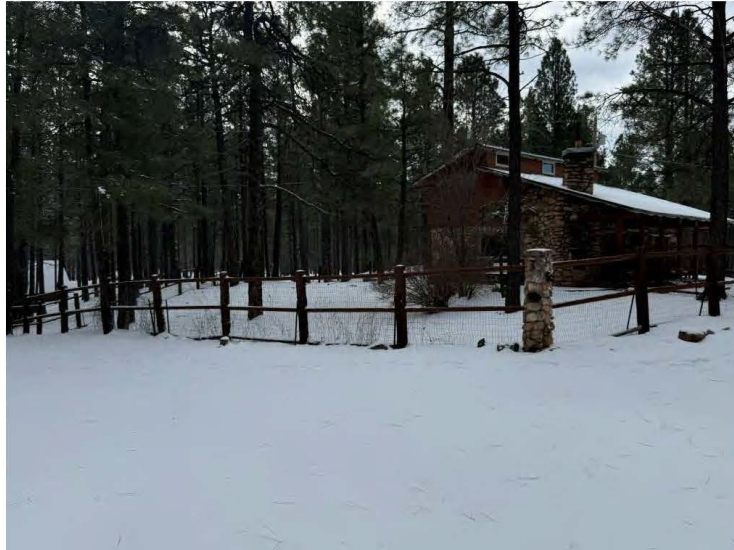
Fenced yard and north wall of Cabin One, view to the southeast.
