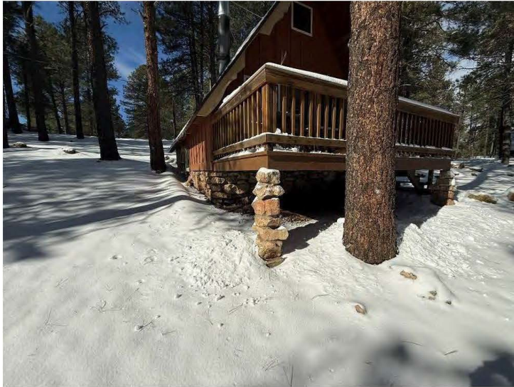
Deck and foundation of Cabin Nine, view southwest.
