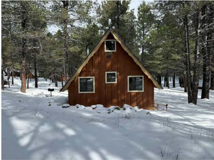
South wall of Cabin Eleven, view north.
