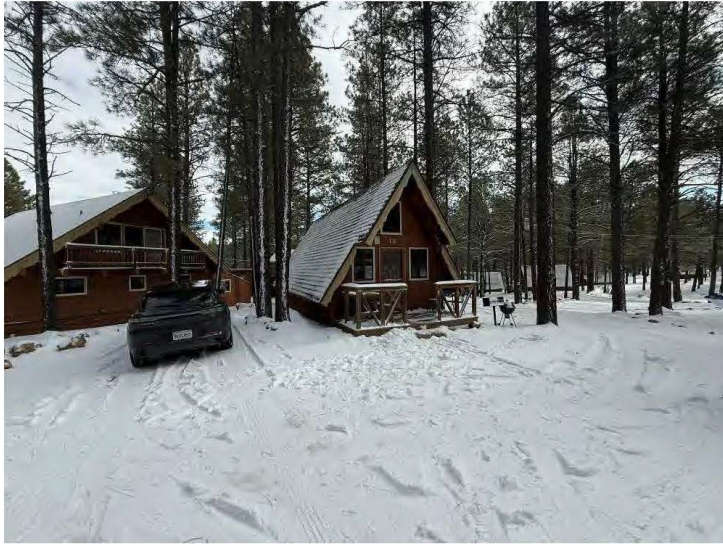
West and south walls of Cabin Nineteen, view north-northeast.
