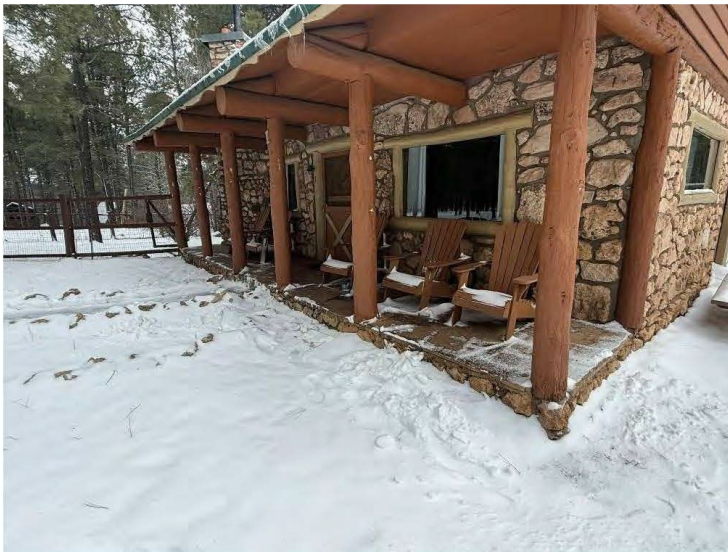
West wall and deck of Cabin One, view to the northeast.
