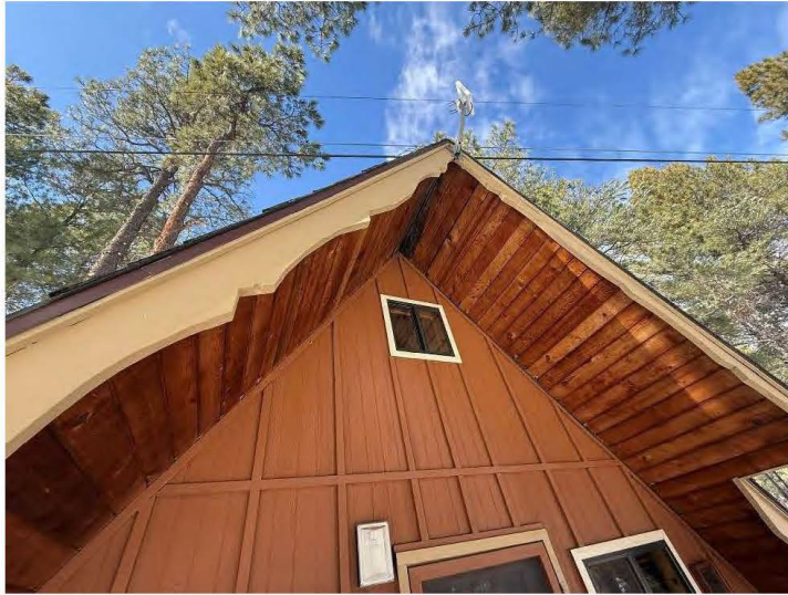
North wall roof and trim details of Cabin Nine, view southwest.
