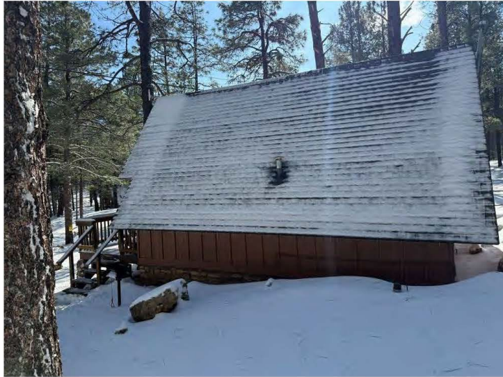
West wall of Cabin Nine, view east.
