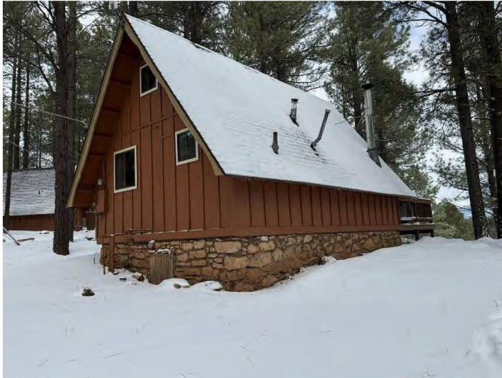
South and east walls of Cabin Six, view northwest.
