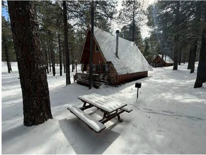
North and west walls of Cabin Thirteen, view southeast.
