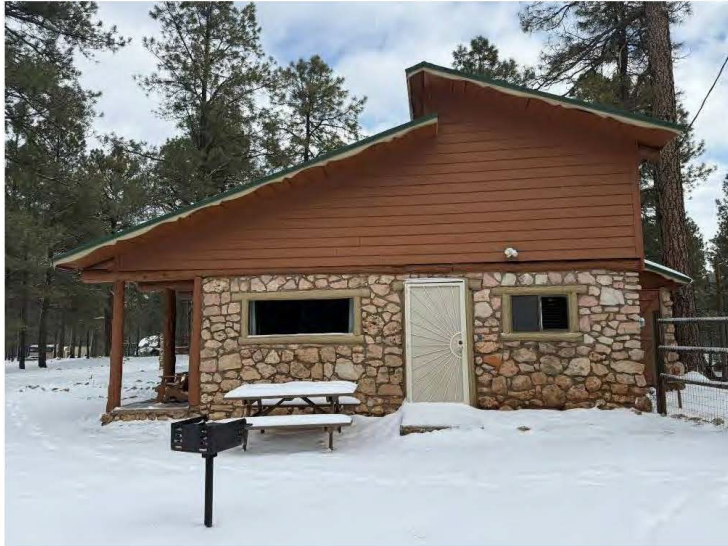
South wall of Cabin One, view to the north.
