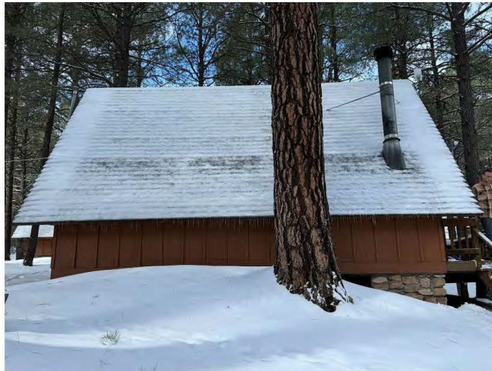
East wall of Cabin Eight, view west.
