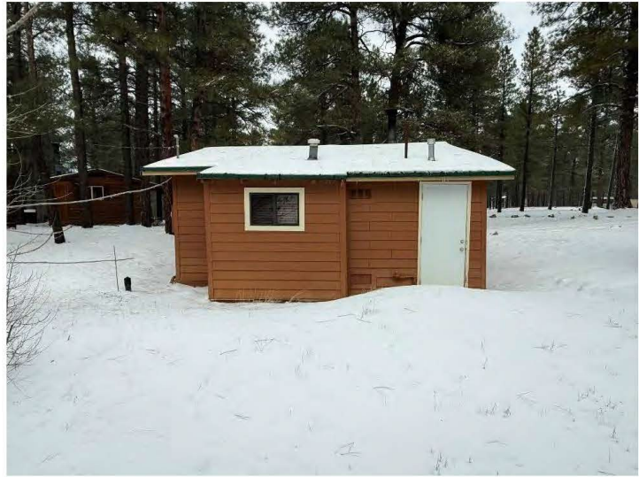
East wall of Cabin Five, view north.
