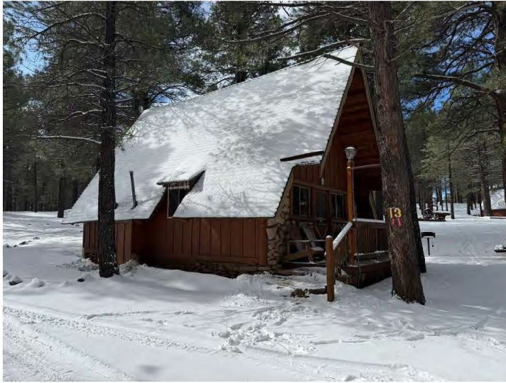
East and north walls of Cabin Thirteen, view southwest.
