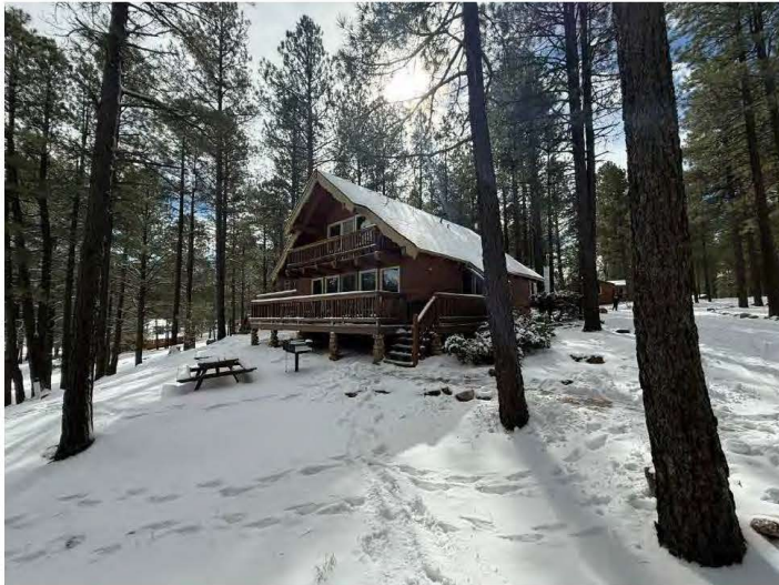
North and west walls of Cabin Sixteen, view southeast.
