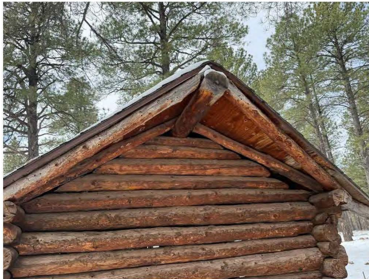
North wall roof details of Small Cabin, view south.
