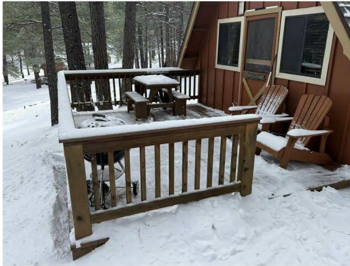
Deck and north wall details of Cabin Six view east-southeast.
