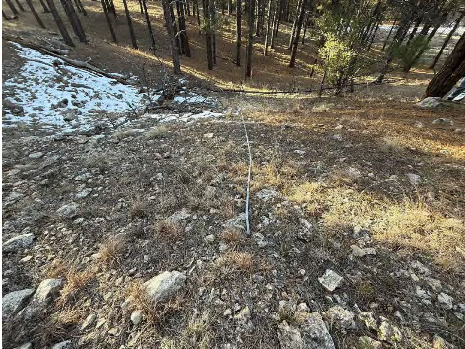
Figure 8 Pipe (IO4), view south.
