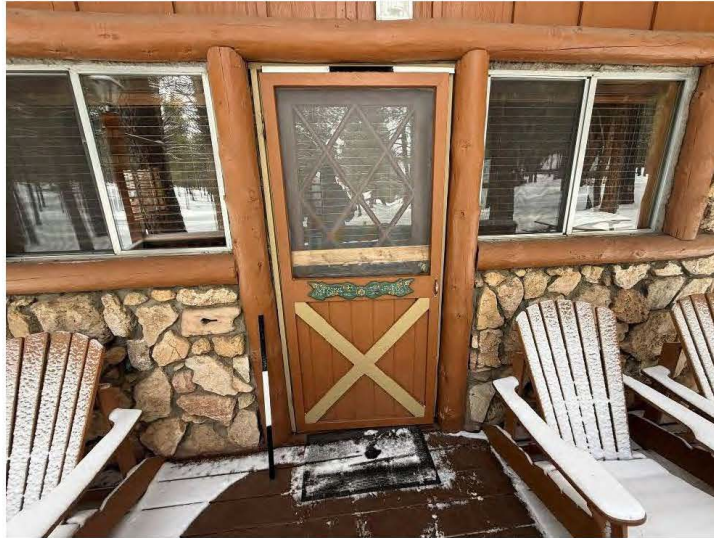
North wall window, door and masonry details of Cabin Thirteen, view south, scale is 3 feet.
