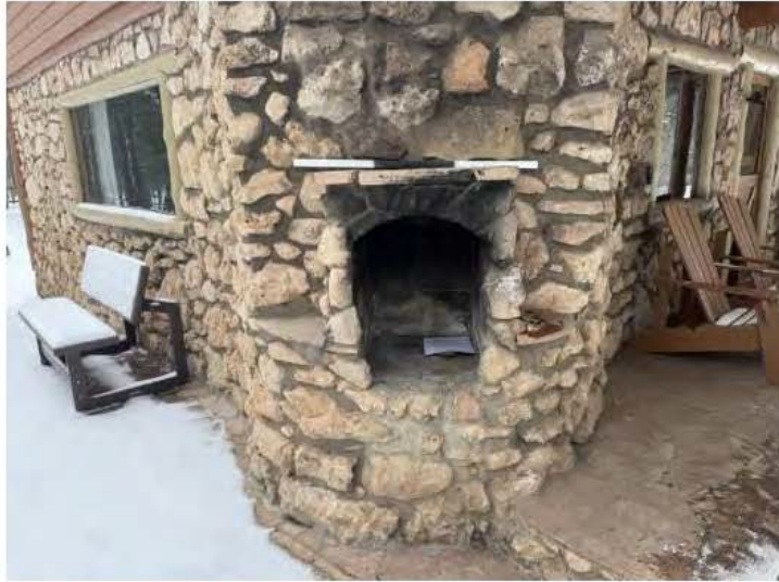
Outdoor fireplace and chimney, connected to interior fireplace.
