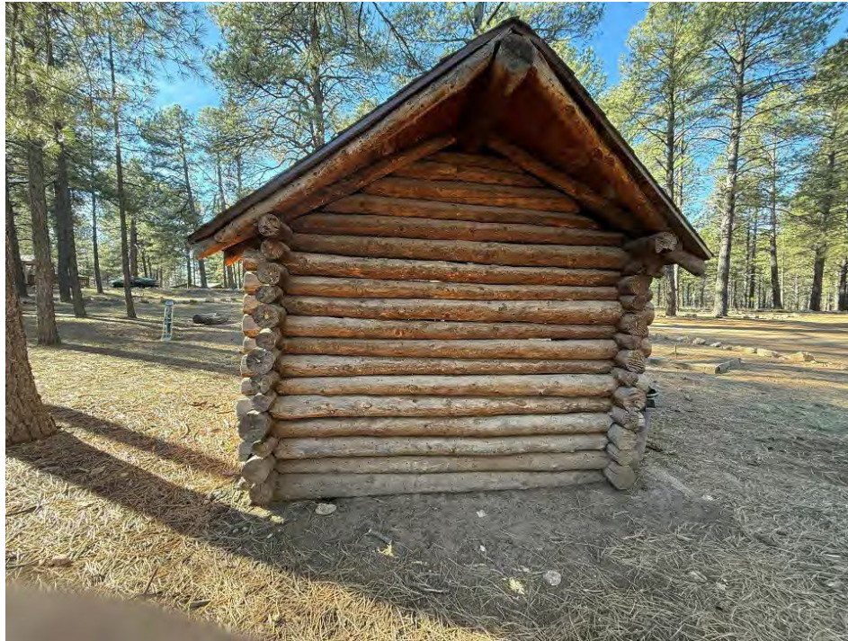
Figure 34 North wall details (IO16), view south.
