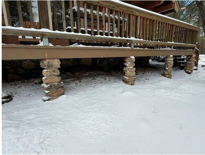
North wall deck and foundation details of Cabin Sixteen, view southwest.
