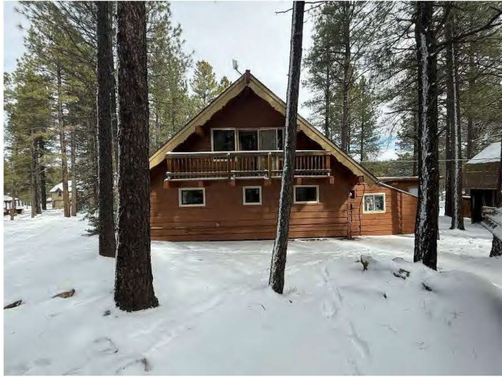
South wall of Cabin Sixteen, view north.
