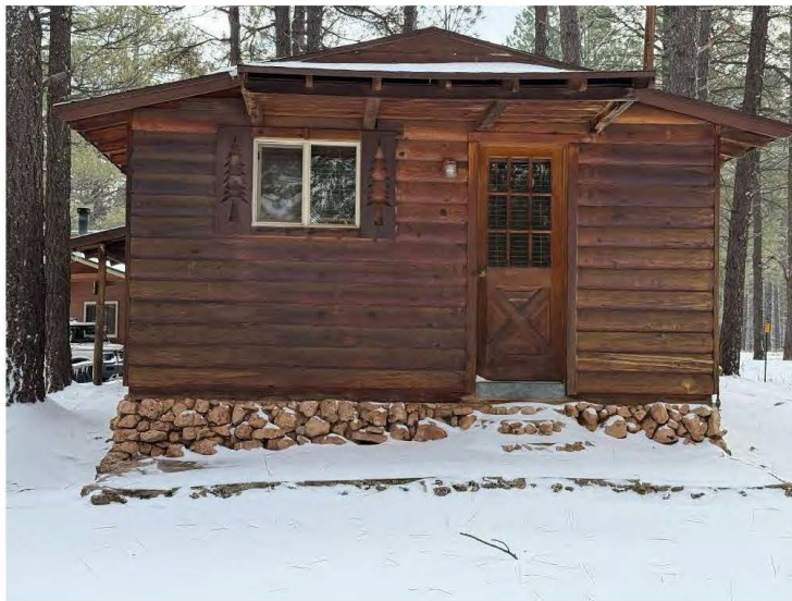
West wall and door of Cabin Two, view to the east.
