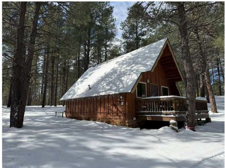
East and north walls of Cabin Eleven, view southwest.
