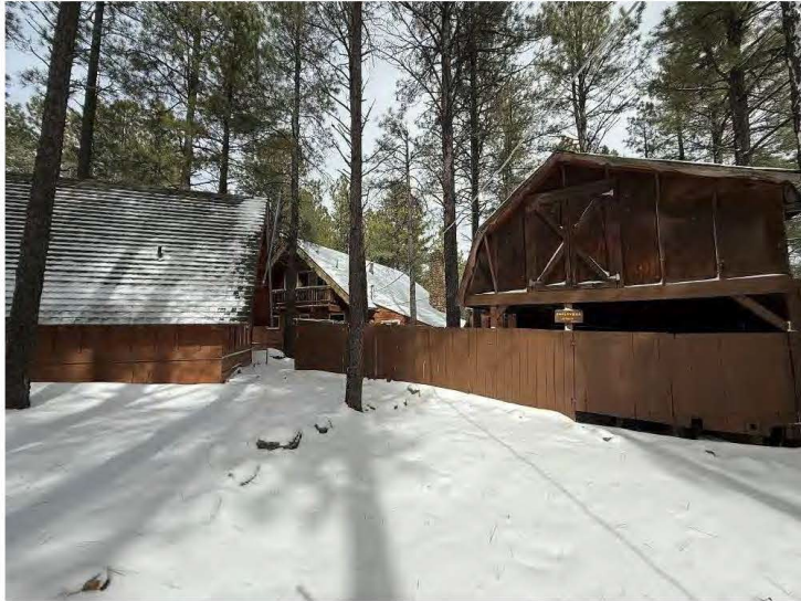
Workshop (right), cabin Nineteen (left) and south/east walls of Cabin Sixteen (center) view northwest.
