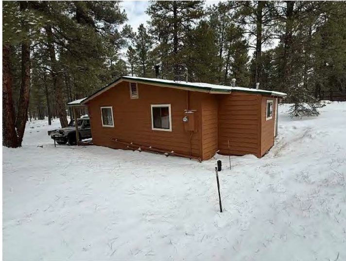
South wall of Cabin Five, view north-northeast.
