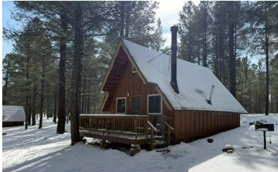
Figure 5-13. Cabin Eleven (View to the Southeast)
