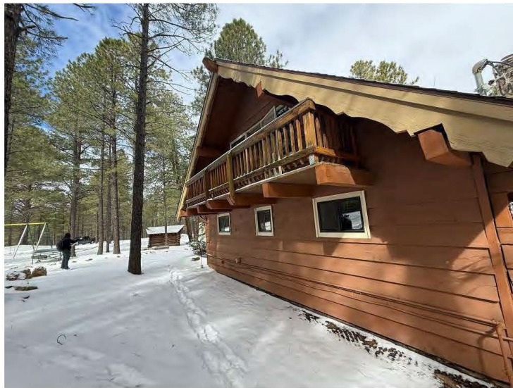
South wall and deck details of Cabin Sixteen, view northwest.
