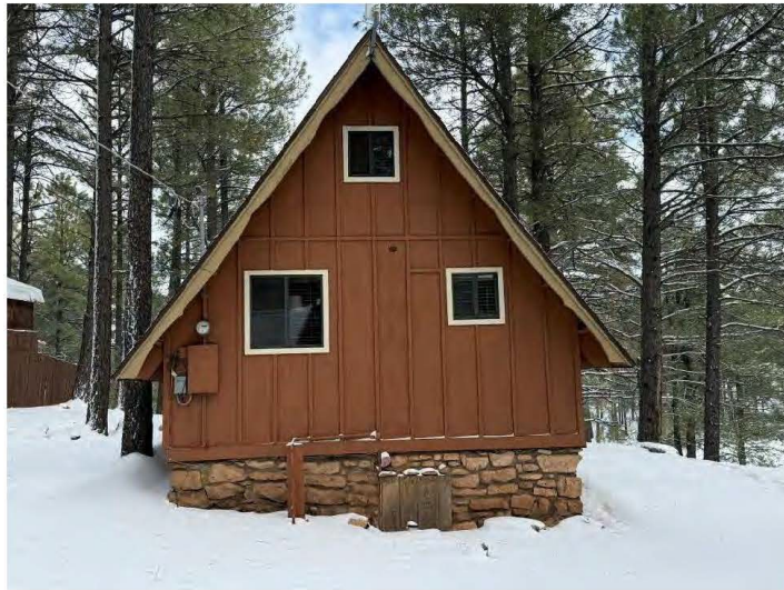
South wall of Cabin Six, view north.
