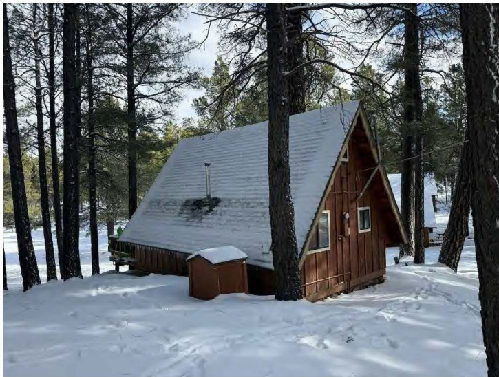
West and south walls of Cabin Eight, view northeast.
