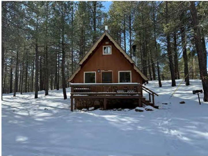
Overview, north wall and deck of Cabin Ten, view south.
