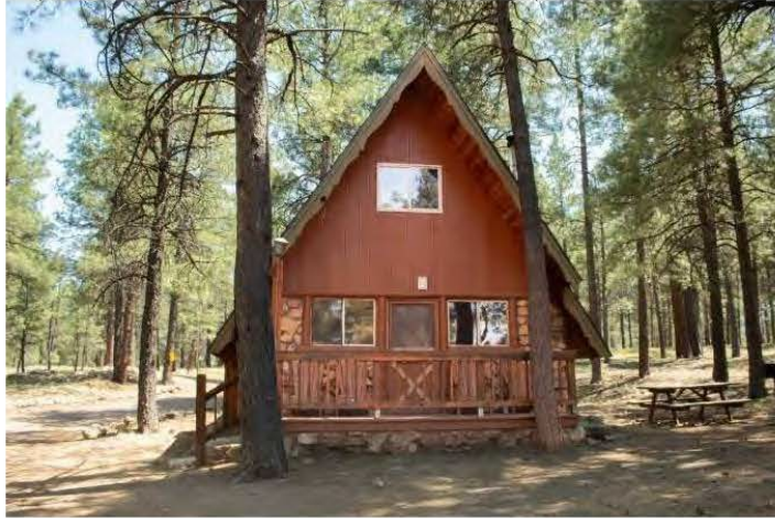
Cabin Thirteen exterior from website.
