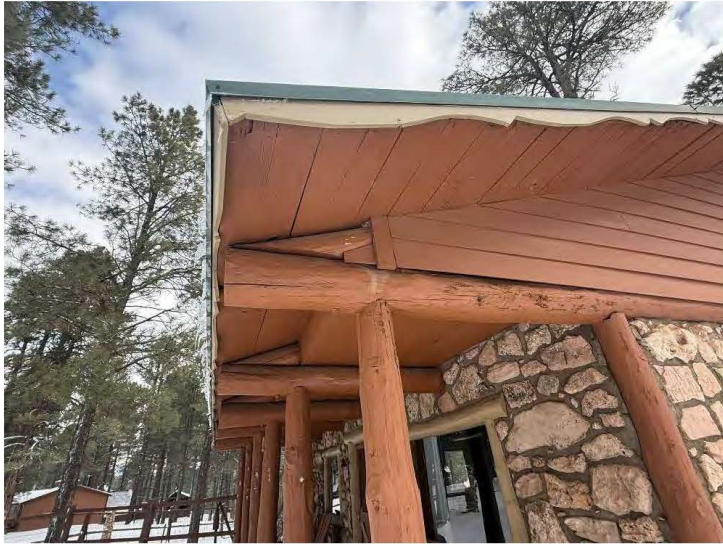
Roof details of Cabin One, view to the northeast.
