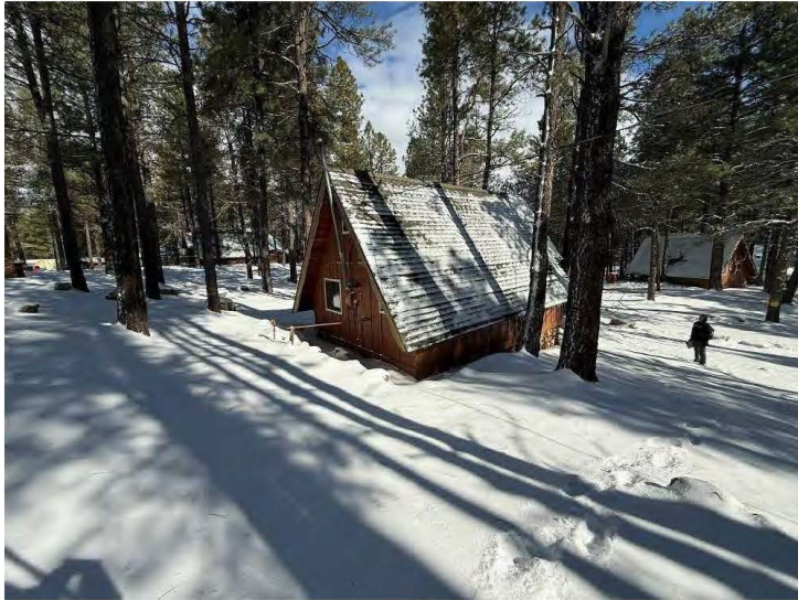
South and east walls of Cabin Nine, view northwest.
