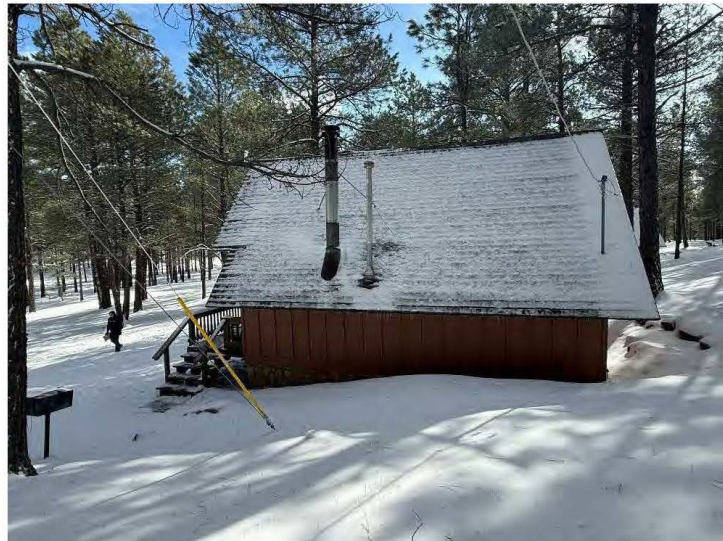
West wall of Cabin Ten, view east.
