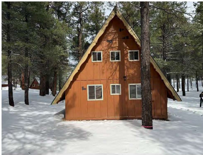
South wall of Cabin Thirteen, view north.
