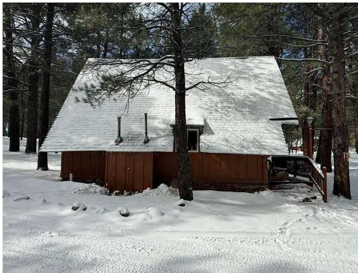
East wall of Cabin Thirteen, view west.
