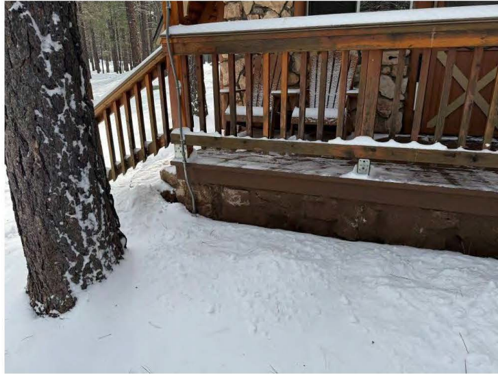
North wall deck details of Cabin Thirteen, view southeast.
