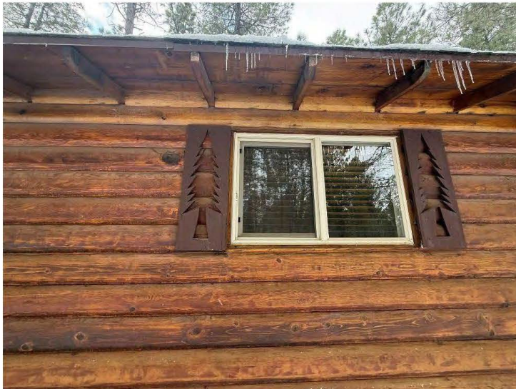
North wall window detail example at Cabin Two, view to the south.
