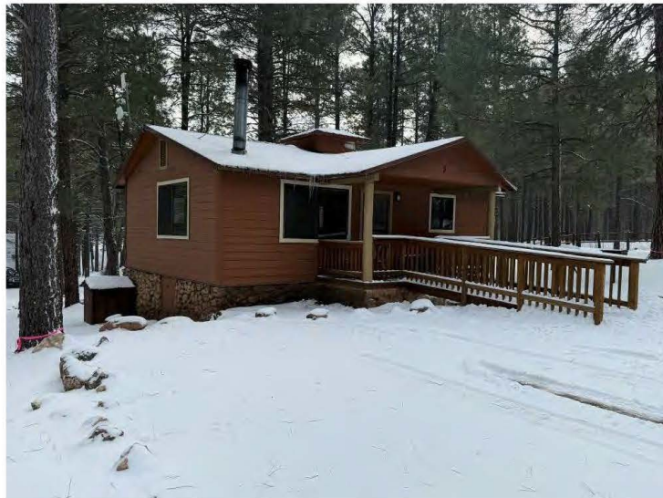
North and west walls of Cabin Three, view southeast.
