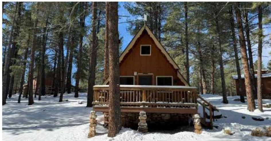
Figure 5-11. Cabin Nine (View to the South)
