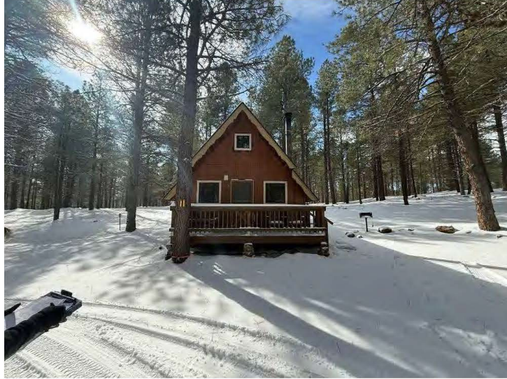
Overview, north wall and deck of Cabin Eleven, view south.
