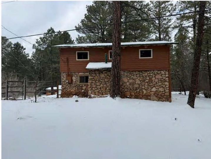
East wall of Cabin One, view to the south.
