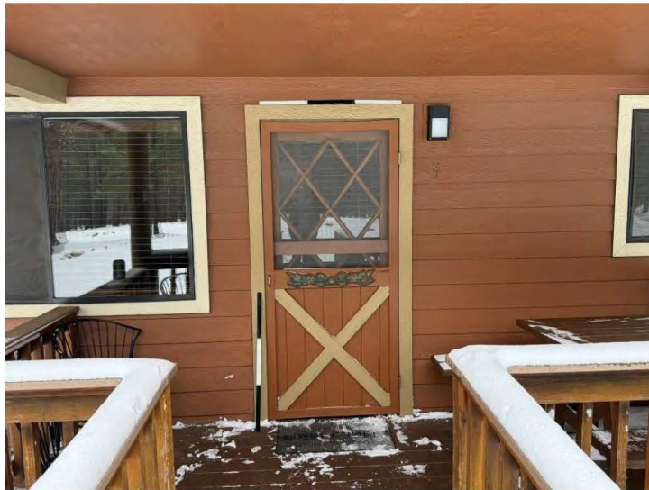
Door of Cabin Three, view east, scale is 3 feet.
