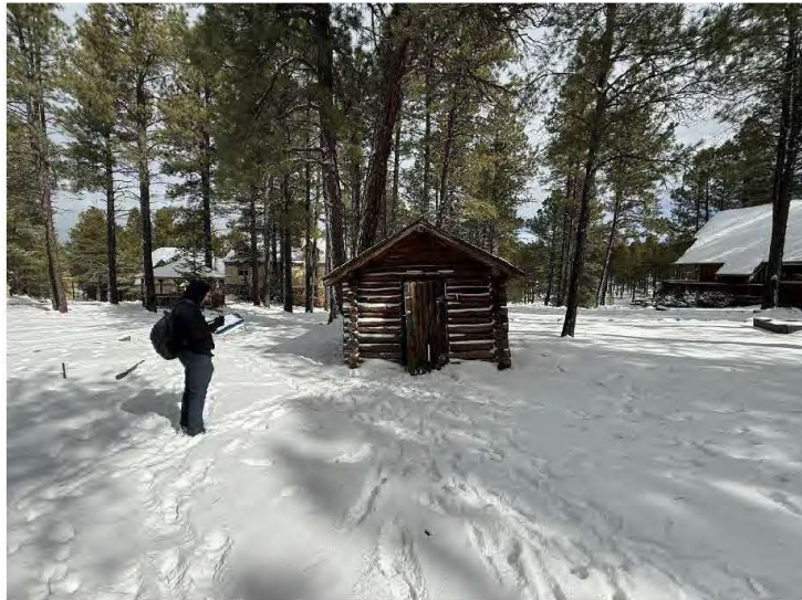
Overview, door and south wall of Small Cabin, view north (Main Inn left).
