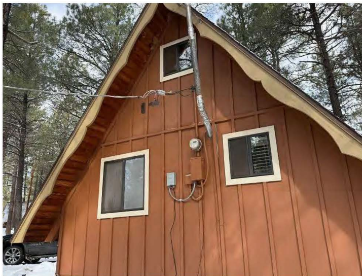
South wall and roof trim details of Cabin Seven, view north-northwest.
