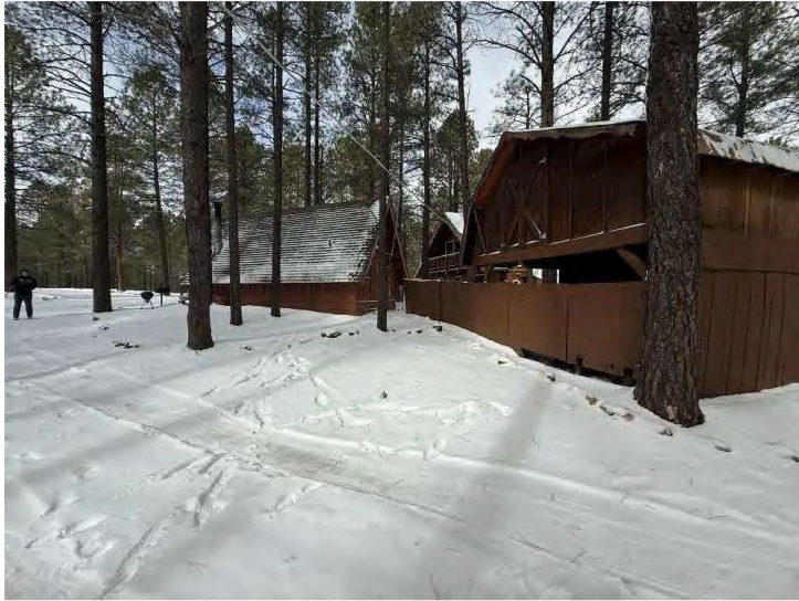
East wall of Cabin Nineteen, view southwest (Workshop right).
