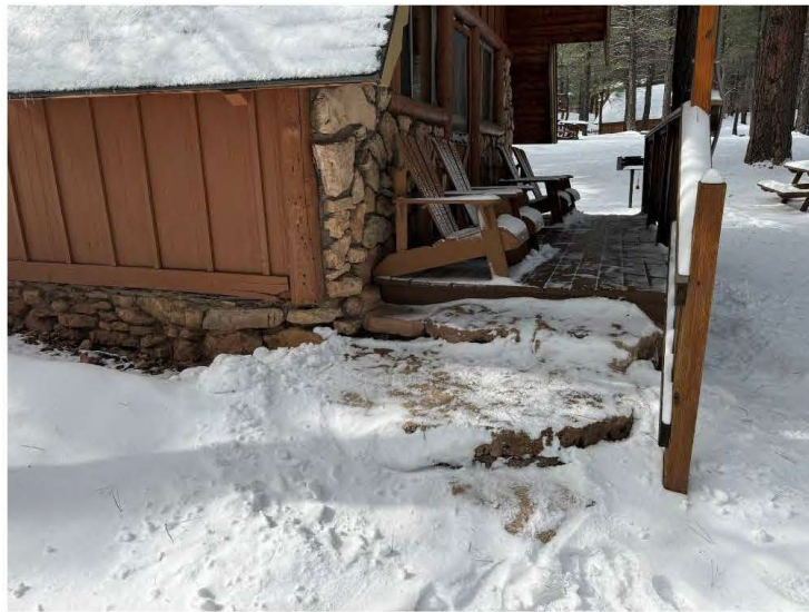
Deck and stair details of Cabin Thirteen, view west.
