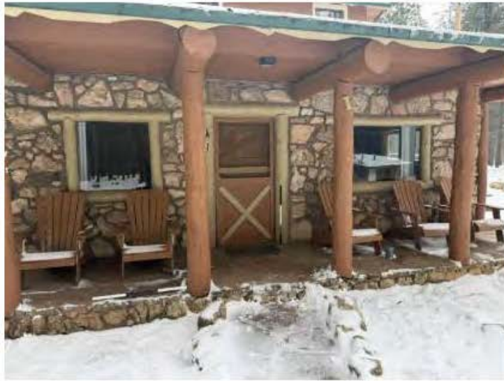
Front door and porch.
