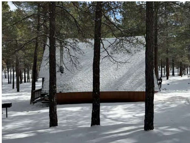
West wall of Cabin Thirteen, view east.
