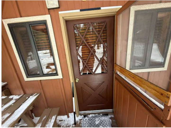
Door of Cabin Nineteen, view north scale is 3 feet.
