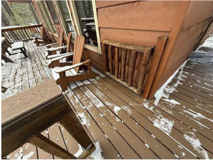
North wall deck and gate of Cabin Sixteen, view southeast.
