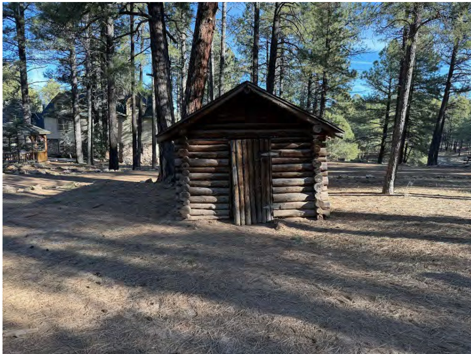
Figure 32 Overview (IO16), view north.
