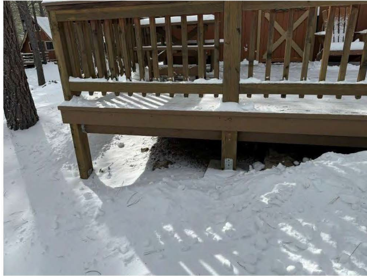
Deck details of Cabin Six, view southeast.
