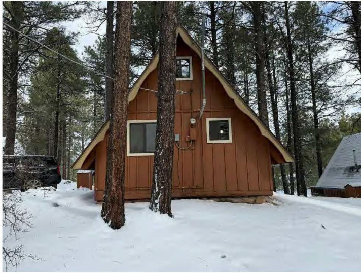
South wall of Cabin Seven, view north.
