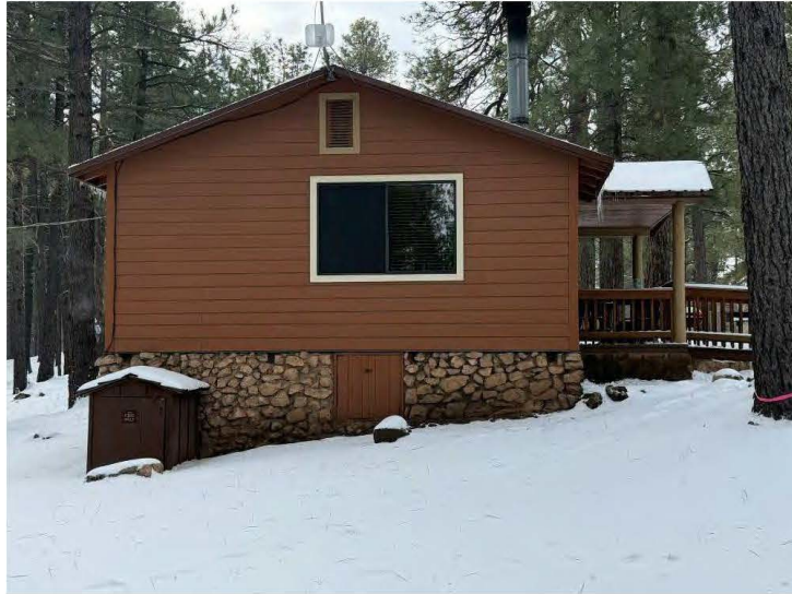
North wall of Cabin Three, view south.
