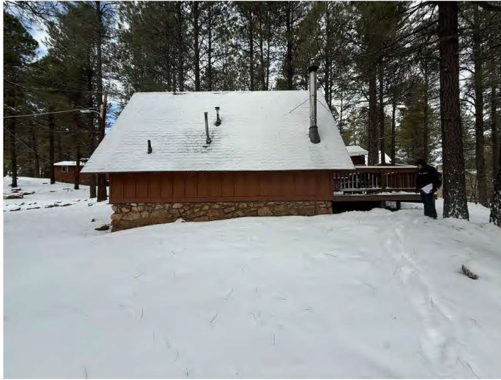
East wall of Cabin Six, view west.
