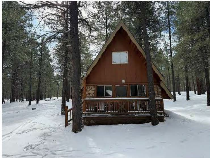
Overview, north wall and deck of Cabin Thirteen, view south.
