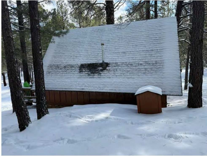
West wall of Cabin Eight, view east.
