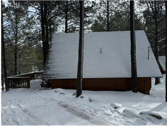
West wall of Cabin Six, view east.
