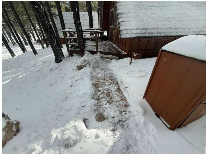
Path and deck at Cabin Seven, view east.
