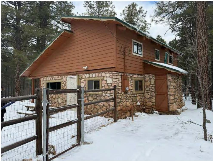
South wall of Cabin One, view to the northwest.
