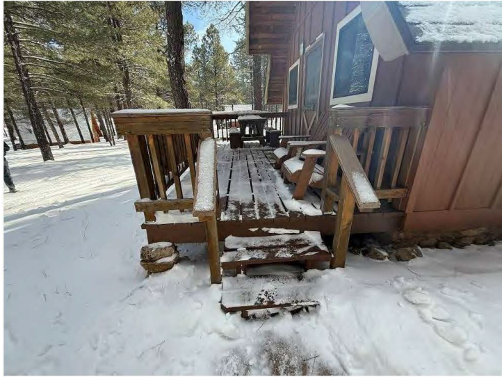
Deck and stairs of Cabin Eleven, view east.
