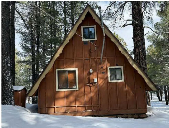
South wall (details and decoration) of Cabin Eight, view north.
