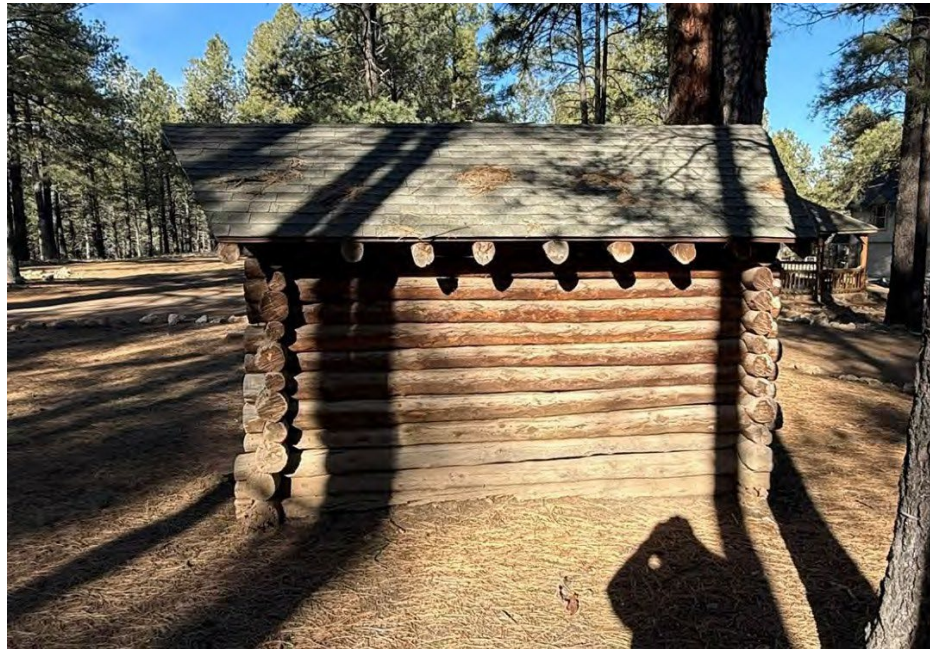
Figure 35 East wall details (IO16), view west.
