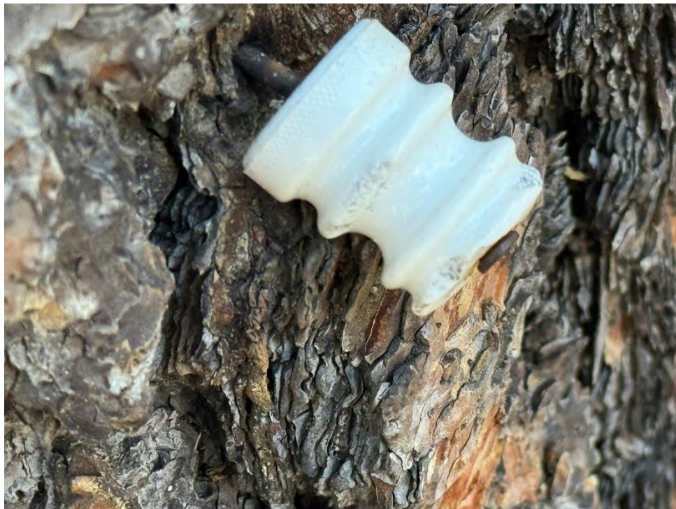
Figure 15 Closer view of insulator (IO10), view east southeast.
