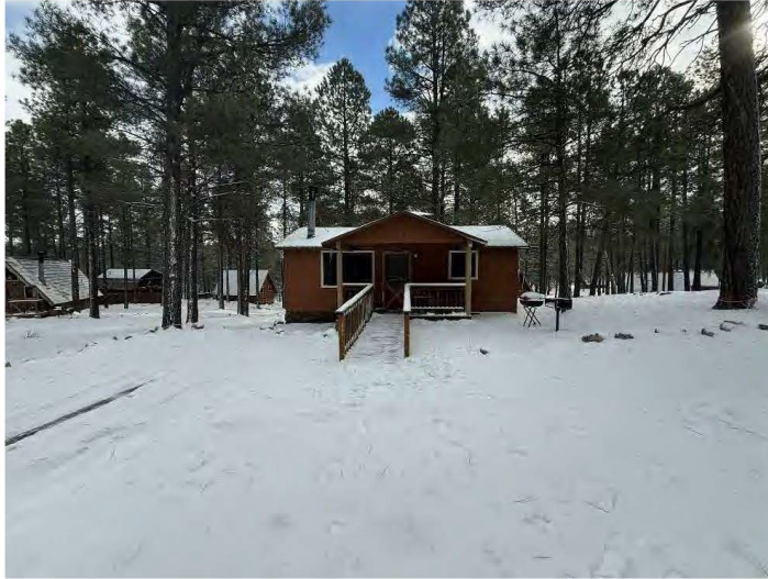
Overview and west wall of Cabin Three, view east.
