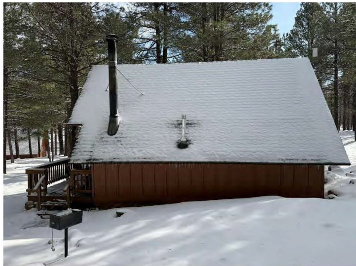
West wall of Cabin Eleven, view east.
