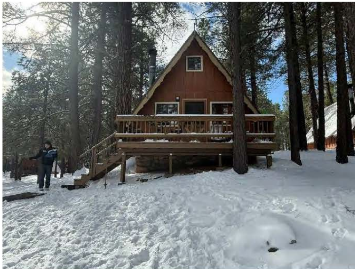
Overview and north wall of Cabin Eight, view south.
