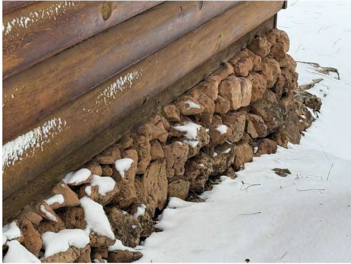
North wall foundation detail example at Cabin Two, view to the southwest.
