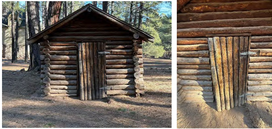
Figure 33 South wall details & doorway (IO16), view north.
