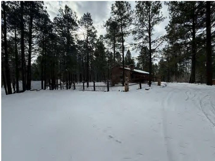
Overview of Cabin One, view to the southeast.
