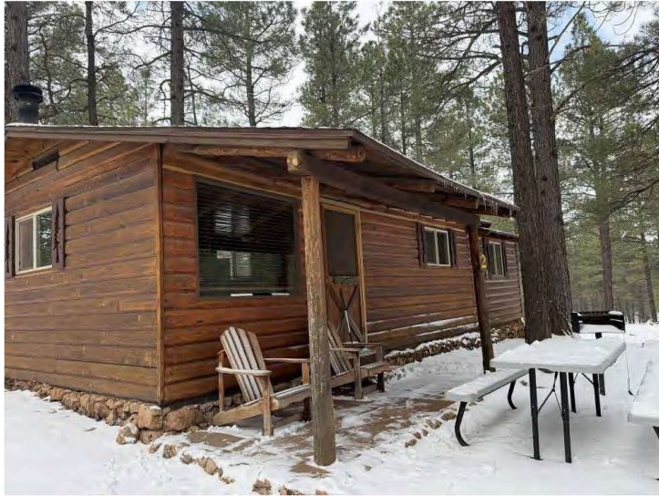
North wall and deck of Cabin Two, view to the southwest.
