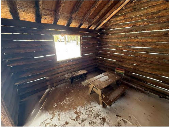
Interior details of Small Cabin, view northwest.
