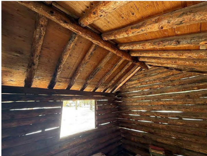
Interior roof details of Small Cabin, view northwest.
