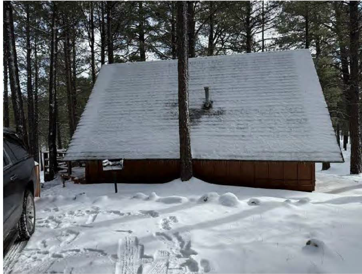
West wall of Cabin Seven, view east.
