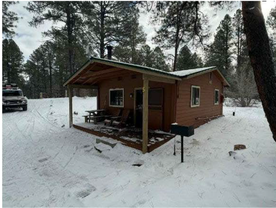
Figure 5-7. Cabin Five (View to the East-Northeast)
