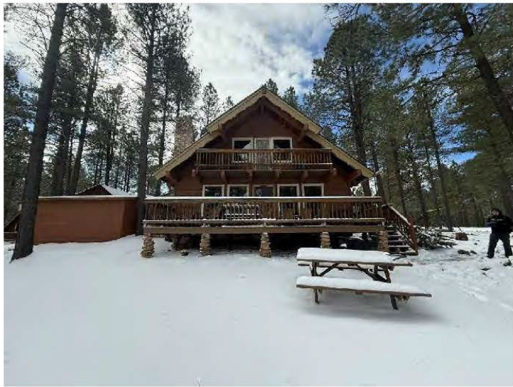
Overview, north wall and deck of Cabin Sixteen, view south.
