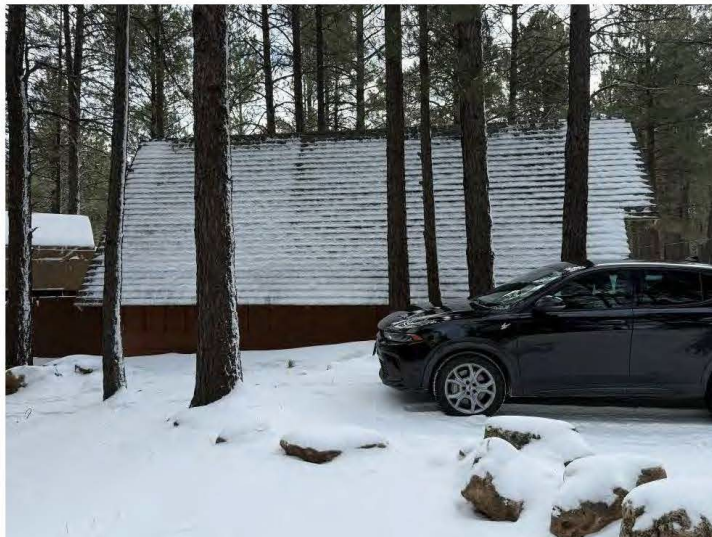
West wall of Cabin Nineteen, view east.
