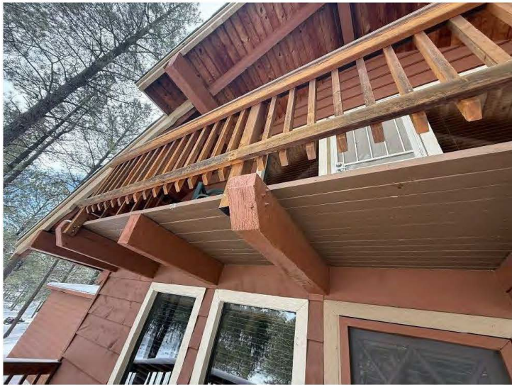
North wall second story deck details of Cabin Sixteen, view southeast.
