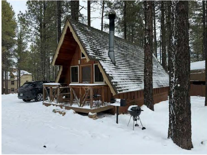
South and east walls of Cabin Nineteen, view northwest (Main Inn left).
