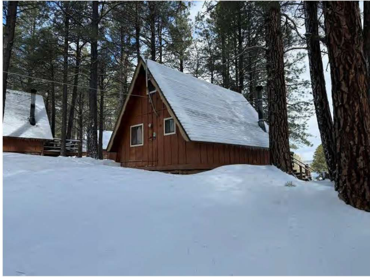
South and east walls of Cabin Eight, view northwest.
