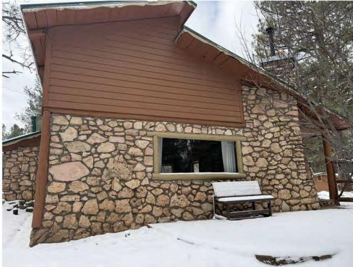
North wall of Cabin One, view to the south.
