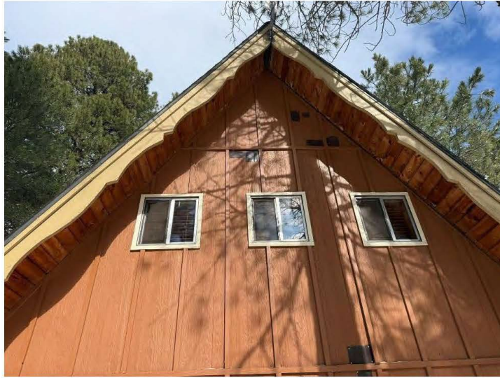
South wall window, roof and trim details of Cabin Thirteen, view north.
