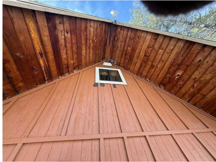
North wall window and roof details of Cabin Ten, view south.
