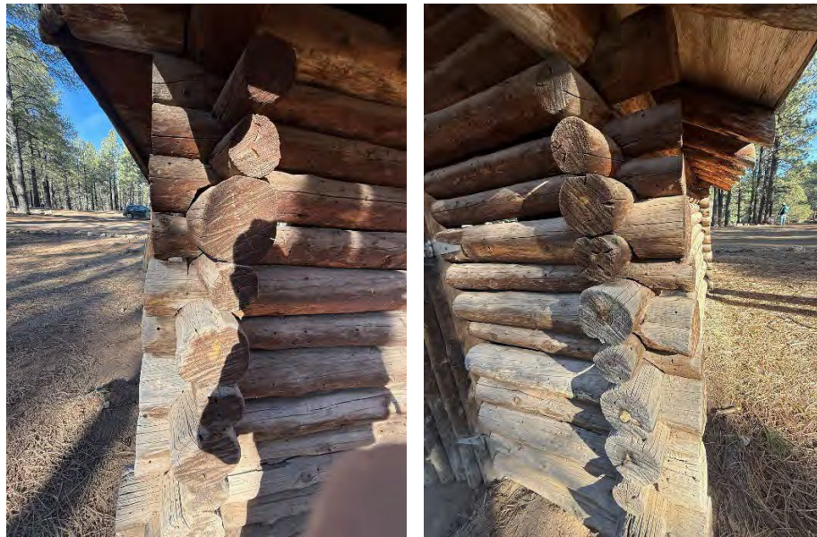
Figure 36 South wall corner details (IO16), view north.
