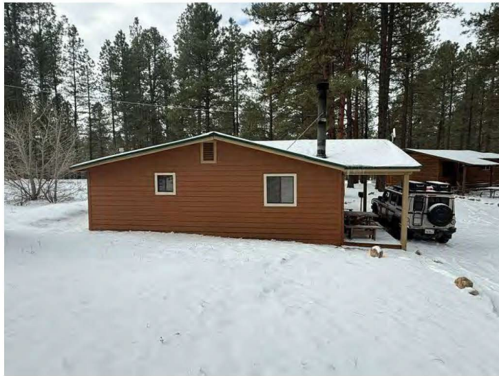
North wall of Cabin Five, view south.
