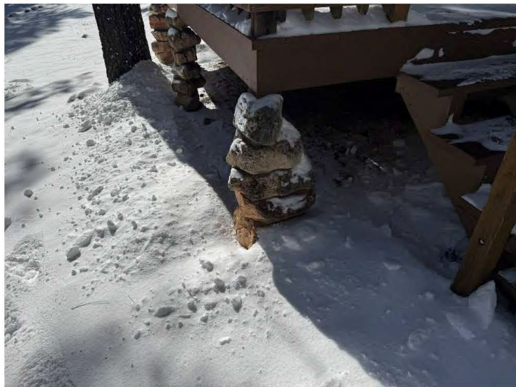
Deck details of Cabin Nine, view southeast.
