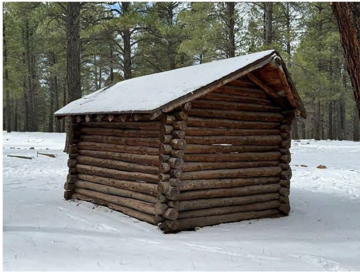
East and north walls of Small Cabin, view southwest.
