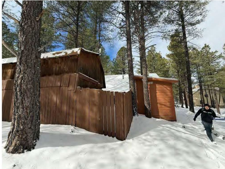
Workshop (left), shed, and fence adjacent and east of Cabin Sixteen, view west.
