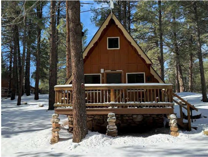
North wall and deck of Cabin Nine, view south.
