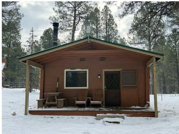
West wall of Cabin Five, view east.
