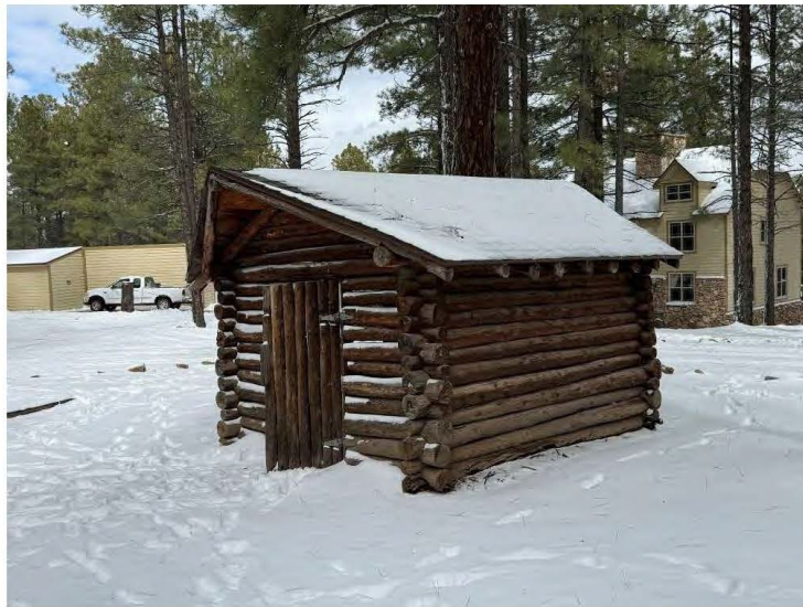
South and east walls of Small Cabin, view northwest (Main Inn rear).
