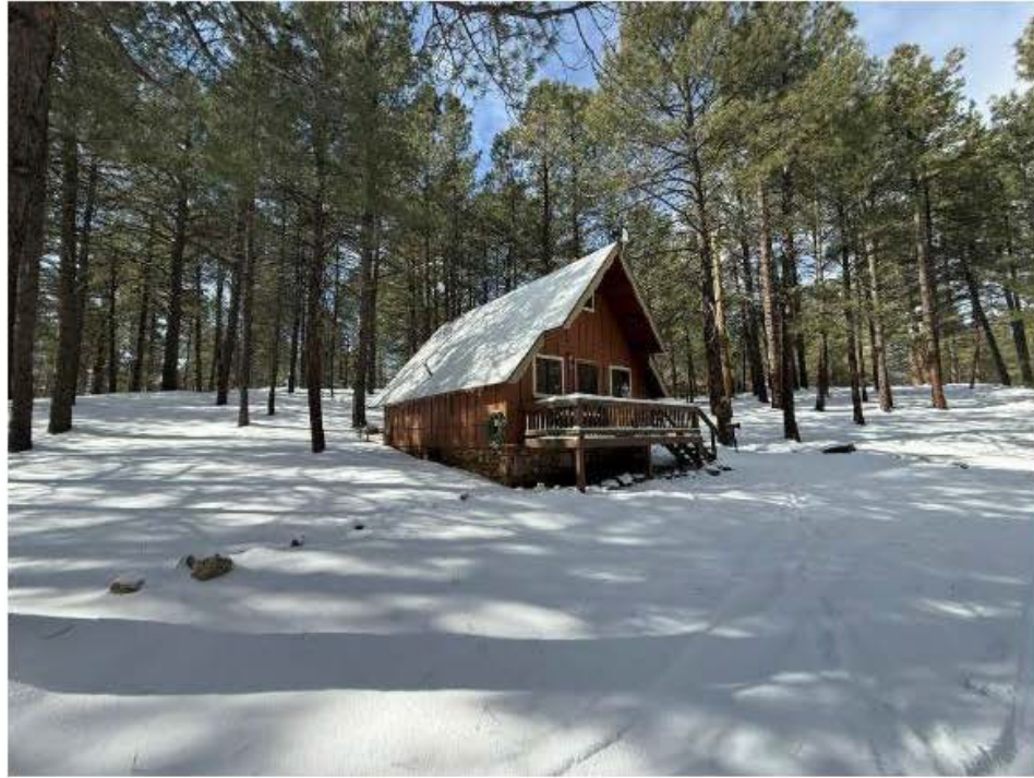
Figure 5-12. Cabin Ten (View to the Southwest)
