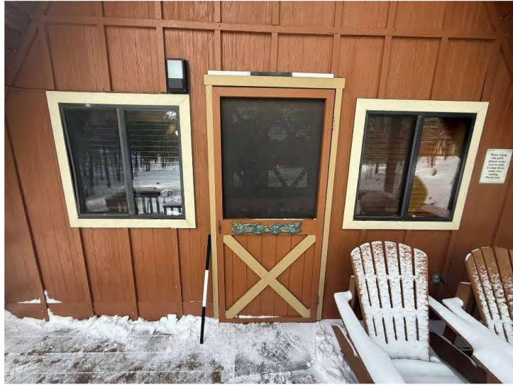
Window and door details of north wall of Cabin Eight, view south, scale is 3 feet.
