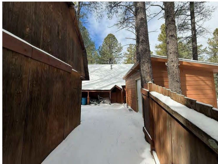
View between Workshop and fence of east entrance of Cabin Sixteen, view west.
