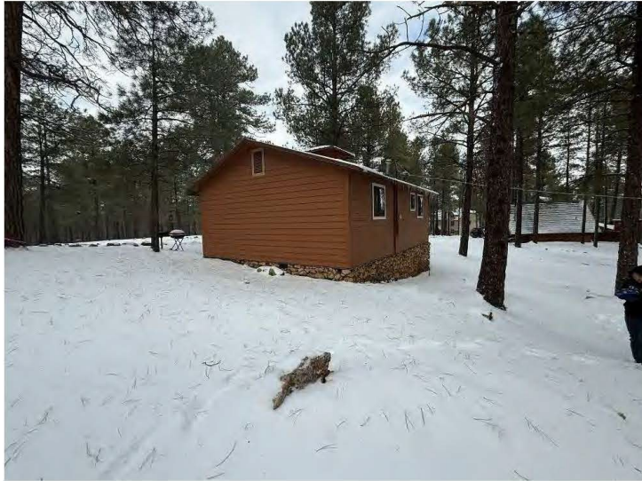
South and east walls of Cabin Three, view northwest.
