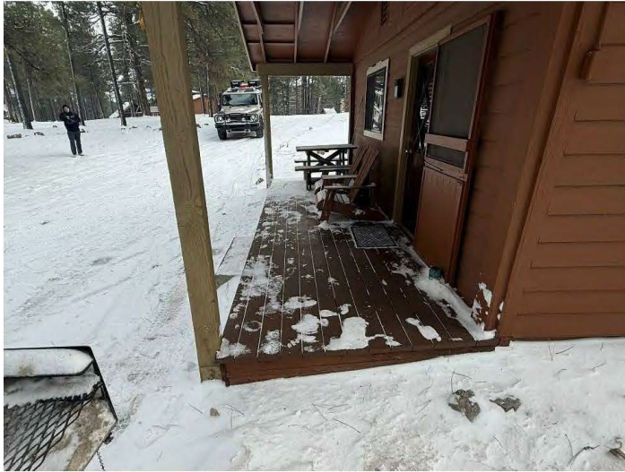
Deck at Cabin Five, view north.
