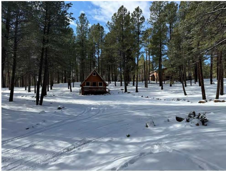
Overview and north wall of Cabin Nine, view south.
