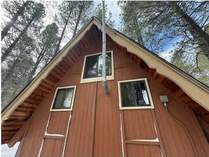
North wall window and trim details of Cabin Nineteen, view south.
