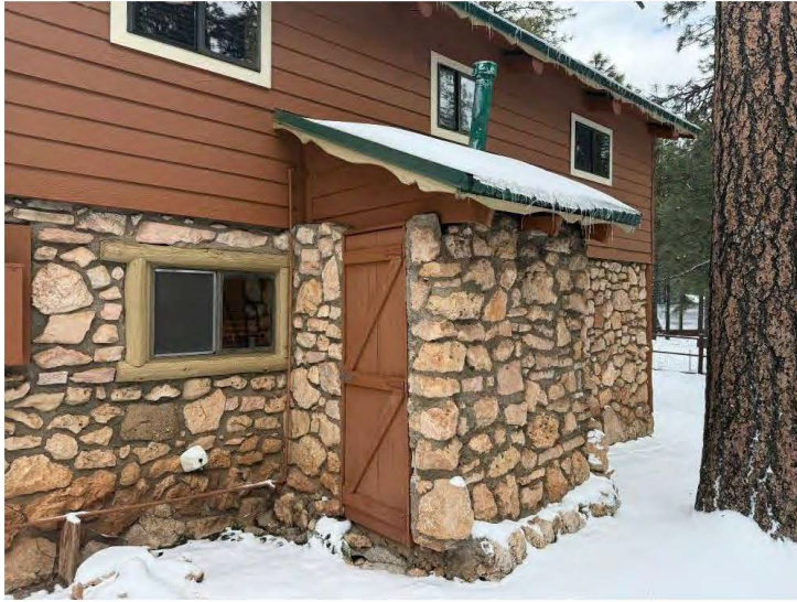
East wall of Cabin One, view to the northwest.
