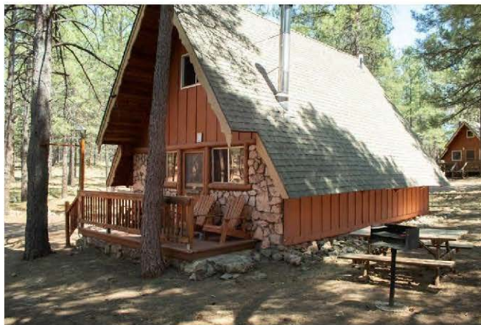
Cabin Thirteen exterior from website.
