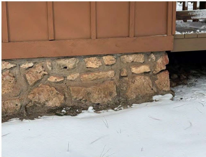
East wall foundation details of Cabin Six, view west.
