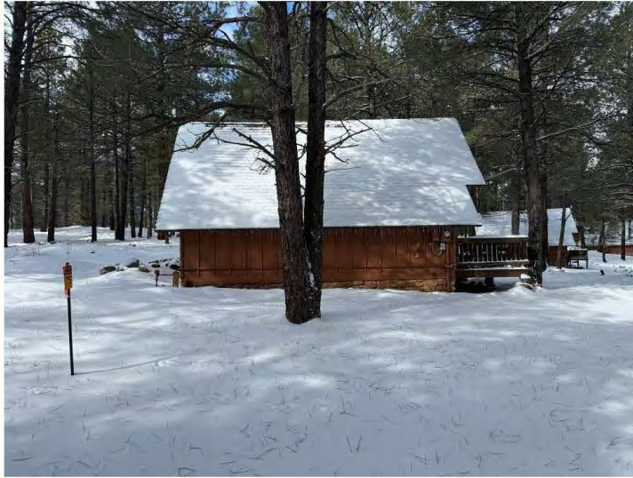
East wall of Cabin Eleven, view west.
