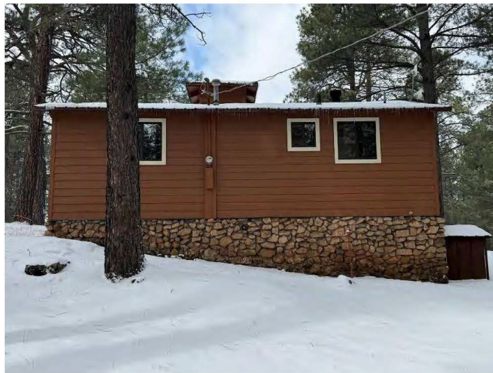
East wall of Cabin Three, view west.
