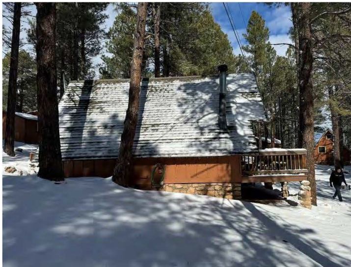
East wall of Cabin Nine, view west.
