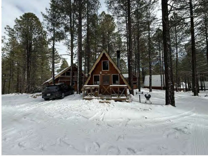
Overview, south wall and deck of Cabin Nineteen, view north.
