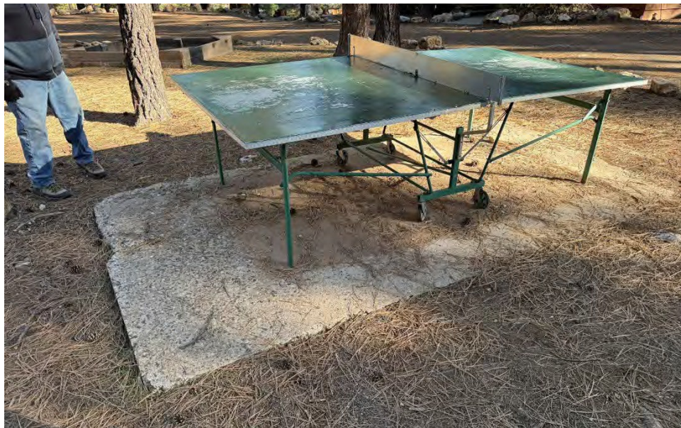
Figure 19 Concrete pad (IO17), view northeast.
