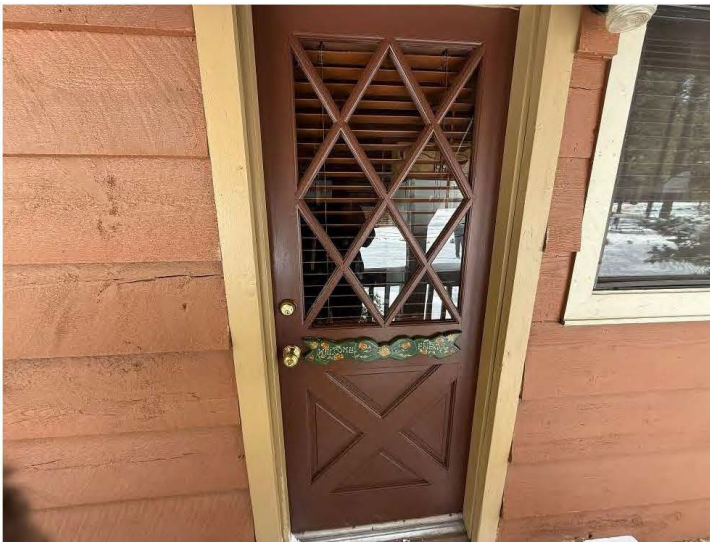
West door of Cabin Sixteen, view east.
