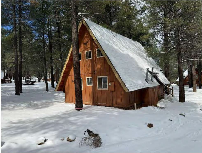
South and east walls of Cabin Thirteen, view northwest.
