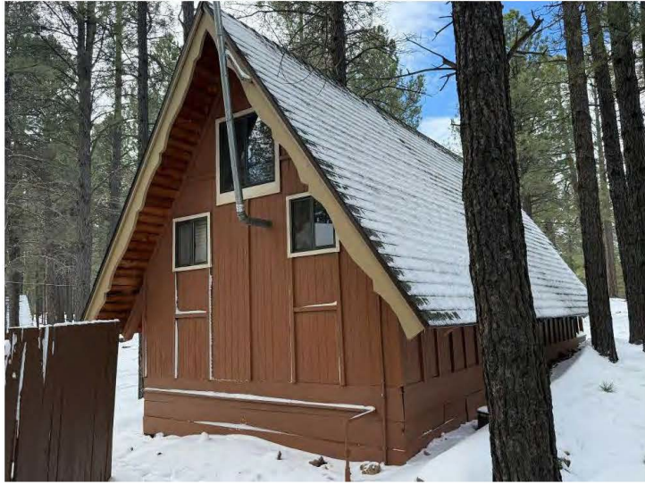
North and west wall of Cabin Nineteen, view southeast.
