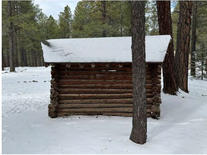
East wall of Small Cabin, view west.
