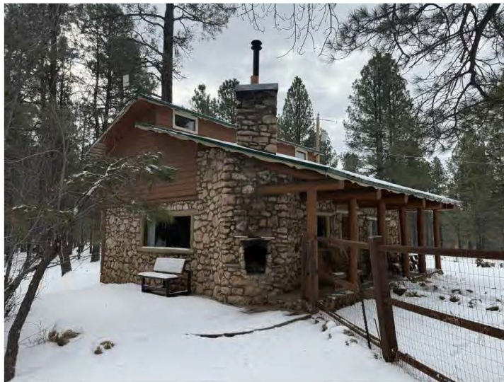
View of Cabin One, view to the southeast.
