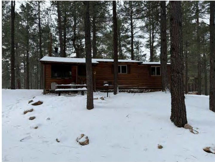
North wall of Cabin Two, view to the south.
