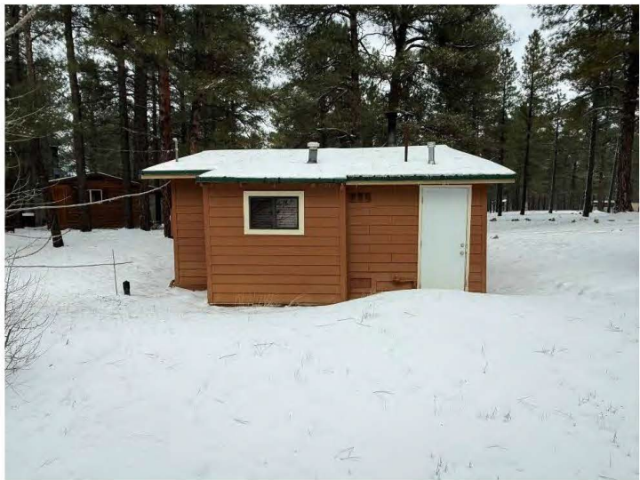
East wall of Cabin Five, view north.
