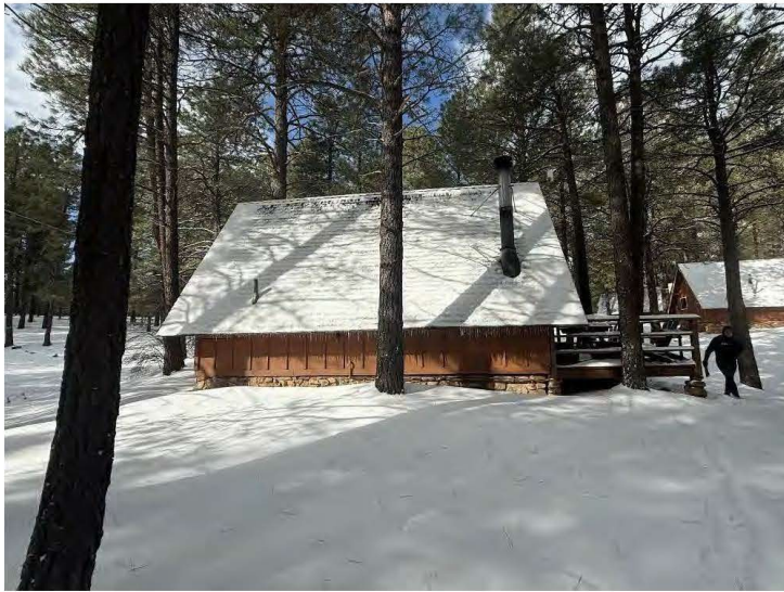
East wall of Cabin Seven, view west.
