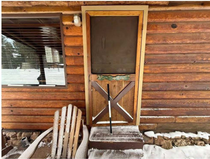
Door of Cabin Two, view to the south, scale is 3 feet.
