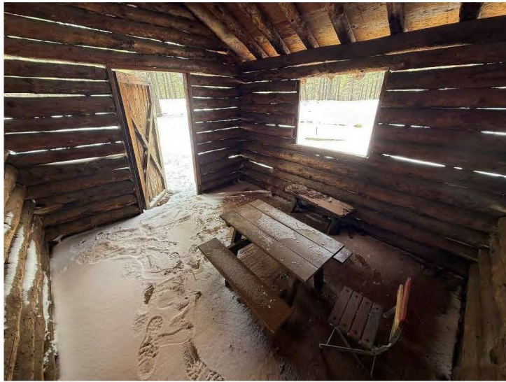
Interior details of Small Cabin, view southwest.
