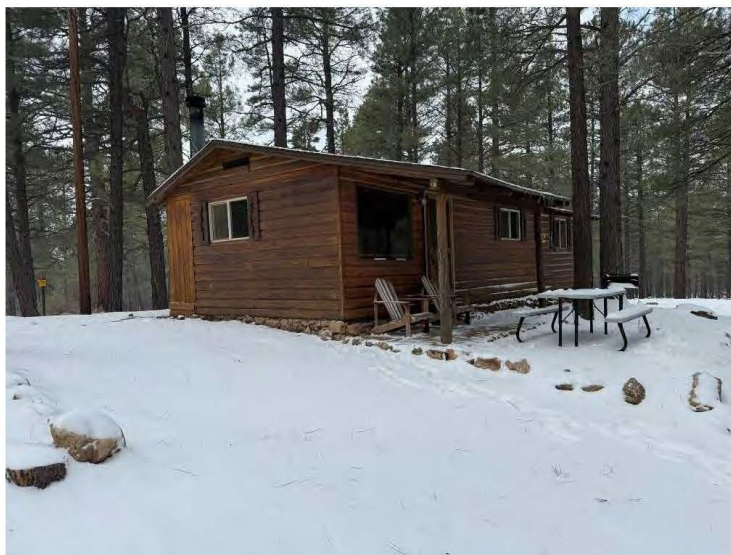
North and east walls of Cabin Two, view to the southwest.
