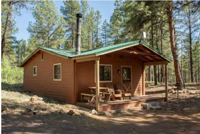
Cabin Five exterior from website.
