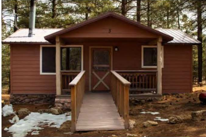
Cabin Three exterior from website.
