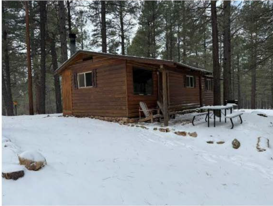
Figure 5-4. Cabin Two (View to the Southeast)
