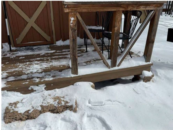
Deck details of Cabin Nineteen, view north.
