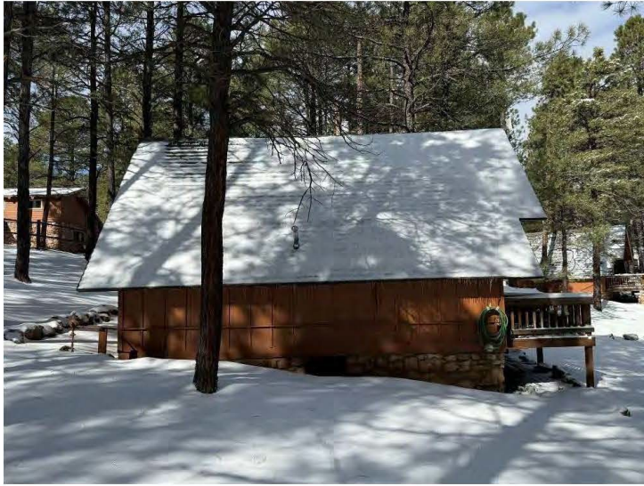
East wall of Cabin Ten, view west.
