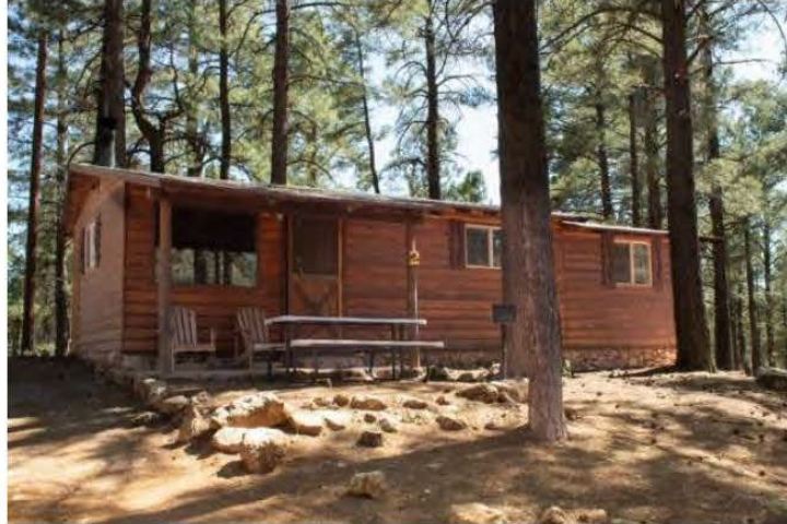
Cabin Two exterior from website.
