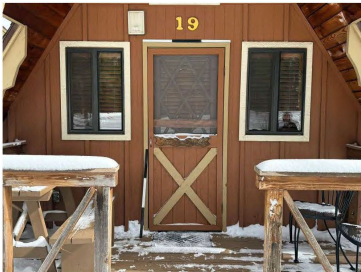
South wall, window and door details of Cabin Nineteen, view north, scale is 3 feet.
