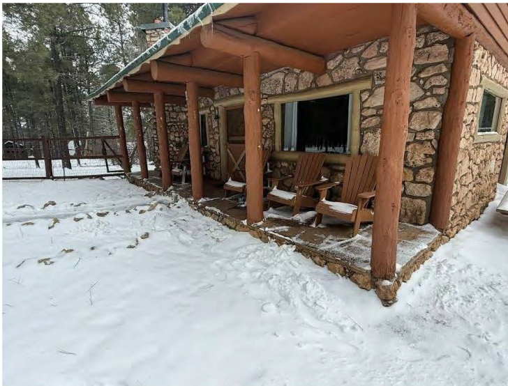
West wall and deck of Cabin One, view to the northeast.
