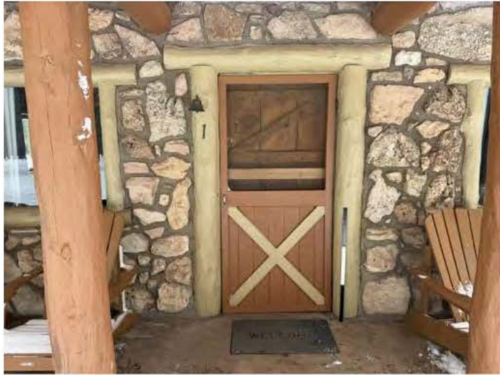
Front door, scale is 3 feet.
