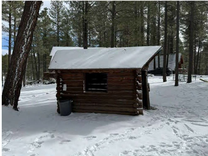
West wall and window of Small Cabin, view east.
