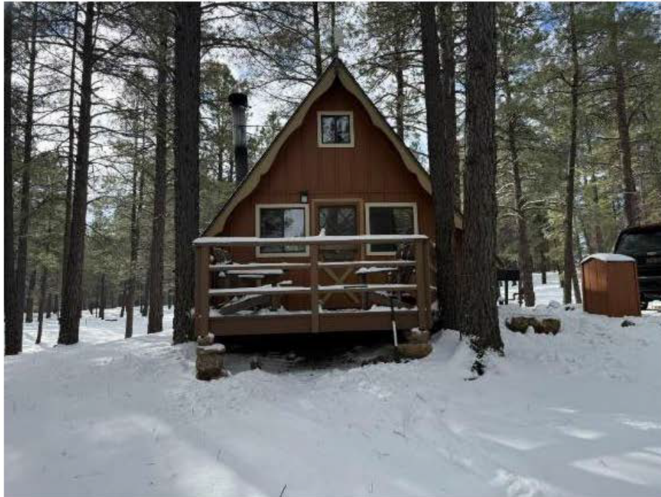
Figure 5-9. Cabin Seven (View to the South)
