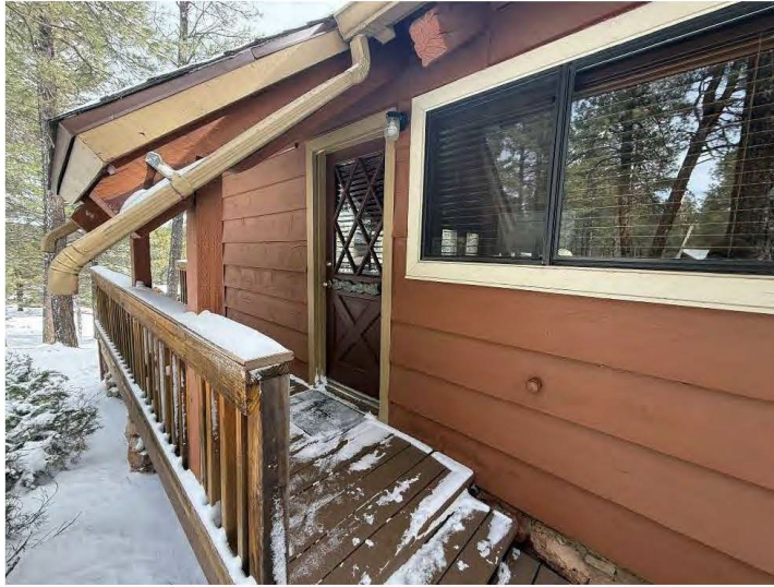
West wall entrance and landing of Cabin Sixteen, view northeast.
