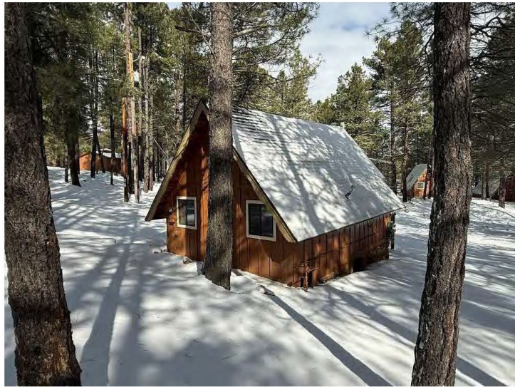
South and east walls of Cabin Ten, view northwest.
