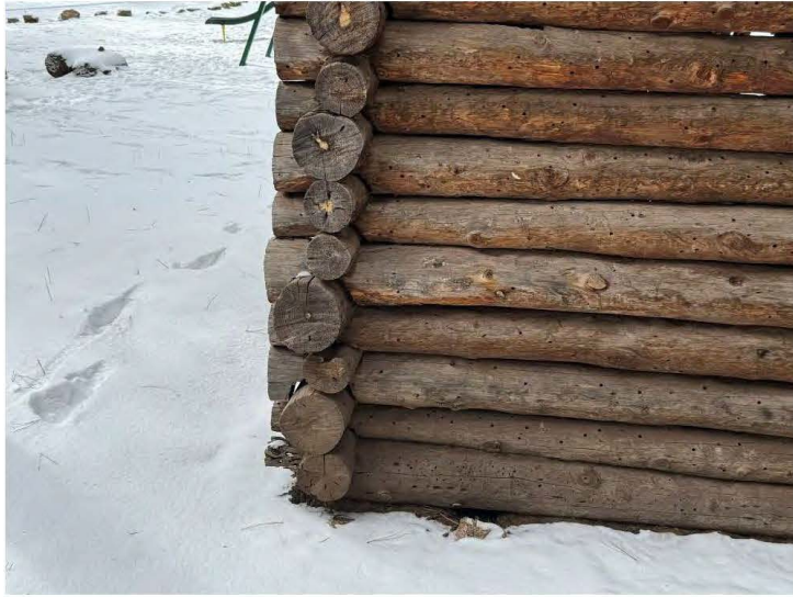
Northeast cabin corner details of Small Cabin, view south.
