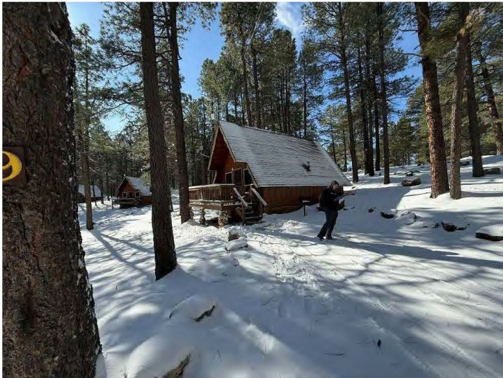
North and west walls of Cabin Nine, view southeast.
