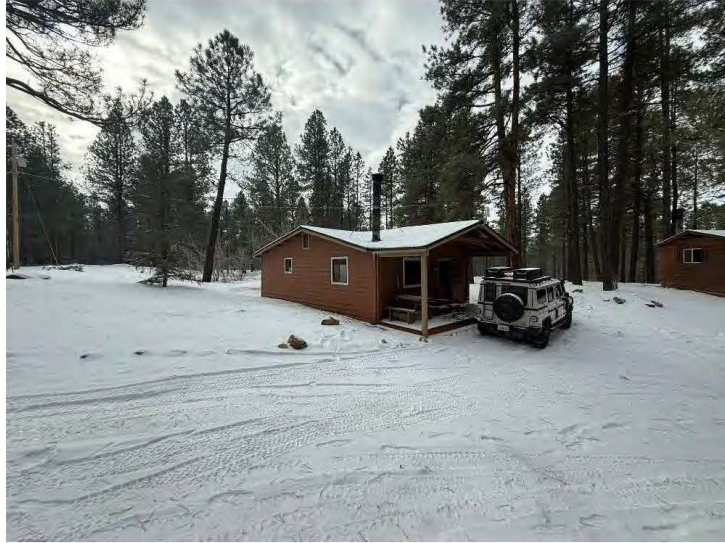
Overview of Cabin Five, view southeast.
