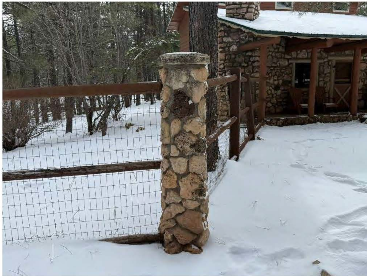
Example of fenced yard pillar made of local limestone at Cabin One, view to the southeast.
