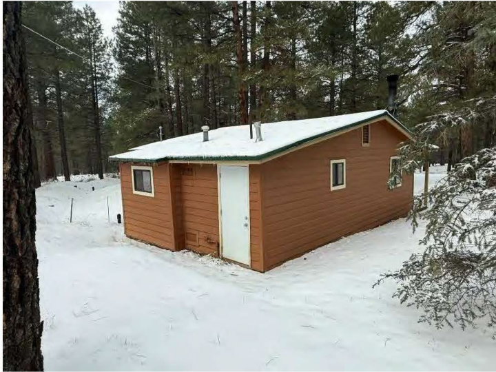
East and north walls of Cabin Five, view southwest.
