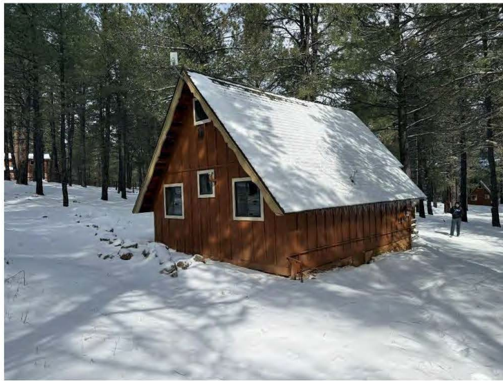
South and east walls of Cabin Eleven, view northwest.
