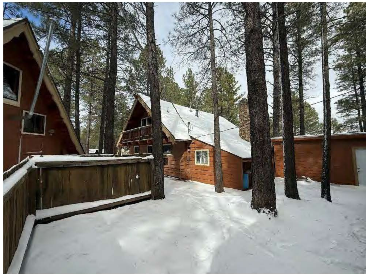
South and east walls of Cabin Sixteen, view northwest.
