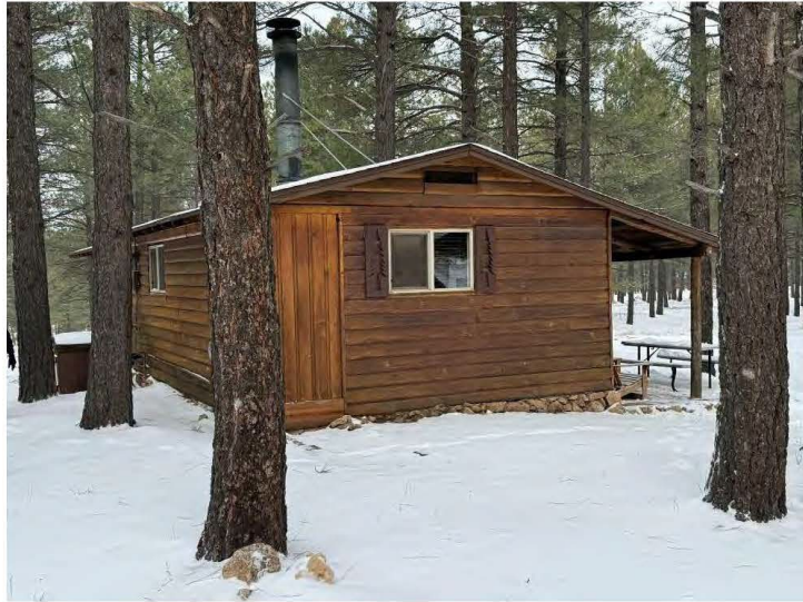
East wall and door of Cabin Two, view to the west-northwest.
