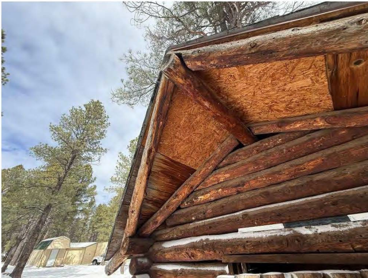
North wall roof details of Small Cabin, view northwest, scale is 3 feet.
