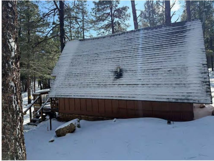
West wall of Cabin Nine, view east.
