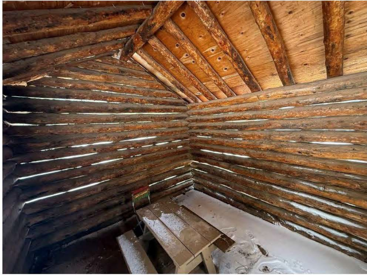
Interior details of Small Cabin, view northeast.
