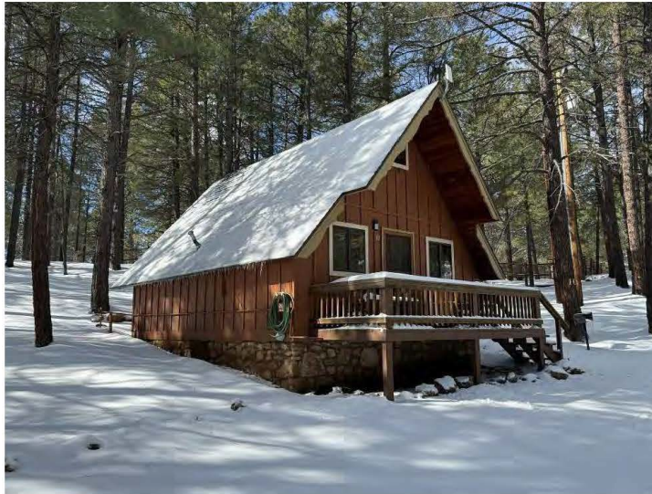
North and east walls of Cabin Ten, view southwest.
