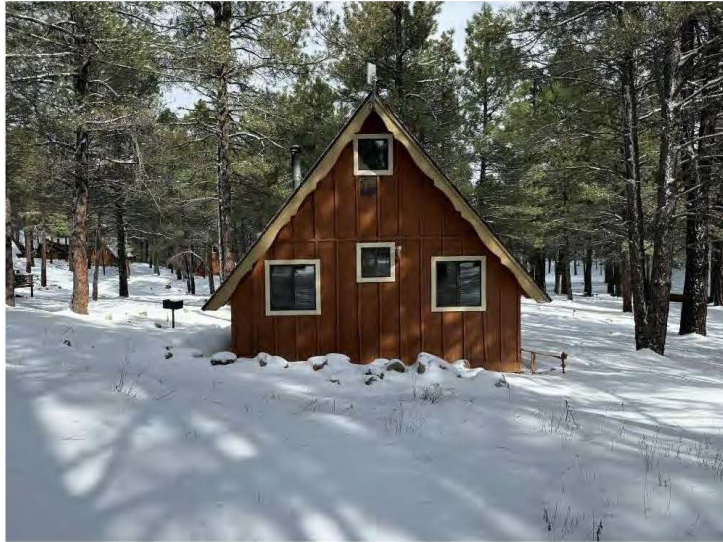
South wall of Cabin Eleven, view north.
