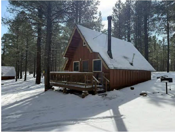
North and west walls of Cabin Eleven, view southeast.
