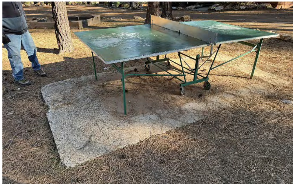
Figure 19 Concrete pad (IO17), view northeast.
