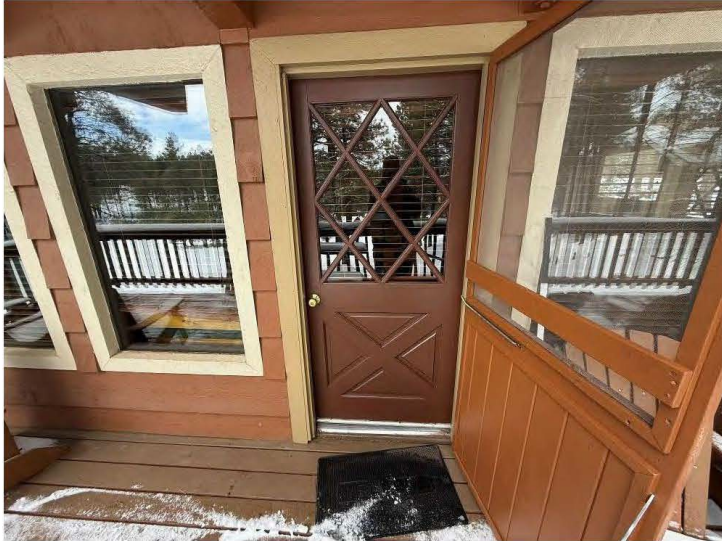
Door details of Cabin Sixteen, view south.
