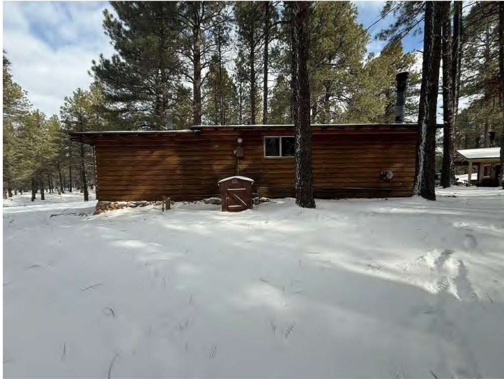
South wall of Cabin Two, view to the north.
