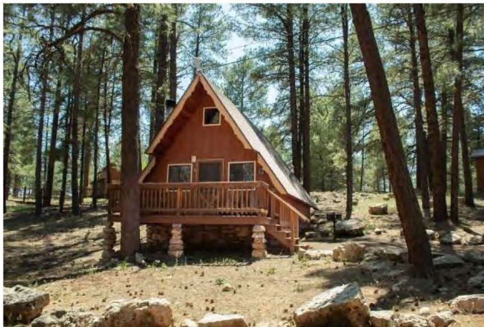
Cabin Nine exterior from website.
