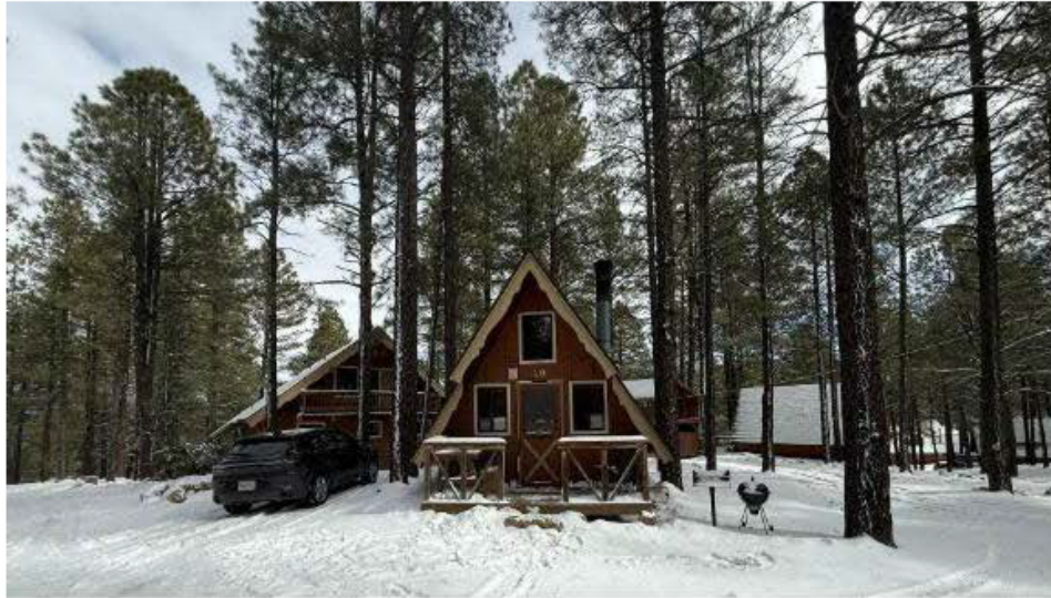
Figure 5-16. Cabin Nineteen (View to the South) (Cabin Sixteen Left Rear, Cabin Nineteen and Cabin Six Right Rear)
