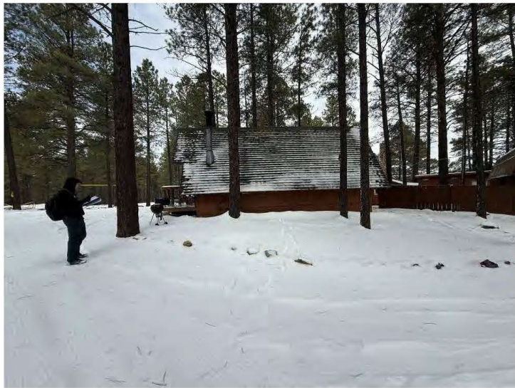
East wall of Cabin Nineteen, view west.
