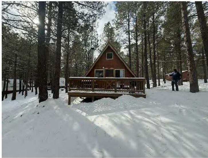
Overview and north wall of Cabin Six, view south.
