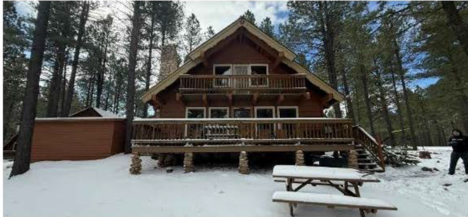
Figure 5-15. Cabin Sixteen (View to the South)
