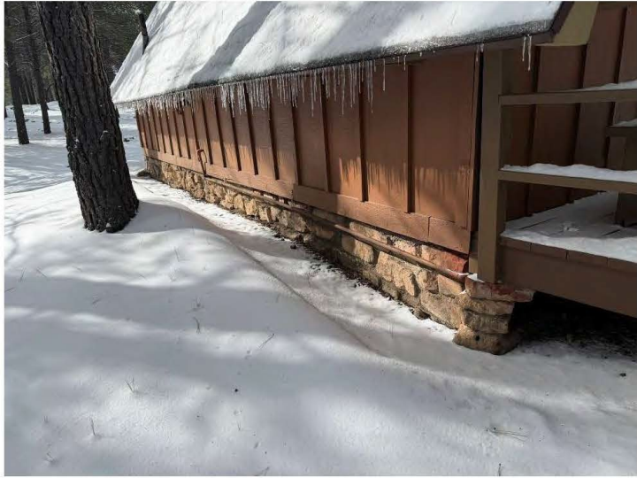
East wall and foundation at Cabin Seven, view southwest.
