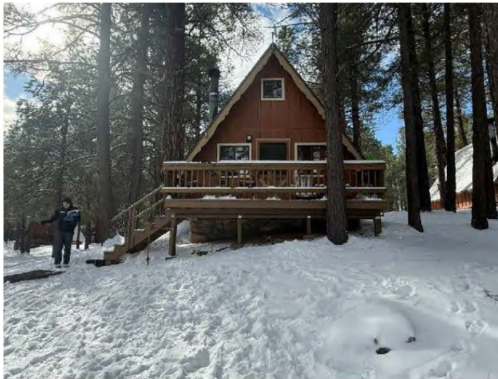
Overview and north wall of Cabin Eight, view south.
