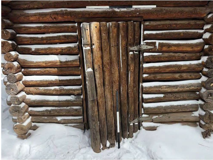
Door of Small Cabin, view north, scale is 3 feet.
