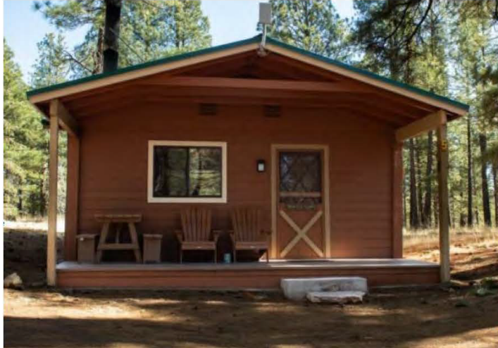
Cabin Five exterior from website.
