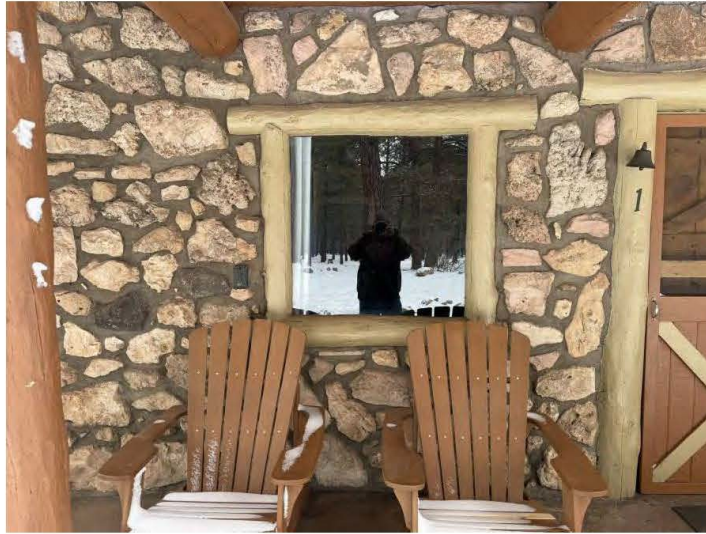
Window and stonework details.
