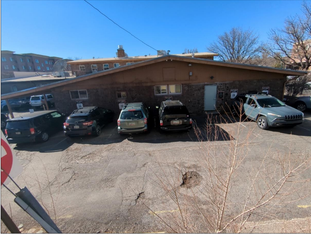
Photograph 7. East elevation of 19 West Birch Avenue, showing the east facade of the former police station.
