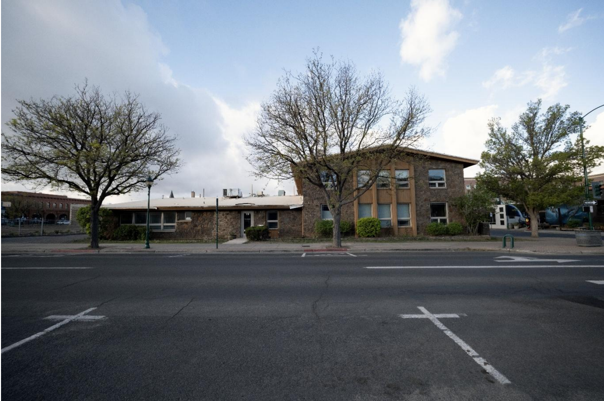
Photograph 17. North elevation of 19 W. Birch.
