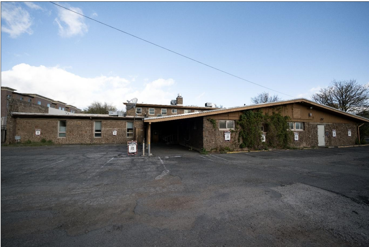
Photograph 16. East elevation of 19 W Birch.
