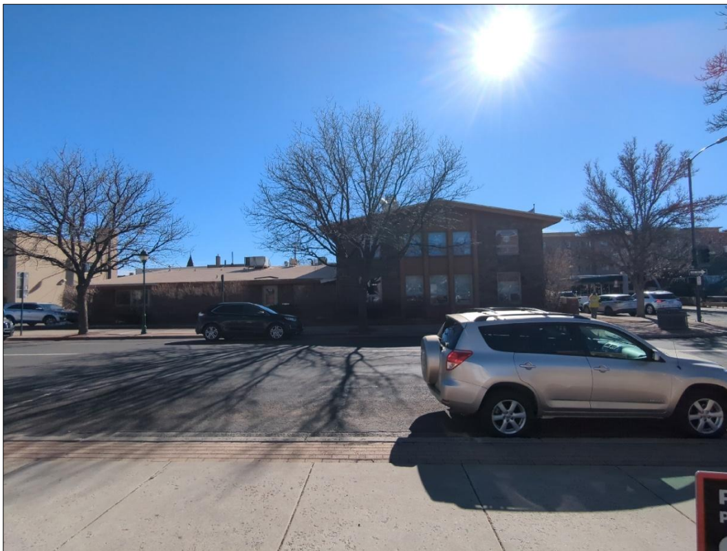
Photograph 4. North elevation of 19 West Birch Avenue, showing the north entryway into the building.
