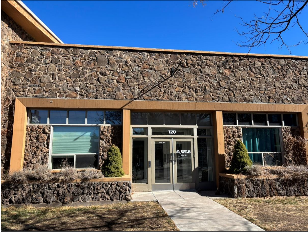
Photograph 5. East facing photograph showing the entryway to southern portion of the building which once housed the fire department.
