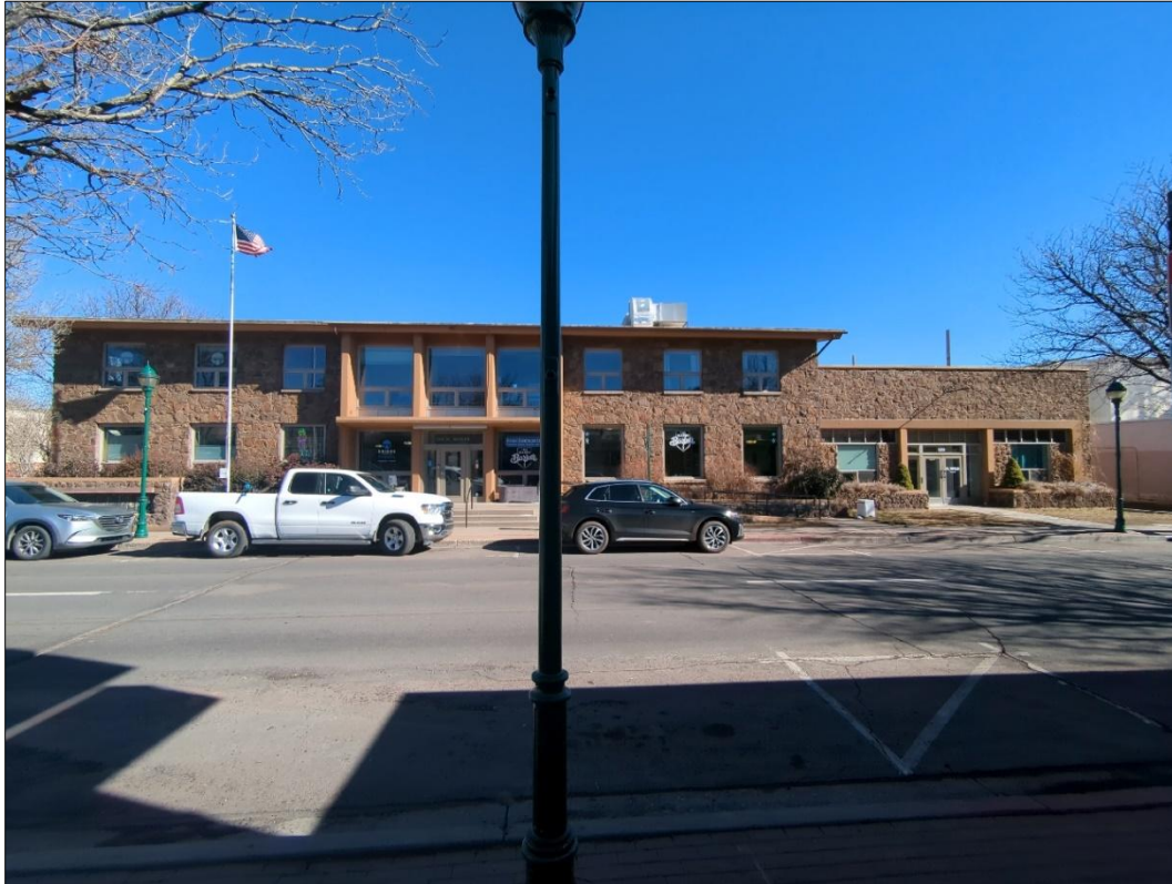
Photograph 3. West elevation of the studied building at 19 West Birch Avenue, the City Hall and Fire Department portions of the building are visible.
