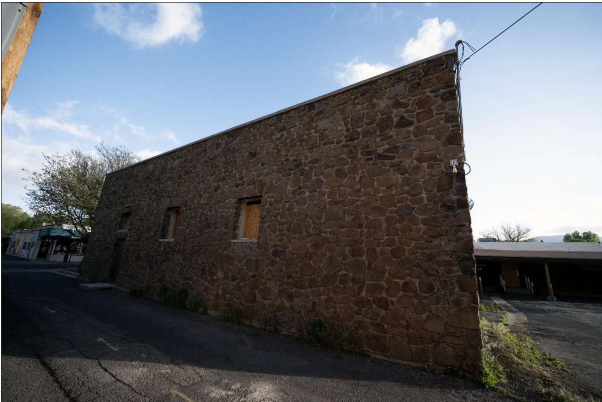
Photograph 18. South elevation of 19 W. Birch.
