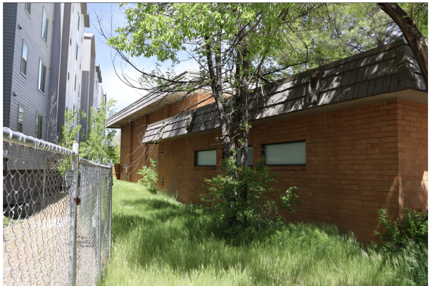
View along west property line looking North
