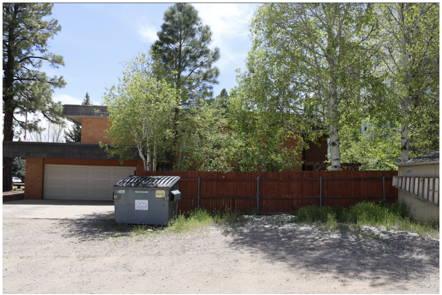
North elevation from North property line
