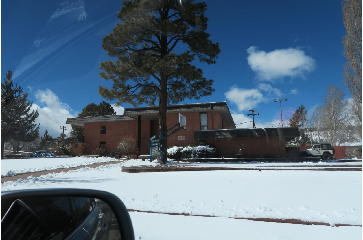
East elevation, looking west
