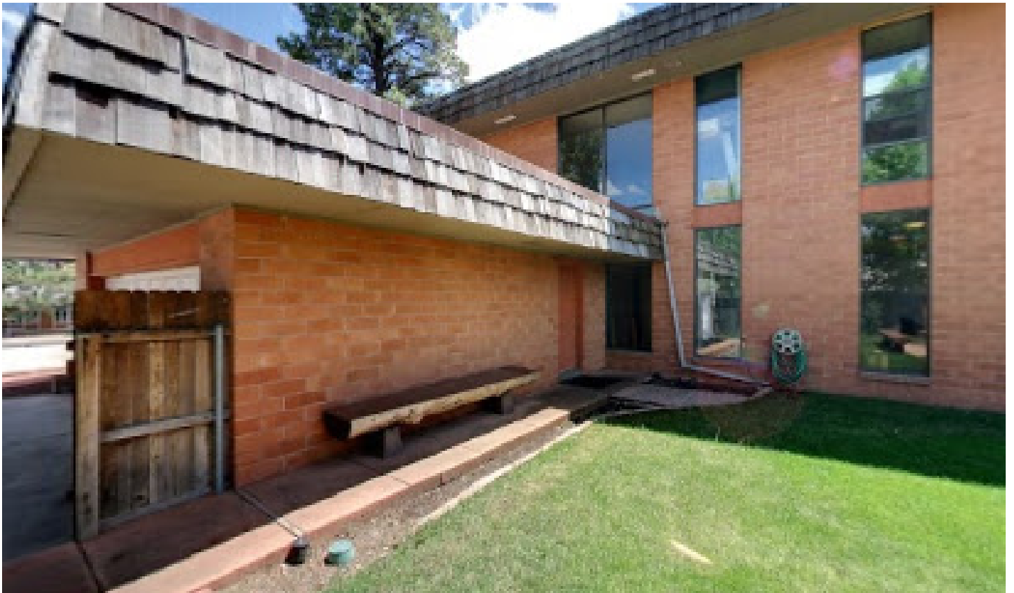
View from north, looking south
