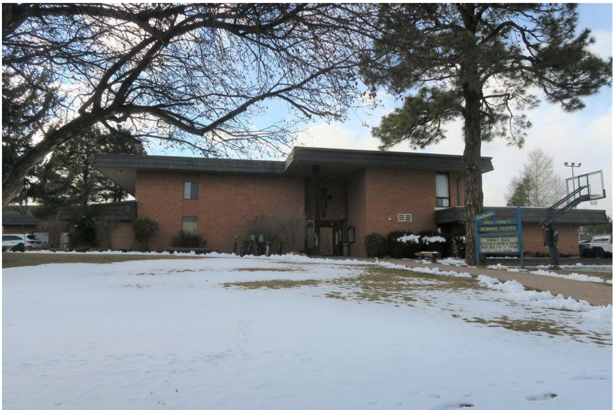
Photo 1. Main façade of Newman Center looking northwest
