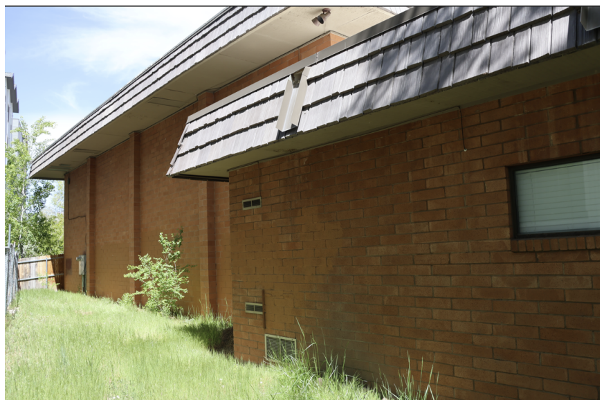
View along west property line looking North
