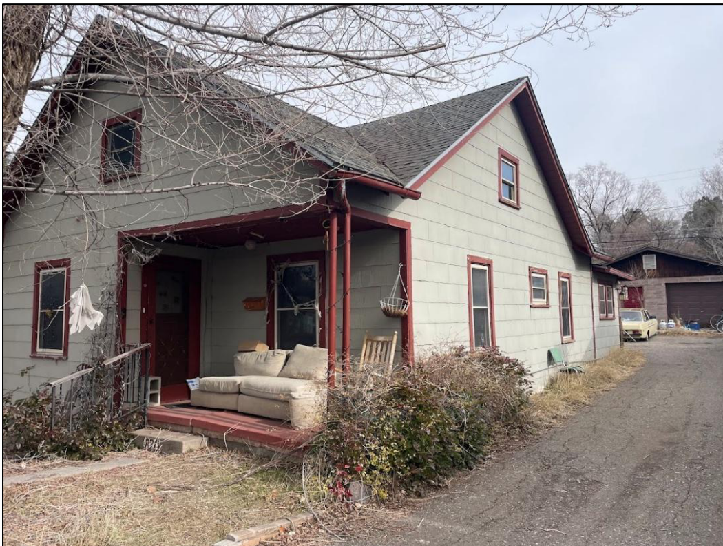
Photograph 7. South elevation showing differential settlement
