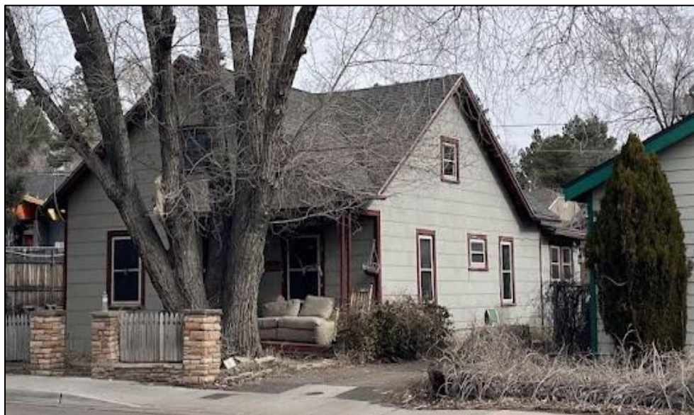
Photograph 4. West Elevation from Beaver Street
