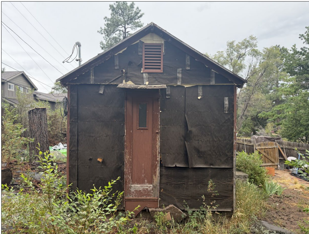
Photograph 8. Overview of the northern elevation at 804 ½ North LeRoux Street, facing south.
