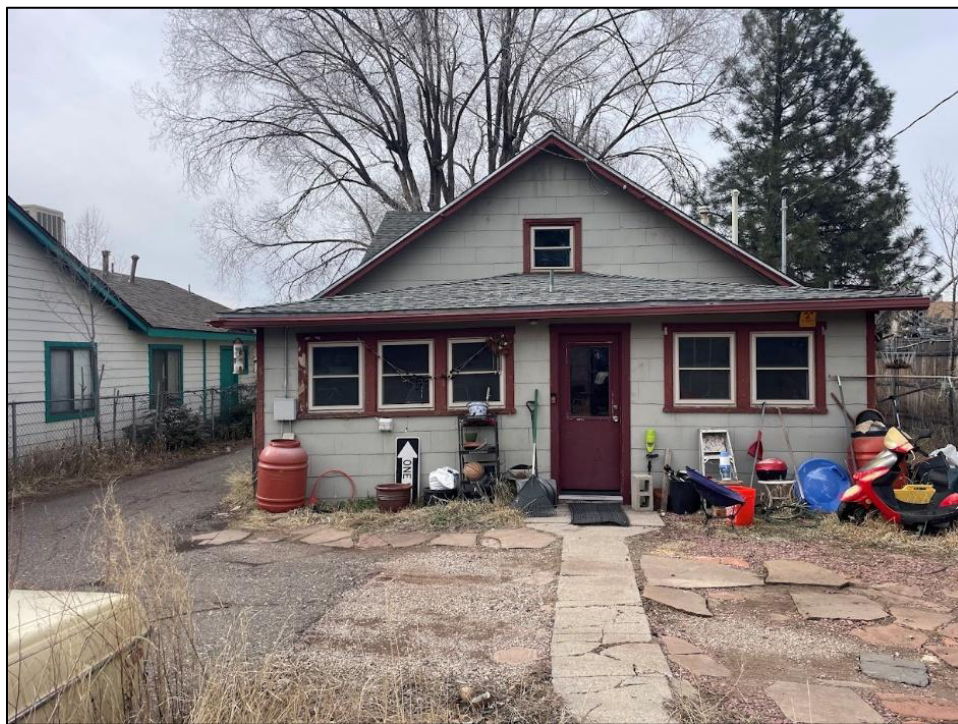
Photograph 6. East elevation showing later addition
