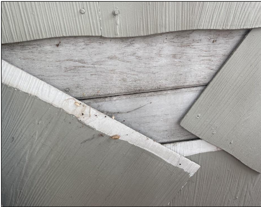
Photograph 5. Original siding beneath the asbestos siding
