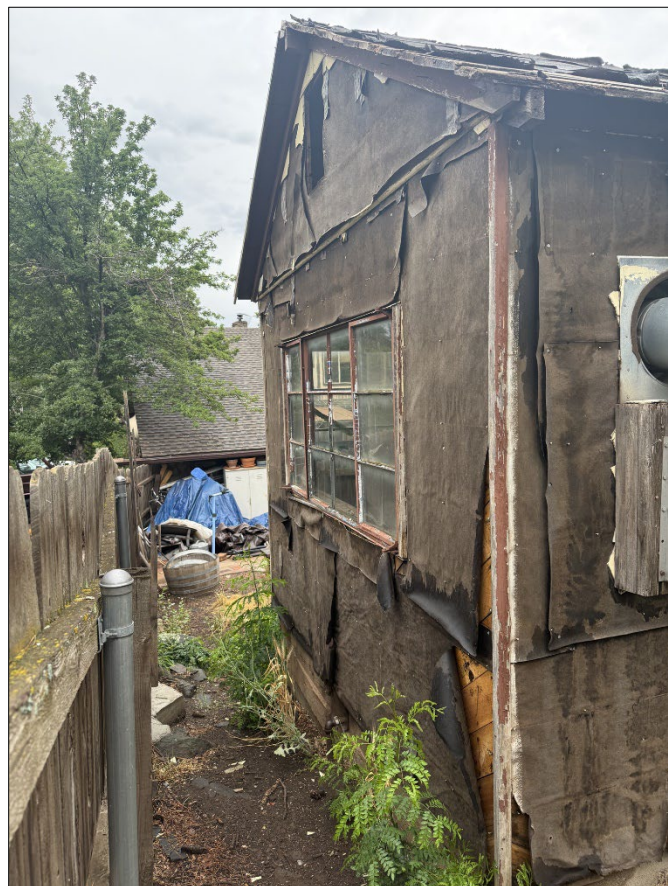
Photograph 2. Overview of the southern elevation at 804 ½ North LeRoux Street, facing northwest.
