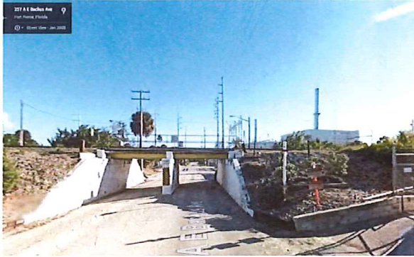
Figure 1: Avenue C Bridge
