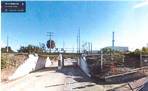
Figure 1: Avenue C Bridge
