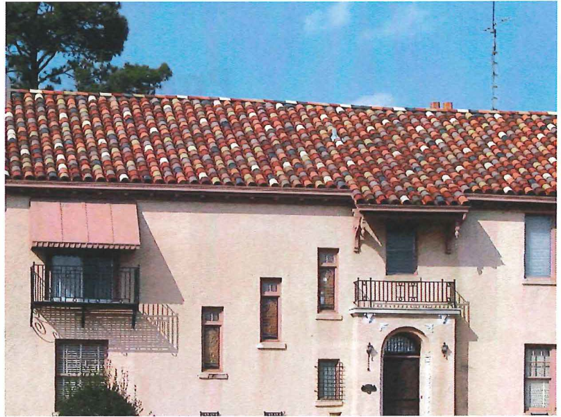
14-1/4" Straight Barrel Mission™ tile in a 7 color blend
