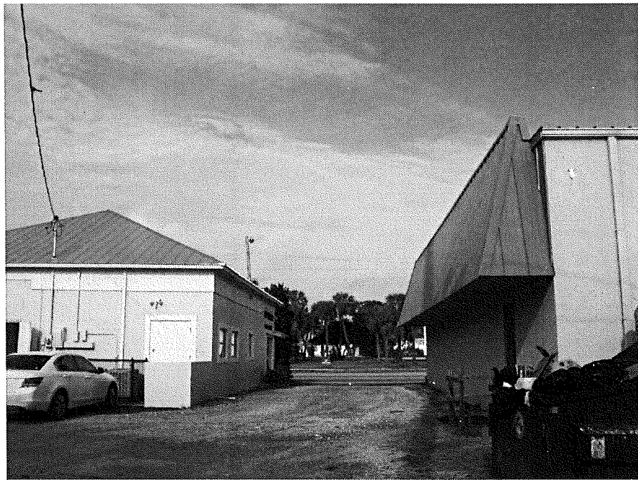
West view along alley connecting to the subject, lying south of adjacent 810 S. US 1
