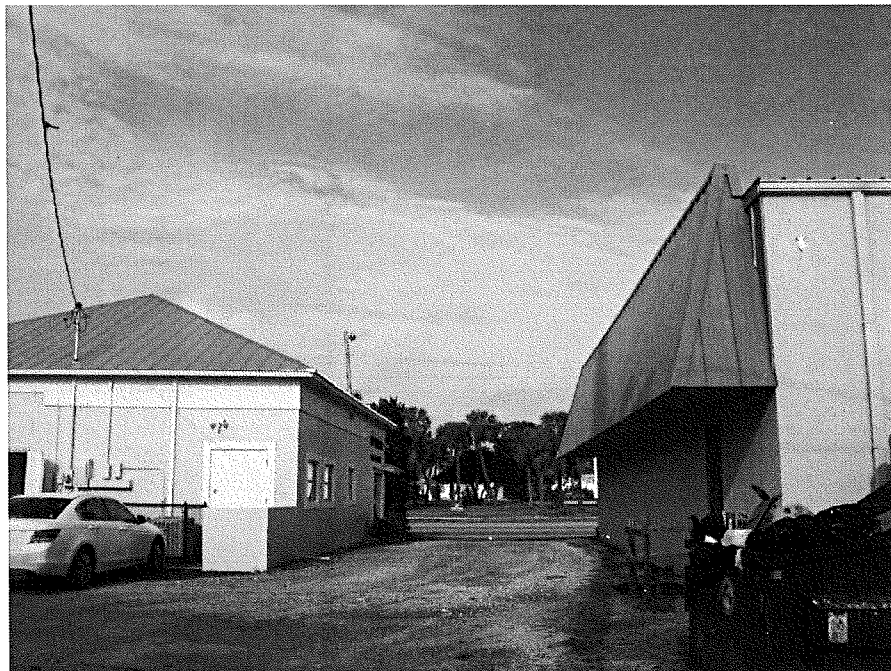
West view along alley connecting to the subject, lying south of adjacent 810 S. US 1
