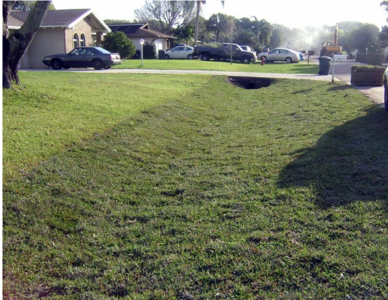
Egret Ave. – Swales Re-graded
