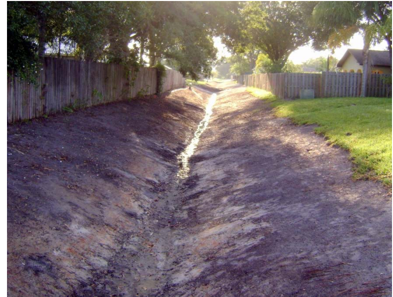
Back Lot Drainage Swales Re-graded
