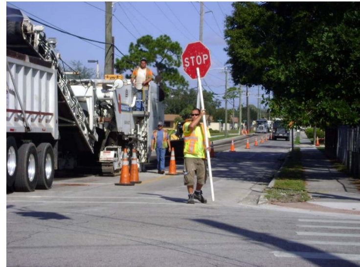
29 th Street Paving
