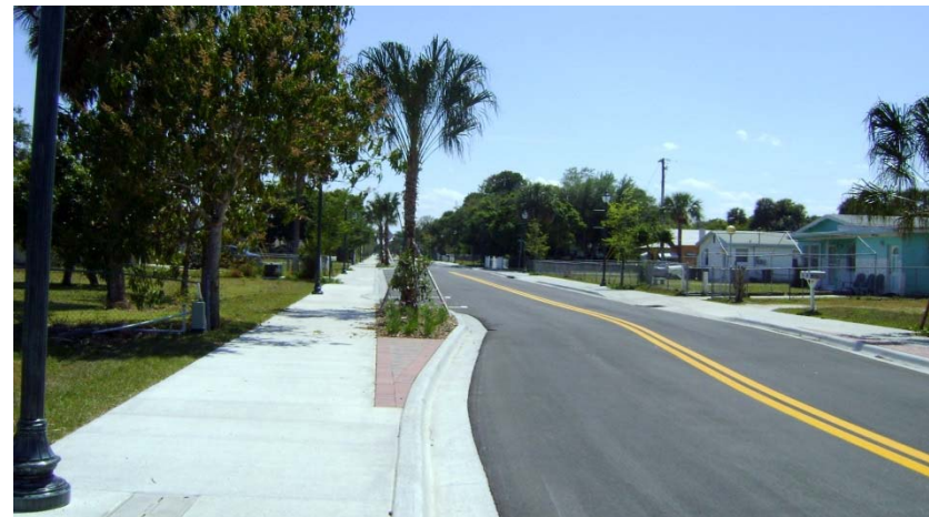
10 th Street Reconstruction
