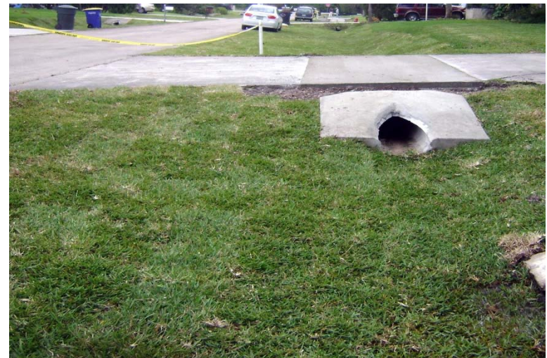
Driveway Culvert Replacement
