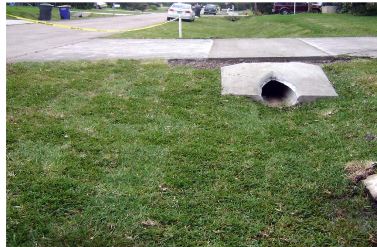
Driveway Culvert Replacement
