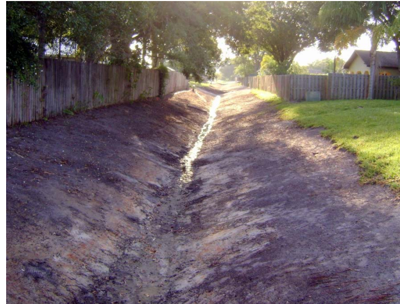
Back Lot Drainage Swales Re-graded
