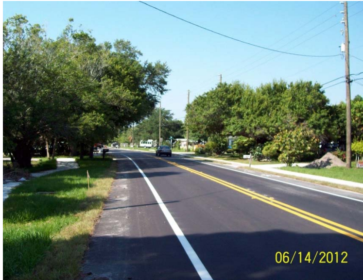
Sunrise Blvd. Completed Project
