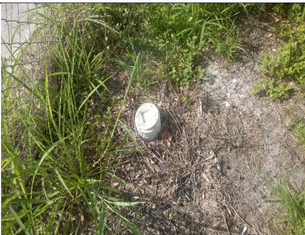
Photo 6: View of clean-out located in east side of site.
