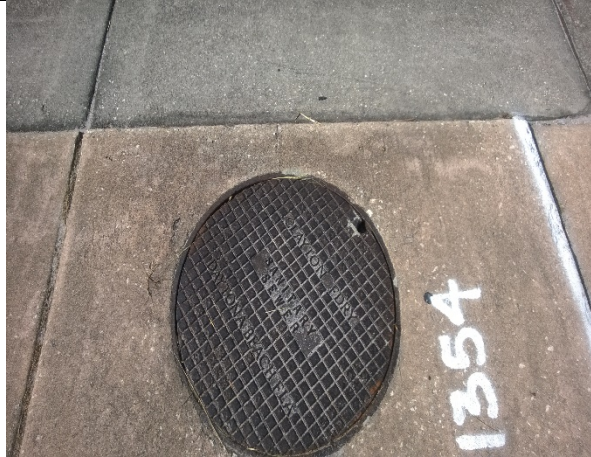
Photo 13: View of sanitary sewer manhole located in south side of site.
