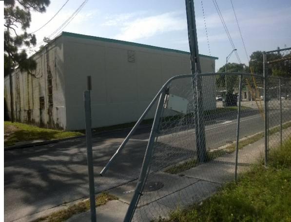
Photo 8: View of N 17 th Street and east adjoining property beyond.
