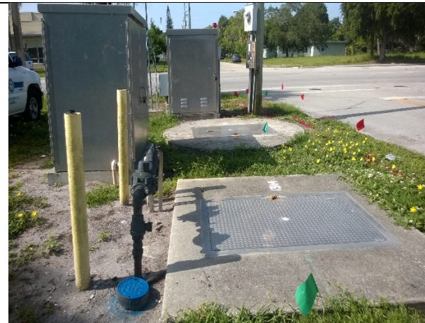
Photo 16: View of lift station located in southwest corner of site.
