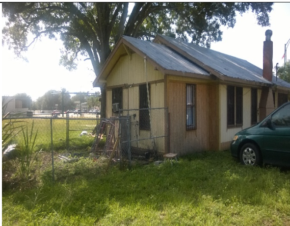
Photo 17: View of residence.
