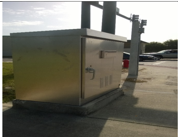
Photo 12: View of traffic signal control box located in southeast corner of site.
