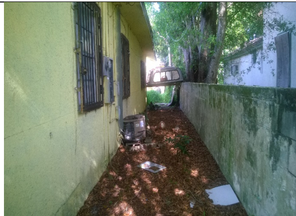
Photo 4: View between residence and north adjoining property.
