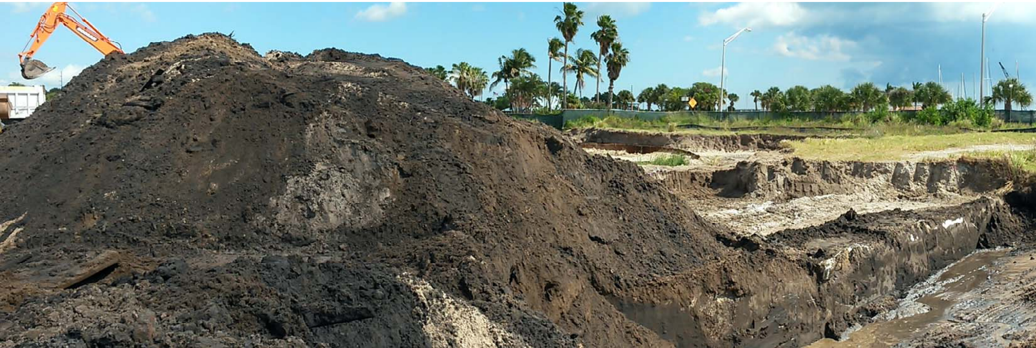
King Plant Property - Contaminated soil removal - April 9, 2014
