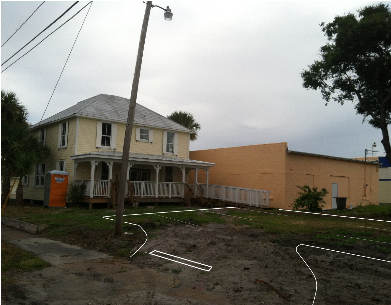
Rear Yard— Prior to Parking Lot Construction
