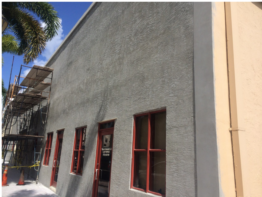
Current Progress of Stucco Repair/Replacement on Southern Façade
