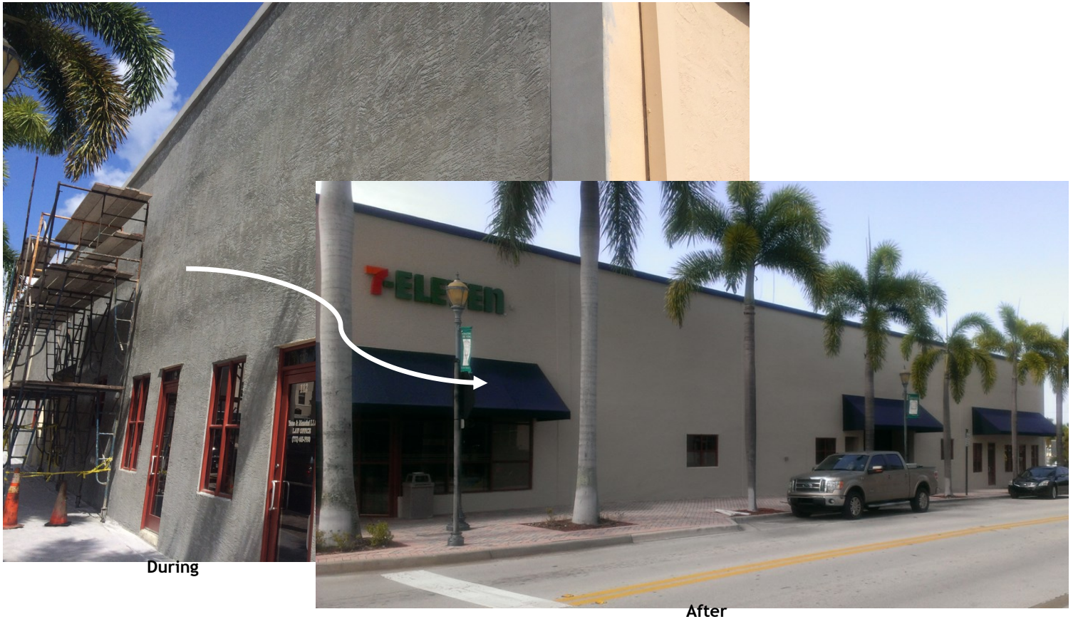
Recent Stucco Repair/Replacement on Southern Façade - Now Completed
