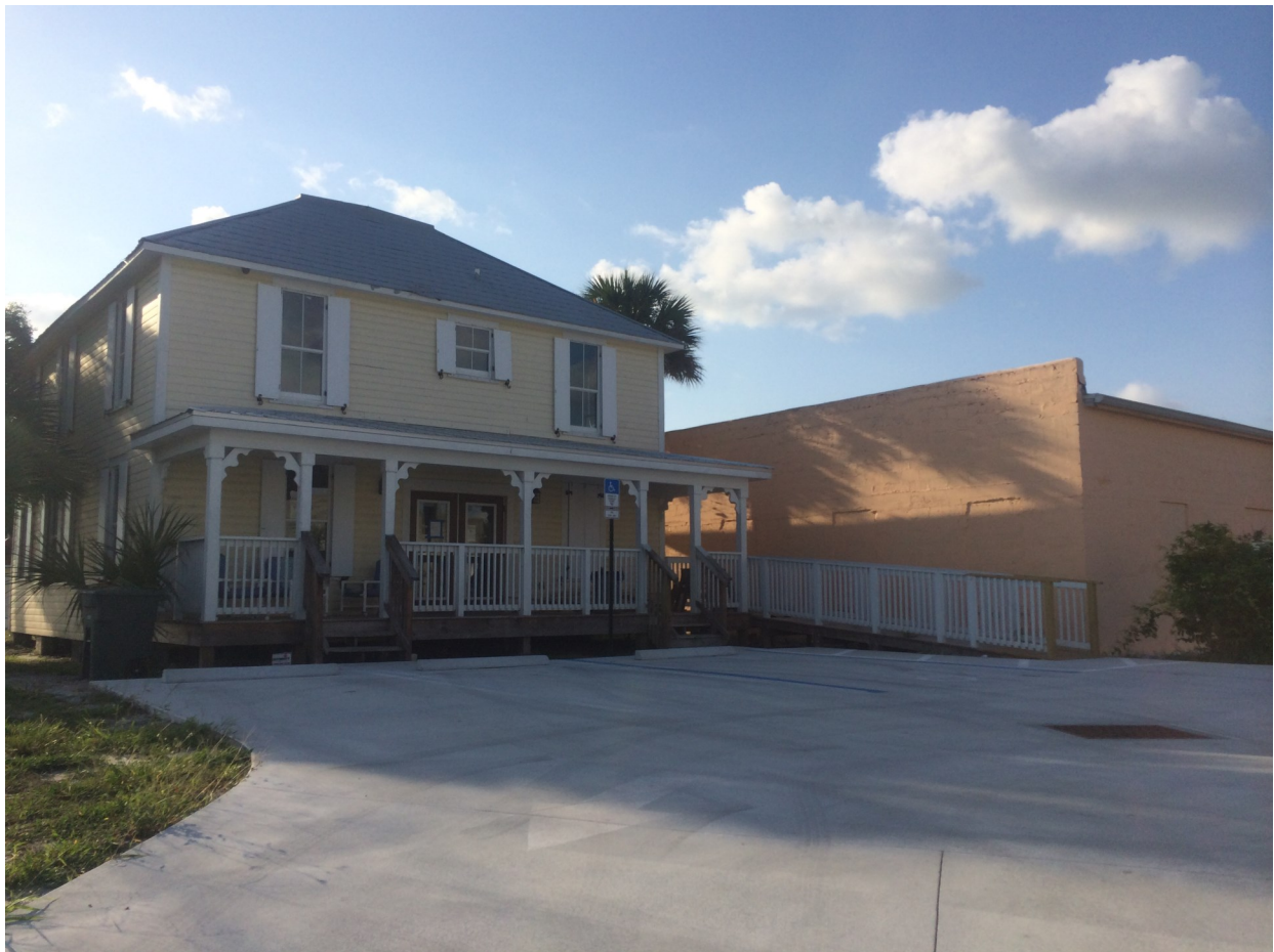
Rear Yard after Parking Lot Construction
