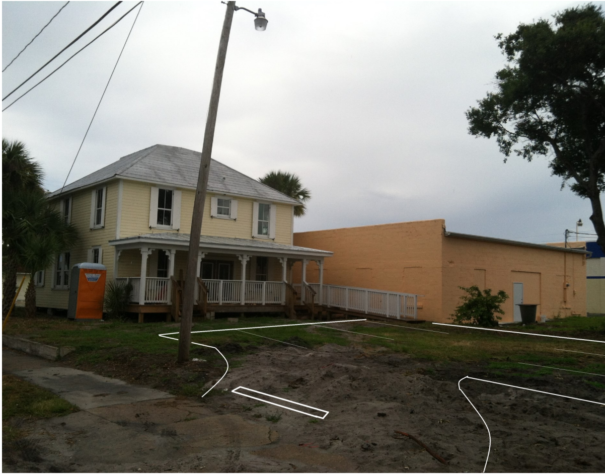
Rear Yard prior to Parking Lot Construction
