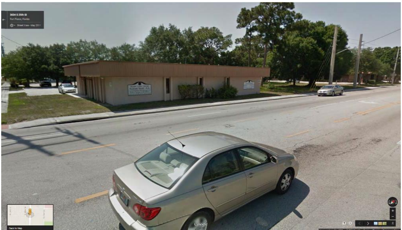
Existing business along South 25th Street which integrates a continuous flat parapet which conceals a low sloping roof as well as any roof top mounted equipment.
