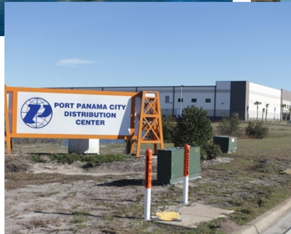
Port Panama City Intermodal Distribution Center
