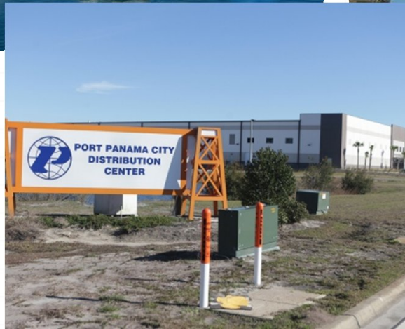
Port Panama City Intermodal Distribution Center
