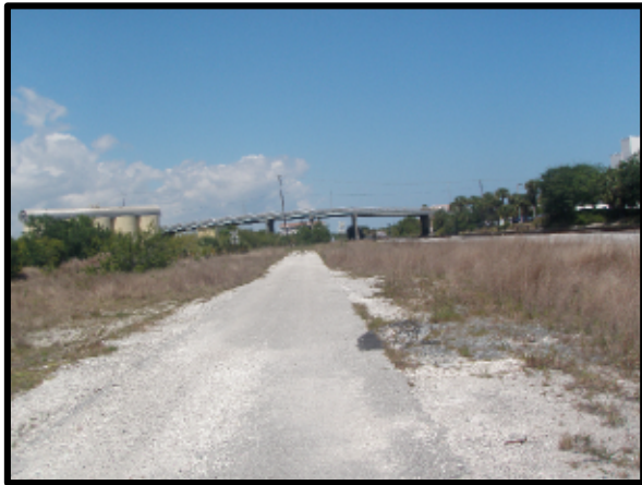
PHOTOGRAPH #01: AT ROAD ALONG EASTERN SITE BOUNDARY, LOOKING NORTHWEST TOWARD CITRUS AVE.
