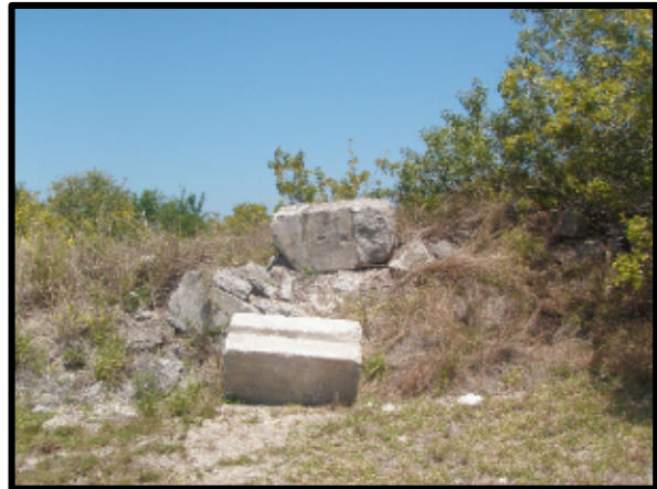
PHOTOGRAPH #04: CONCRETE RUBBLE LEFT ON-SITE
