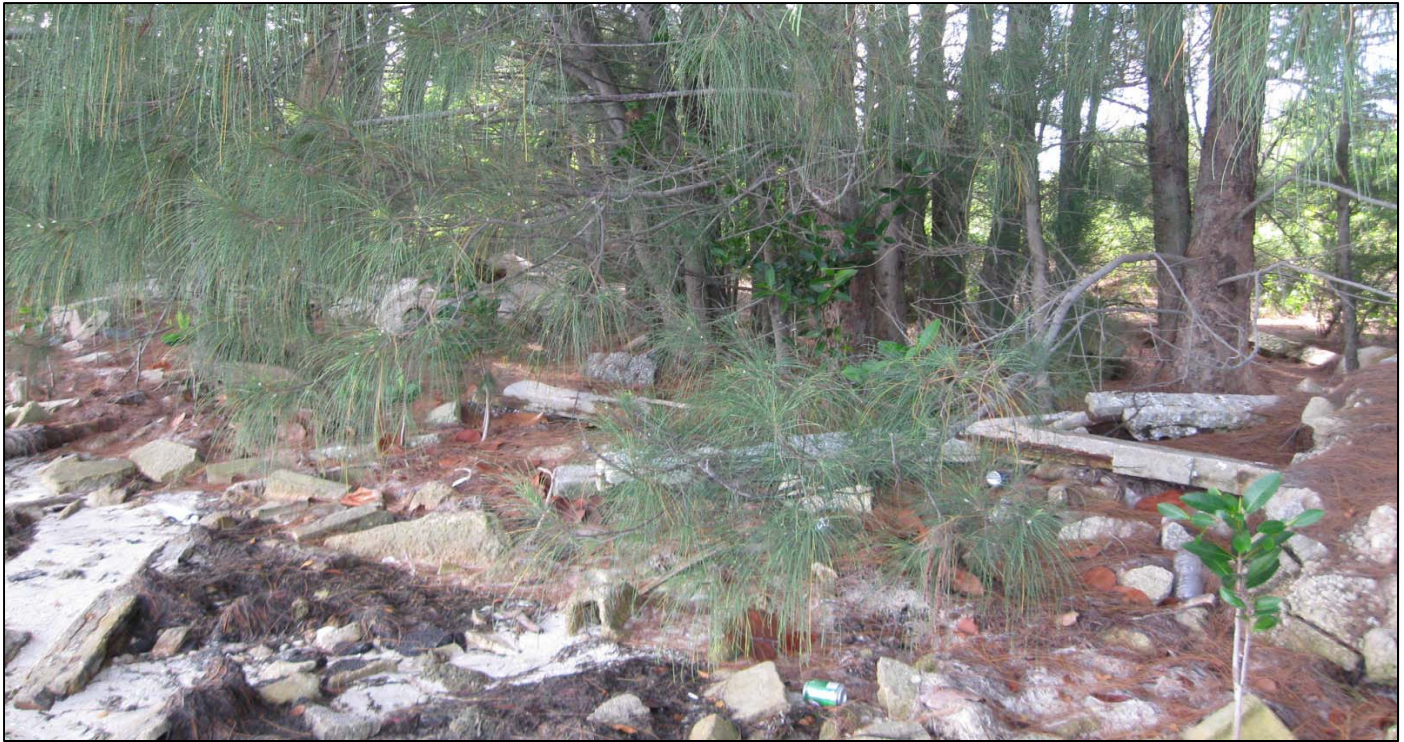
Photo looking at concrete rubble in shoreline area.
