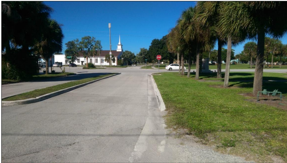
VIEW LOOKING WEST ALONG HAYES STREET
