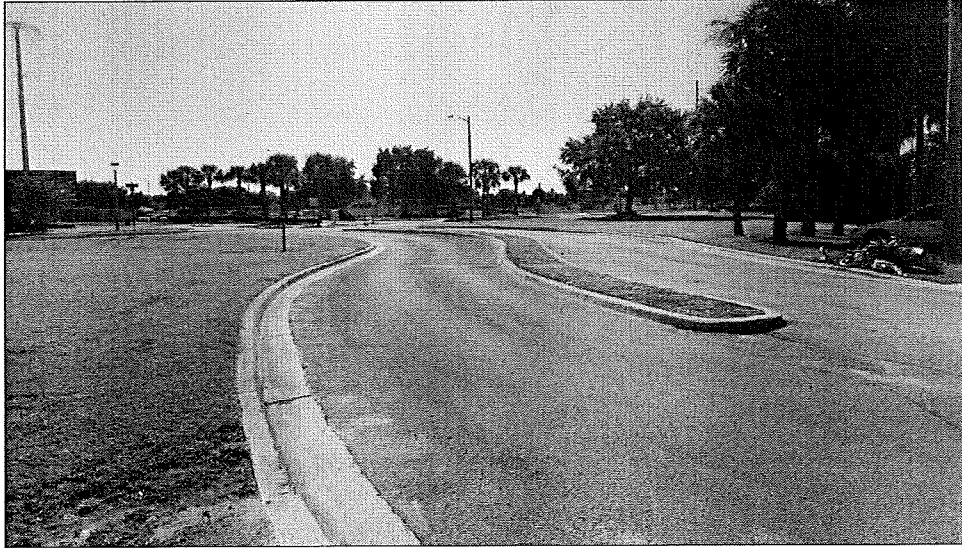
VIEW LOOKING EAST ALONG HAYES STREET
