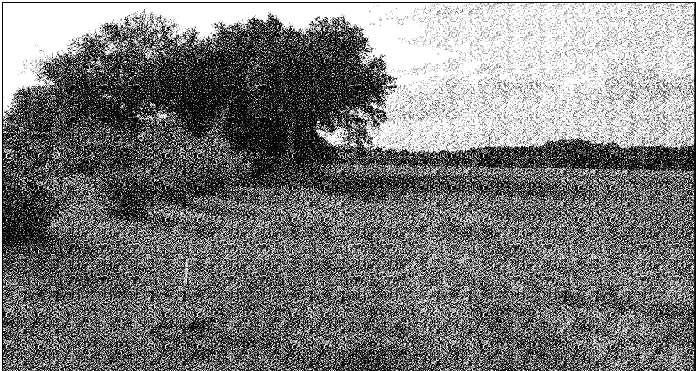
Photo looking west along a portion of the south property line showing vegetative encroachment.
