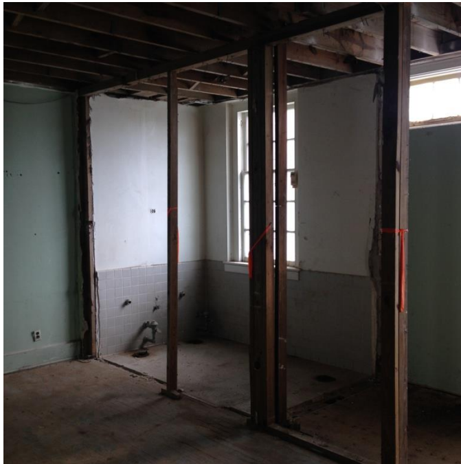
Ground floor underneath the rear loft
