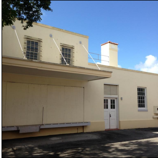
Rear view from loading dock area
