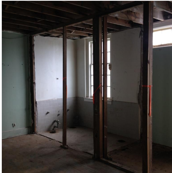
Ground floor underneath the rear loft
