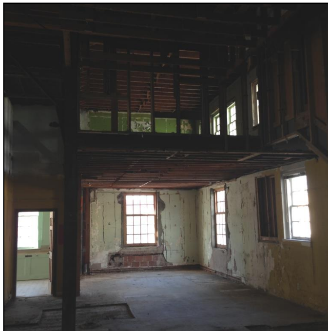
Front loft area
