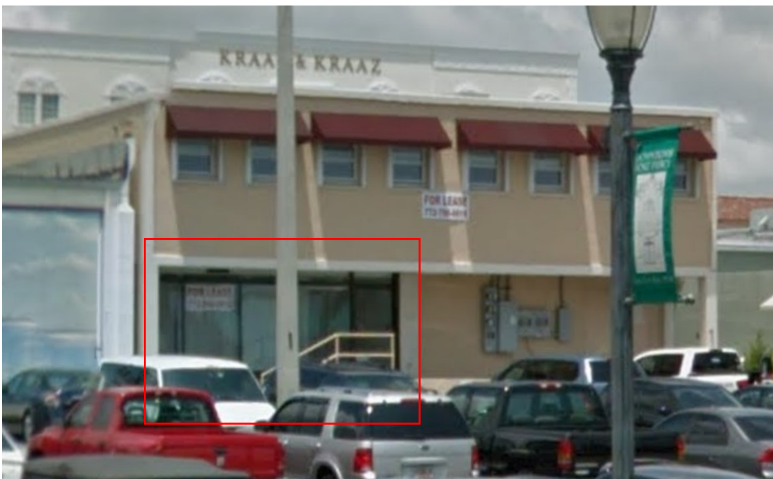
Existing – Rear Façade
