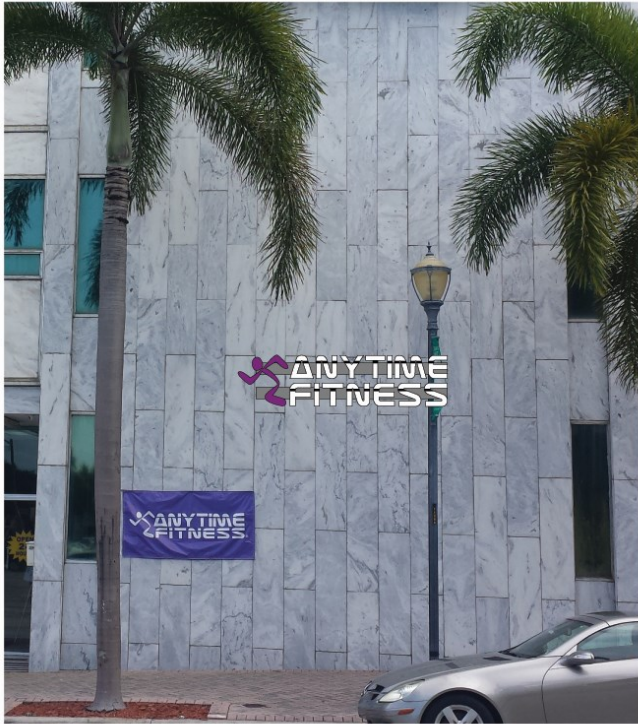
x1 Sign Installed per side of building
