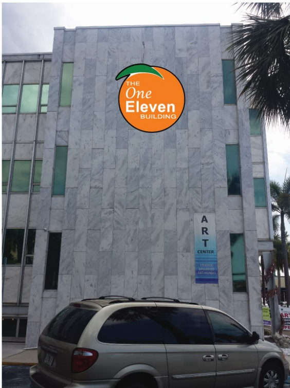
xl Sign Installed per side of building
