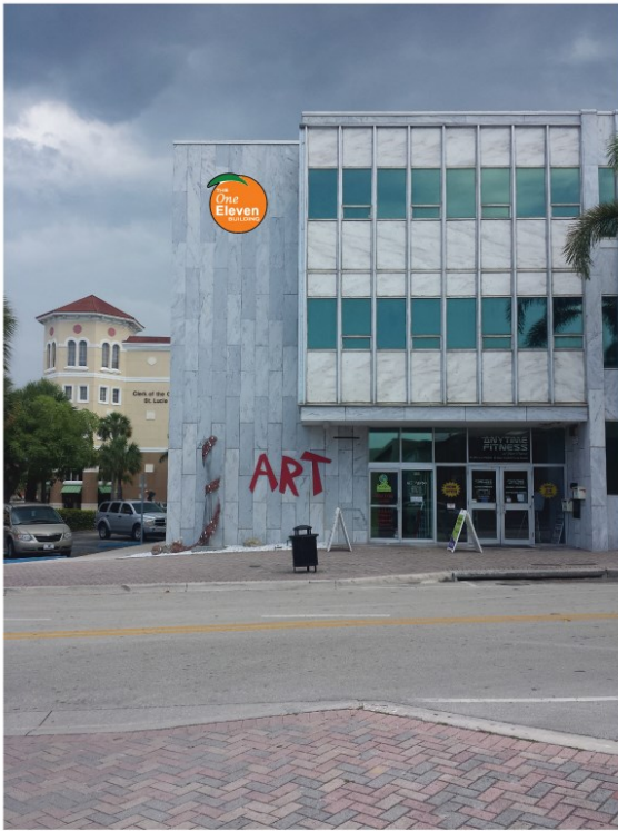
xl Sign Installed per side of building
