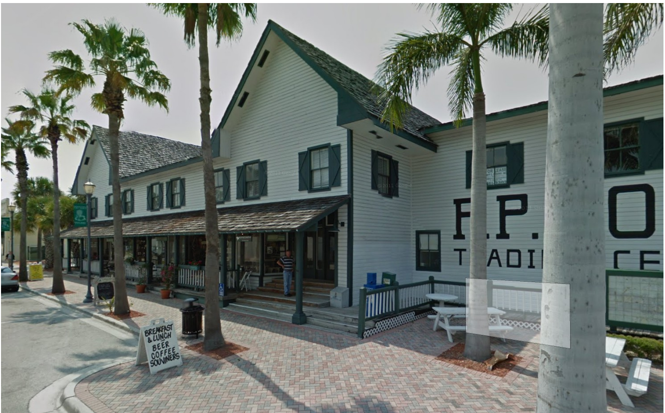
Photo of the PP Cobb Building, noting the absence of signs for upper story commercial businesses.
