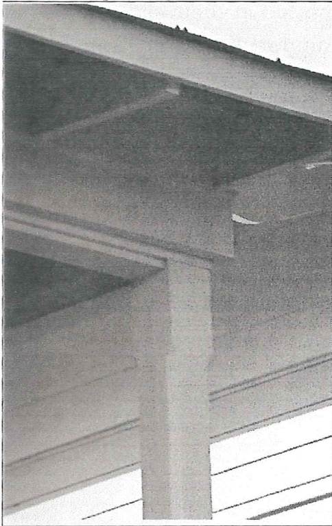
Board beam over chamfered wood column
