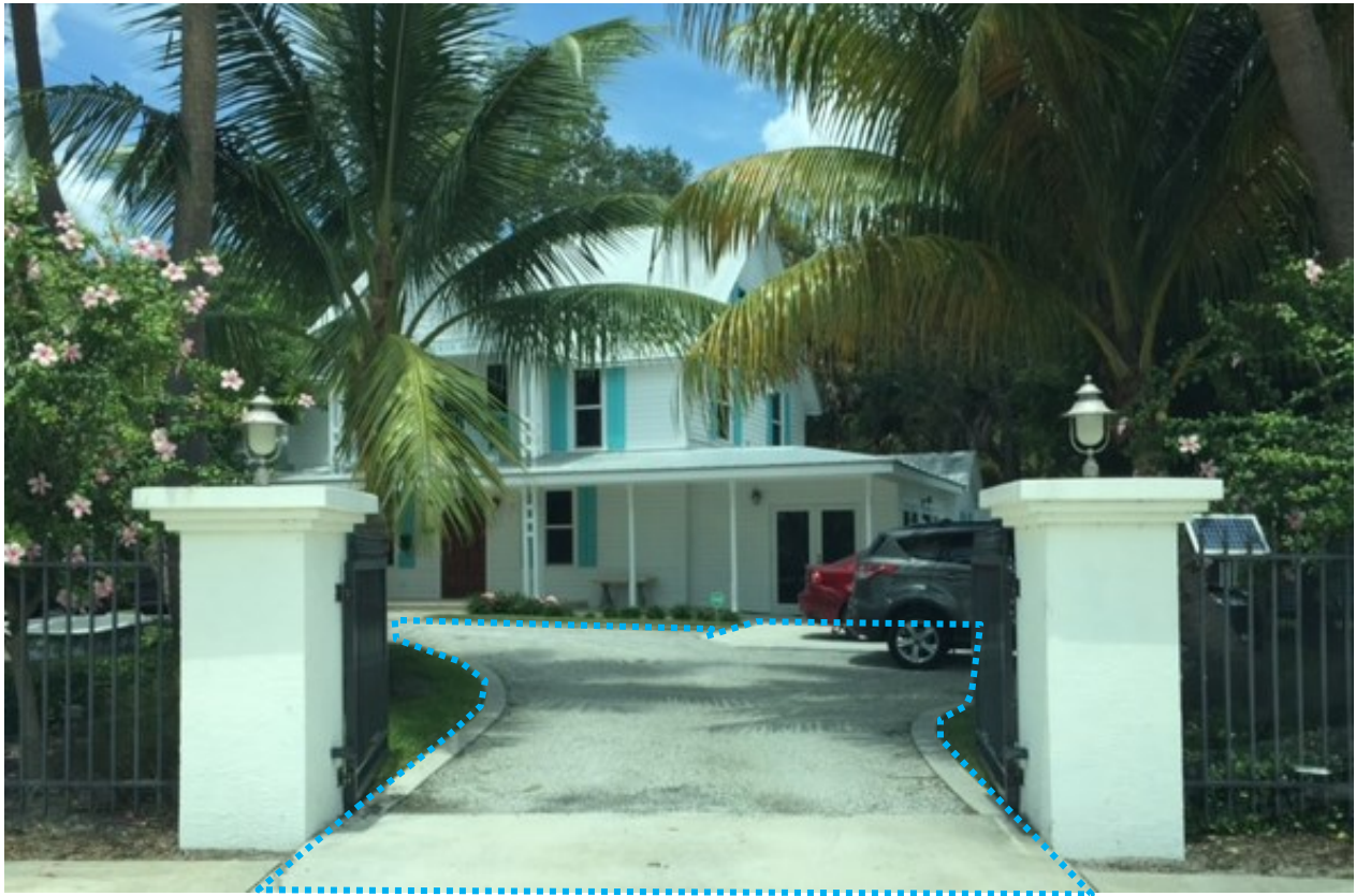
Existing example of cut cap rock and stone, on a coquina base, paving system
