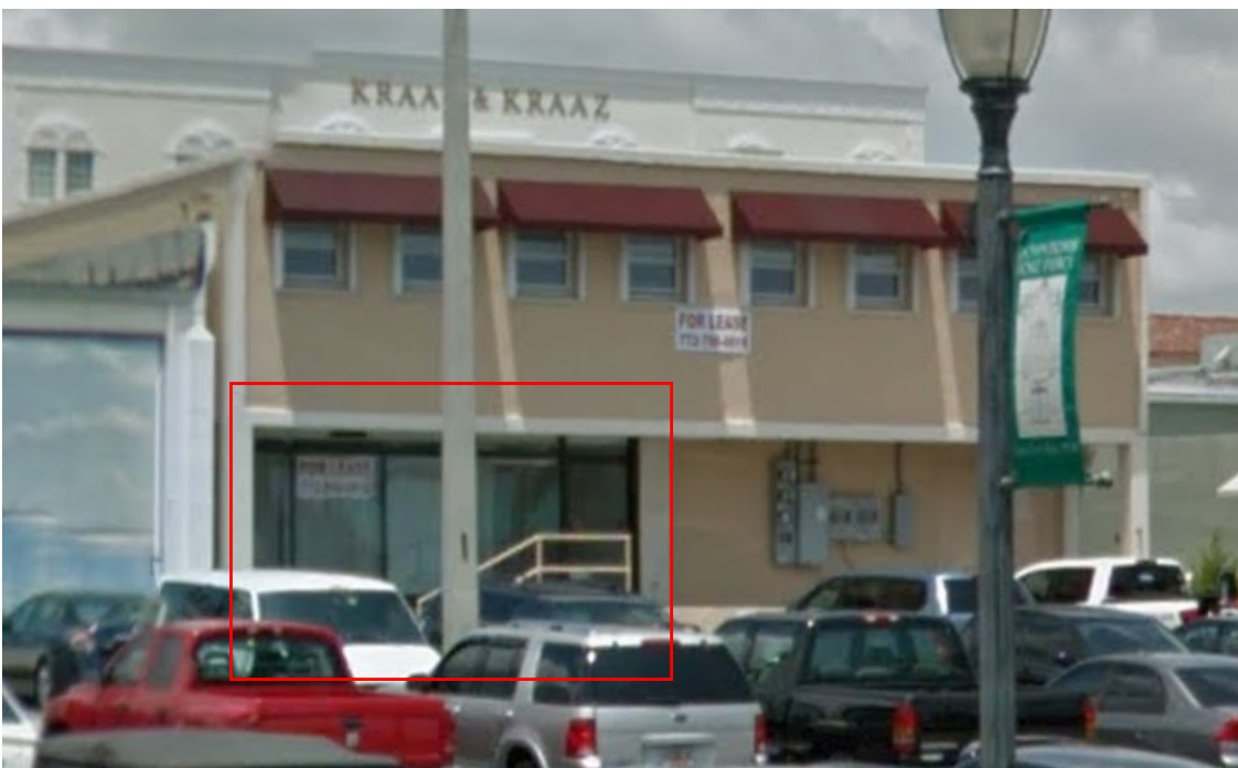
Existing – Rear Façade
