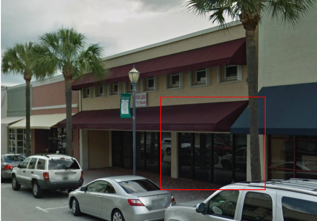
Existing – Front Façade
