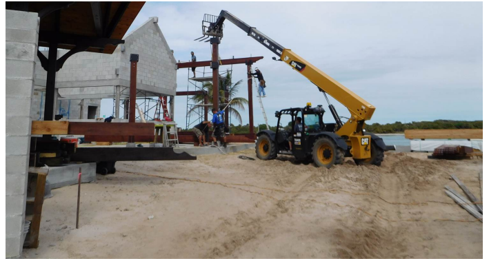
Installing a support for the outdoor tiki bar
