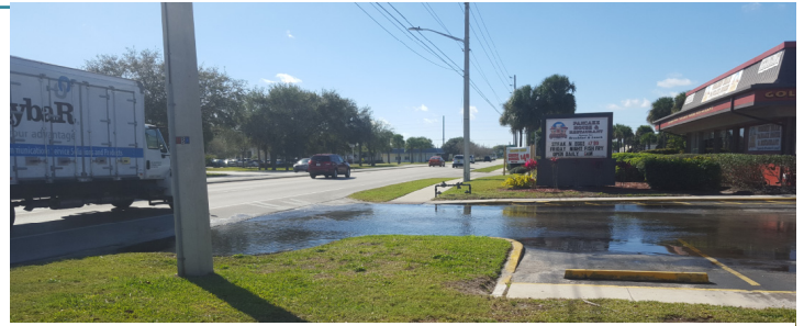
Flooding issue - post storm event
