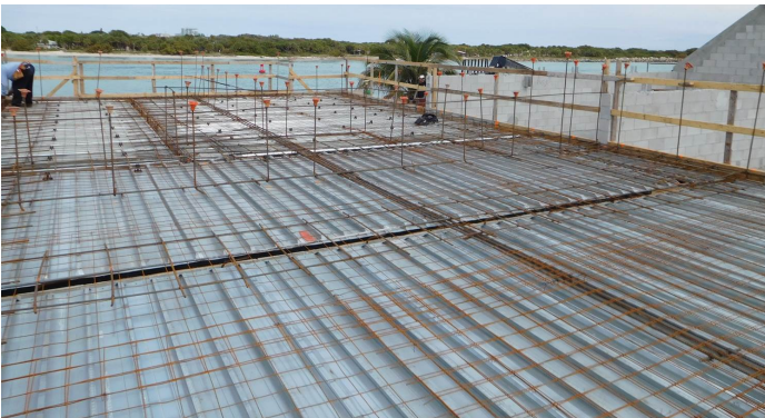
Second floor deck ready for inspection
