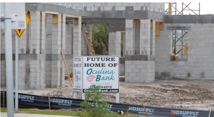
Oculina Bank construction progress 2/29/16
