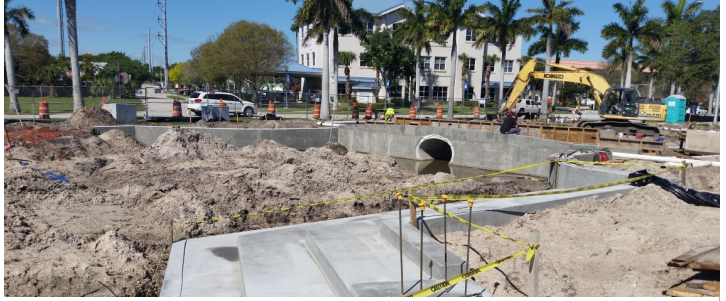
Pedestrian bridge and terrace seating
