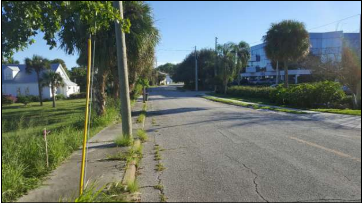
STREET SCENE ALONG SOUTH 2 ND STREET
