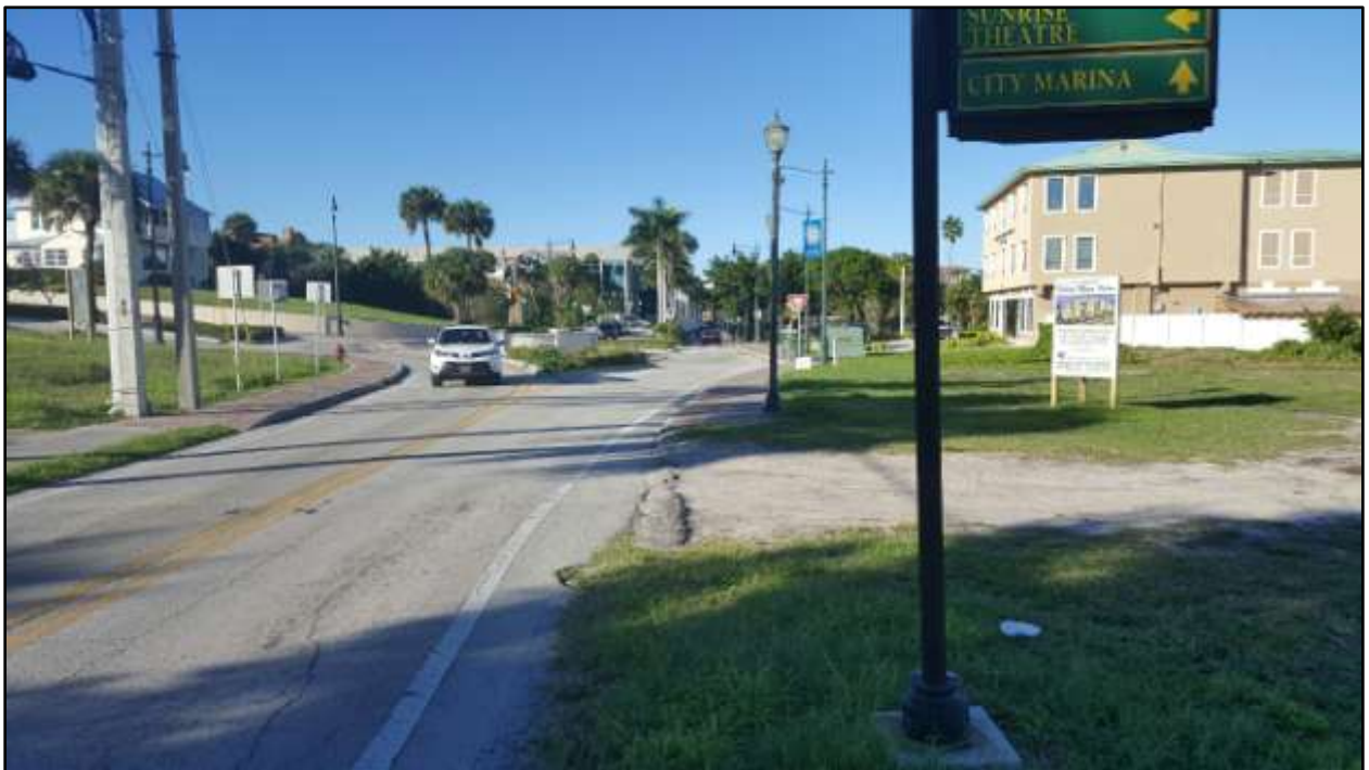
STREET SCENE ALONG SOUTH INDIAN RIVER DRIVE
