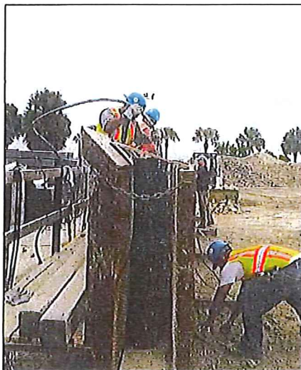
The 12-inch mats required a filling frame, fabricated by the contractor. The panels came pre-assembled with the exception on the side panel, through which a front-end loader placed the stone fill. Then, the side panel was attached and loaded into the stockpile.
