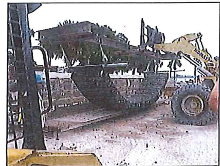
The 12-inch mats required a filling frame, fabricated by the contractor. The panels came pre-assembled with the exception on the side panel, through which a front-end loader placed the stone fill. Then, the side panel was attached and loaded into the stockpile.
