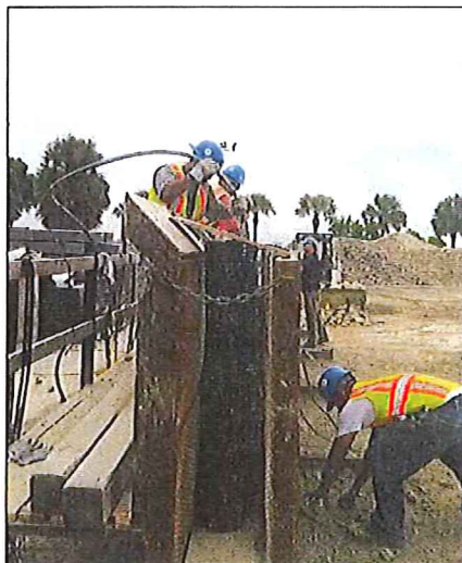
The marine mattresses were filled on-site. The smaller ones were placed on a flat surface and filled by hand to reduce the void space.
