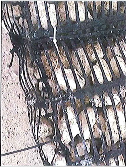
The mattresses used were two different thicknesses, 12-inch and five-inch, and were five feet and six-and-a-half feet wide. The stone fill ranged in diameter from five to 20 inches.
