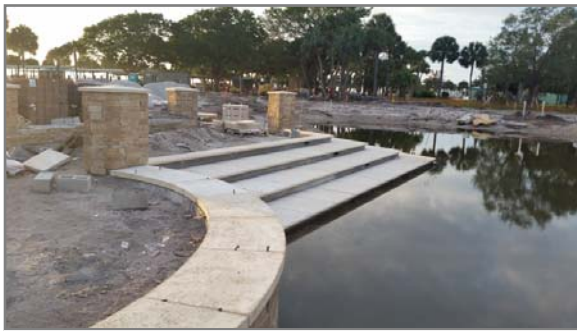
Lake Seating Terrace Area
