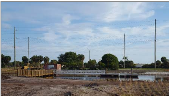
Completed Canoe Launching Facility / Docks
