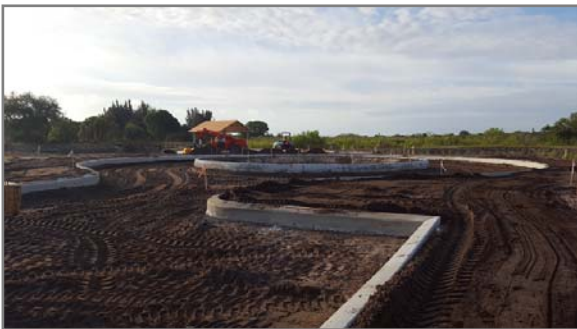
Picnic Shelter and Parking Area
