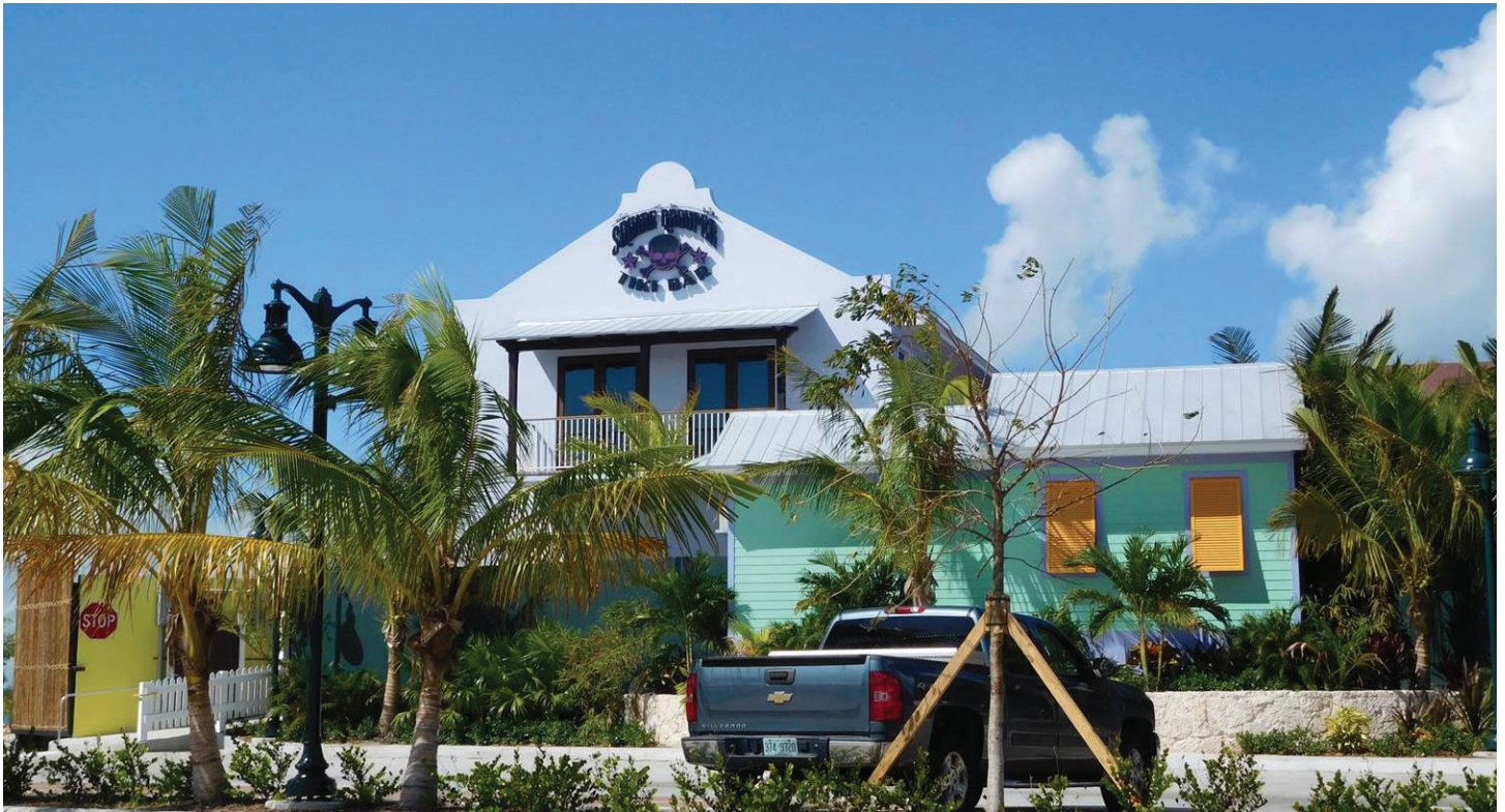
Square Grouper sign has been installed. Restaurant is nearing completion.
