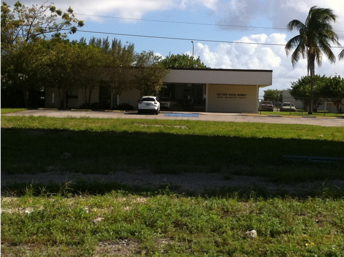
Wastewater Treatment Plant – North Elevation
