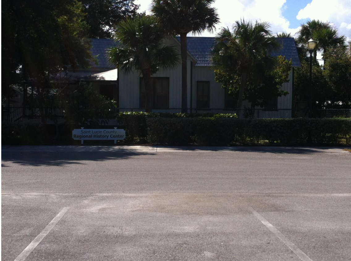
St. Lucie County Historical Center – South Elevation
