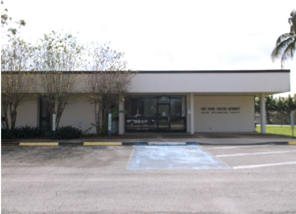
Wastewater Treatment Plant - North Elevation
