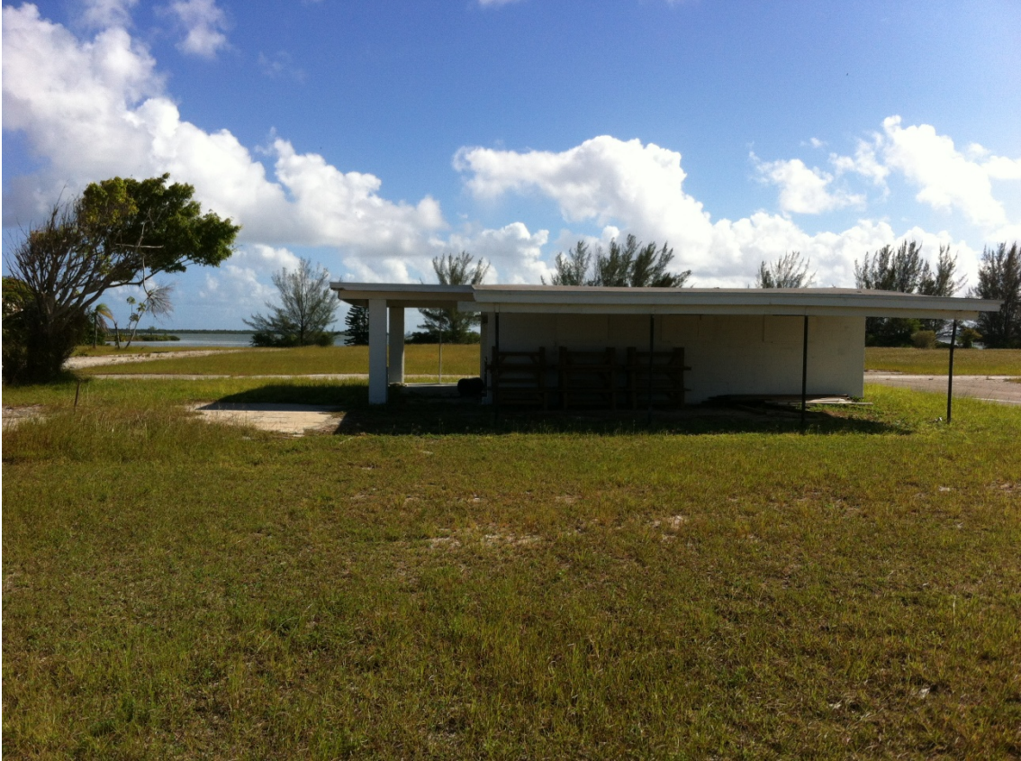
Existing Maintenance Building at 601 Seaway Drive – North Elevation
