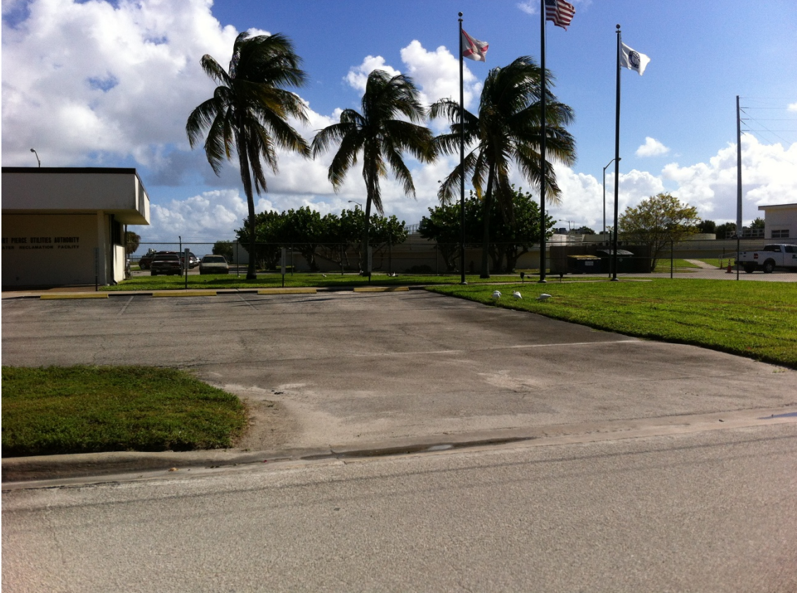
Wastewater Treatment Plant – North Elevation
