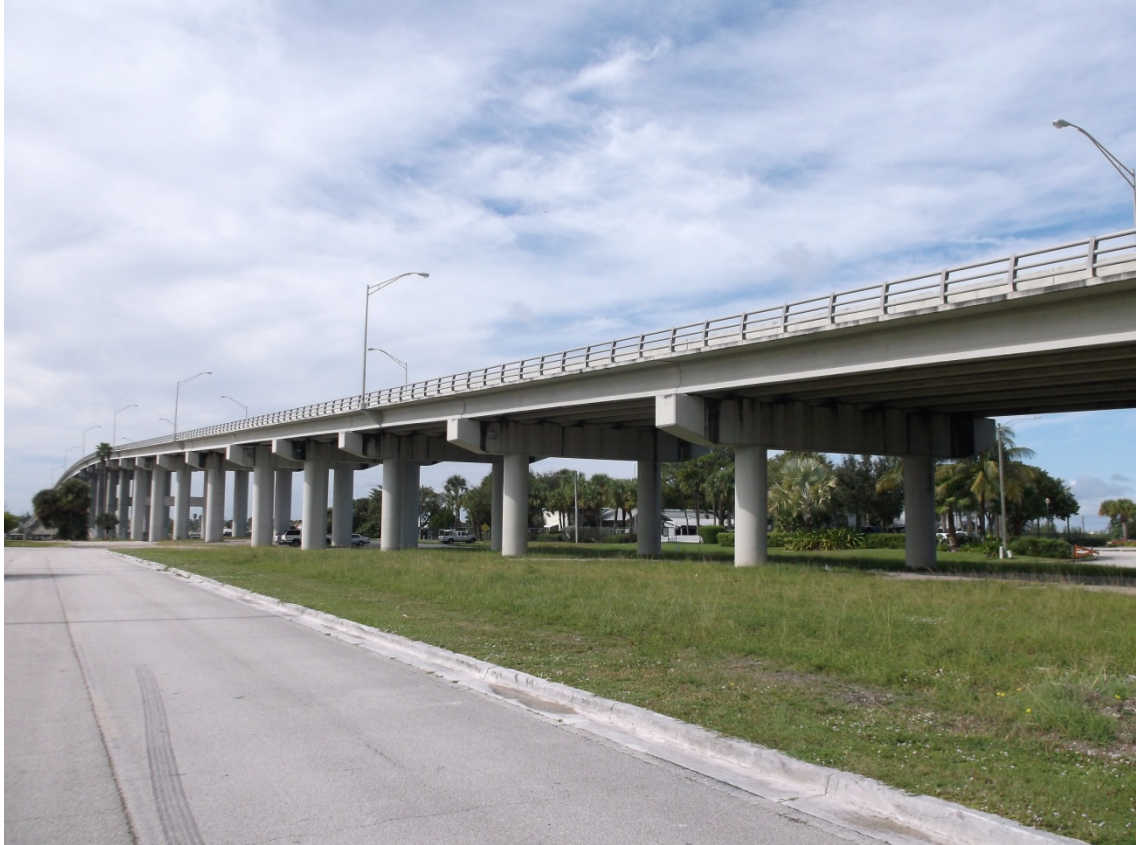
Seaway Drive Bridge
