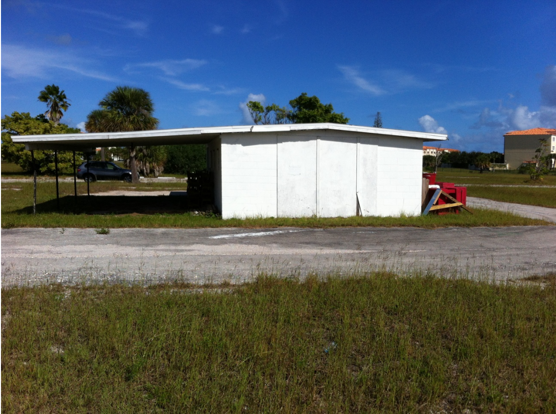
Existing Maintenance Building at 601 Seaway Drive – West Elevation
