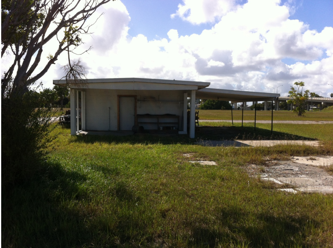
Existing Maintenance Building at 601 Seaway Drive – East Elevation
