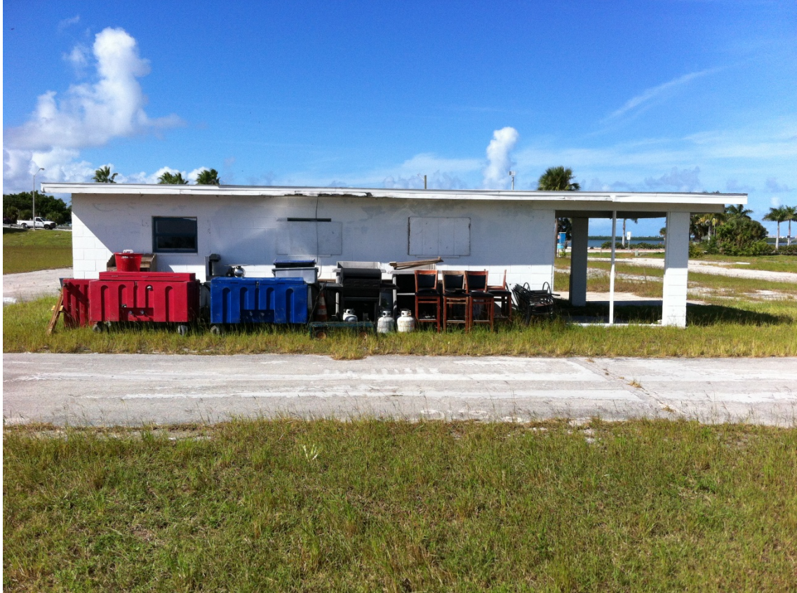
Existing Maintenance Building at 601 Seaway Drive – South Elevation
