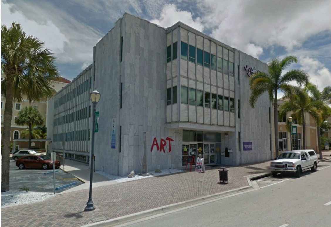
Existing Building - Orange Avenue View
