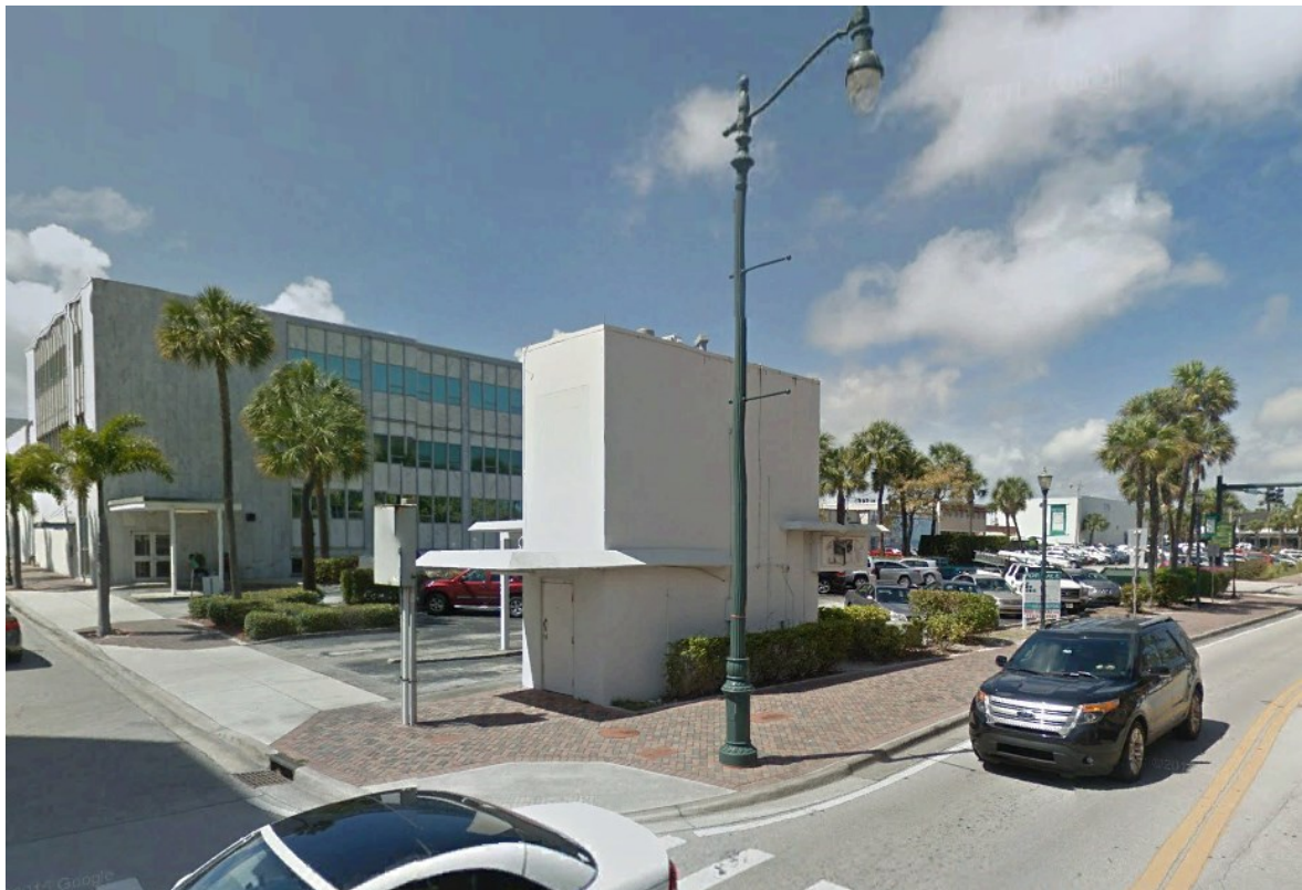
Existing Parking Accessory Structure - S Indian River Drive View
