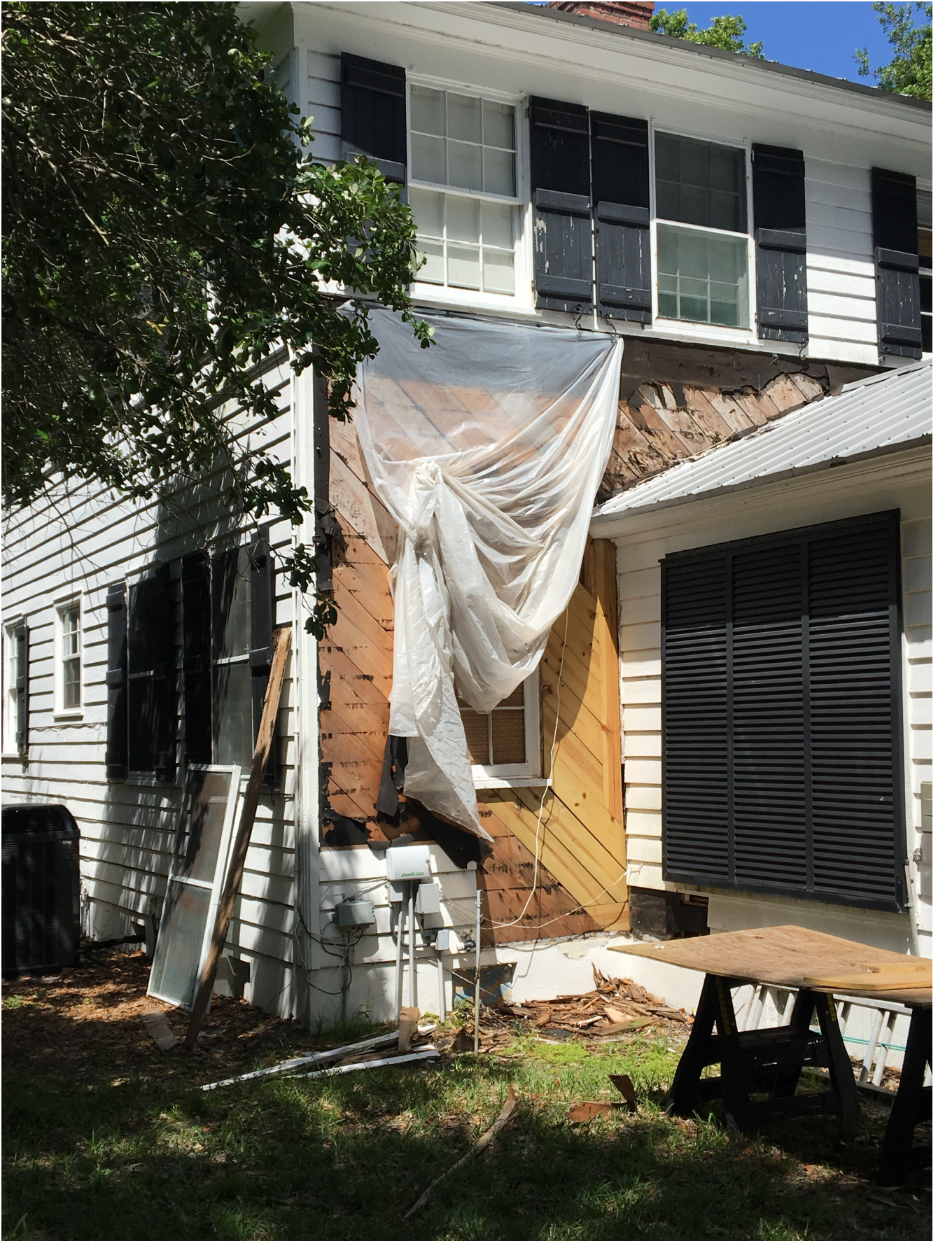
Rotten siding replacement
