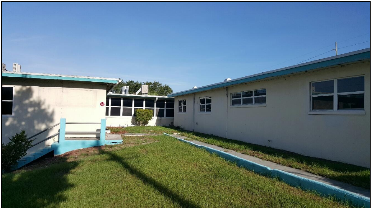
FRONT VIEW OF SUBJECT IMPROVEMENTS
