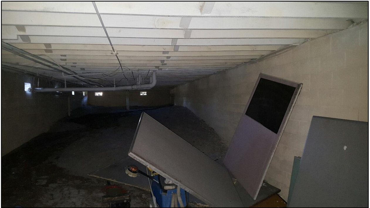
INTERIOR VIEW OF BASEMENT AREA
