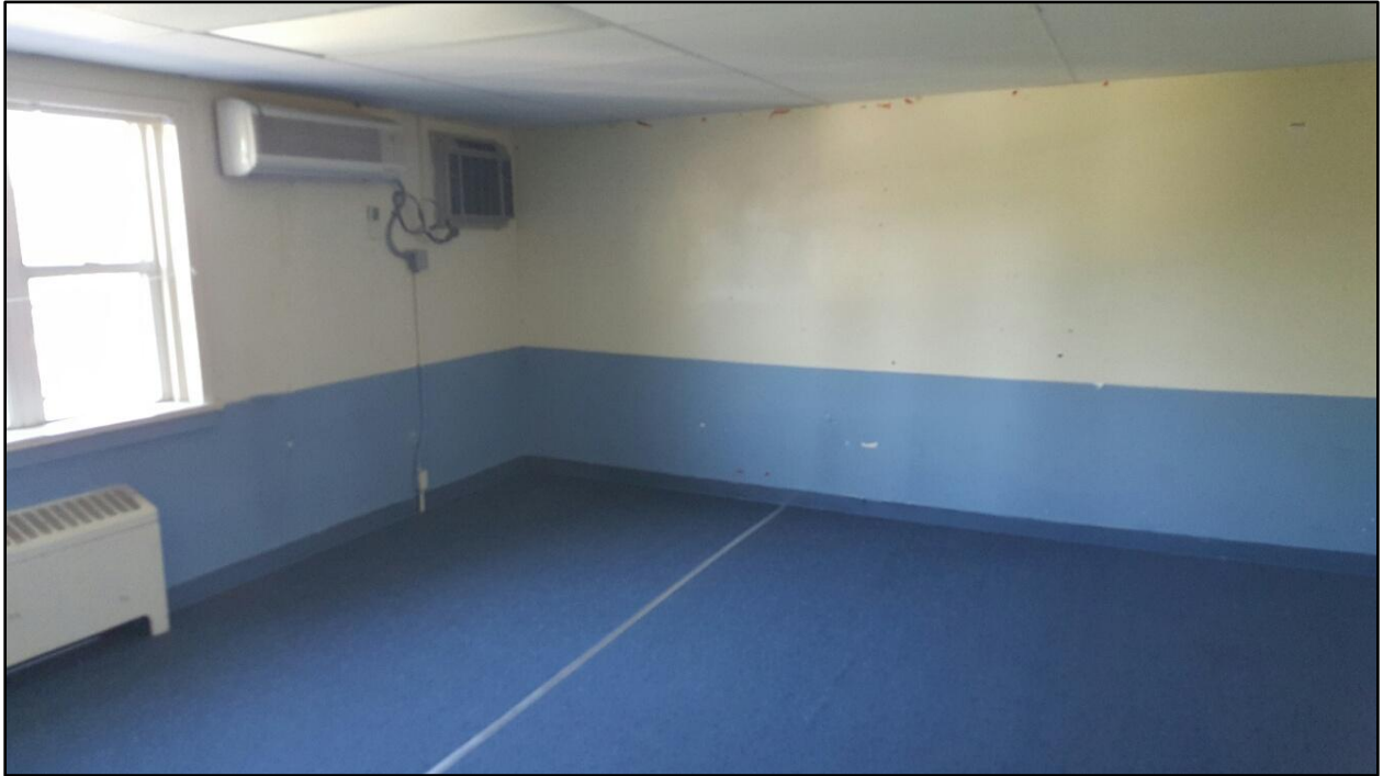
TYPICAL INTERIOR VIEW
