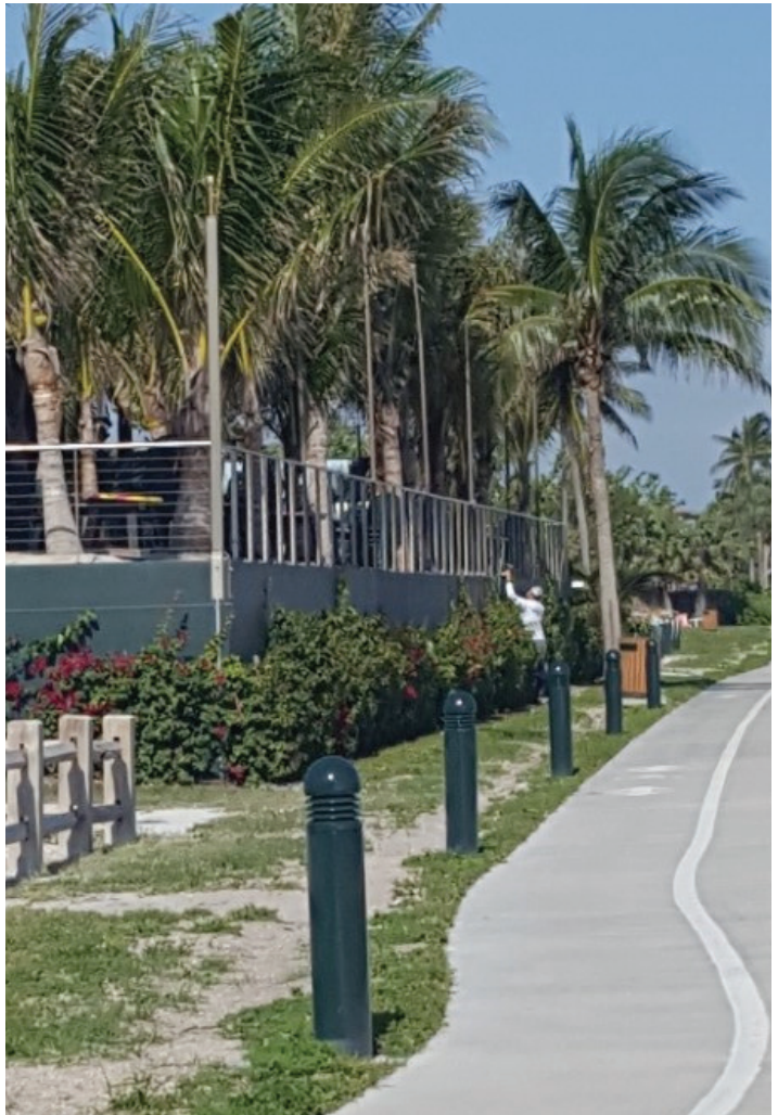
Another exciting project going on in the Public Works Department is the installation of bollard lights along Inlet Linear Park. Over 30 decorative lights are being installed and will be operational soon. These are the same turtle friendly, low level lights that are installed within Jetty Park.
