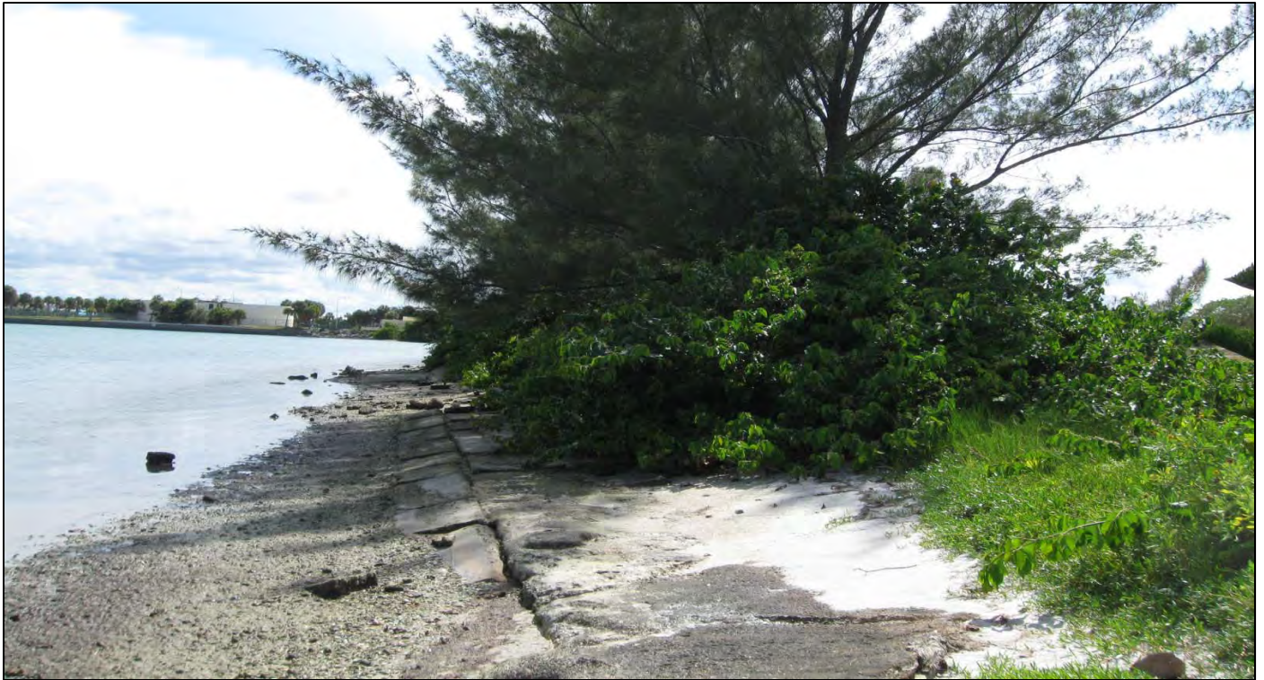
Photo looking west along shoreline showing concrete rubble, coin vine, Australian pine and some mangroves.
